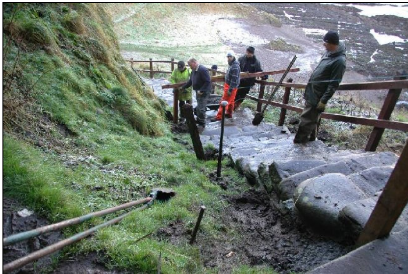
Illus 5: Installation of posts, looking NW
