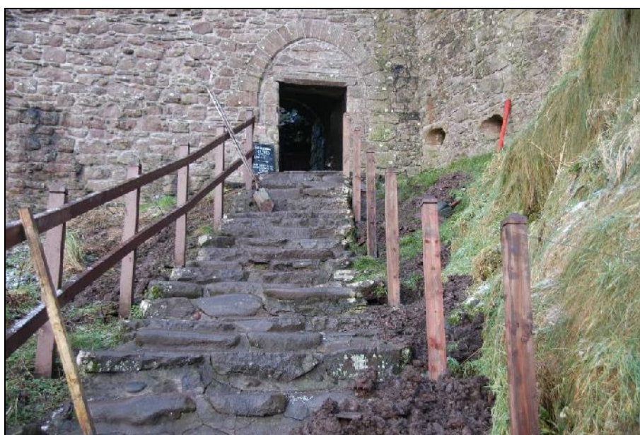
Illus 3: Fence 2, looking towards castle entrance
