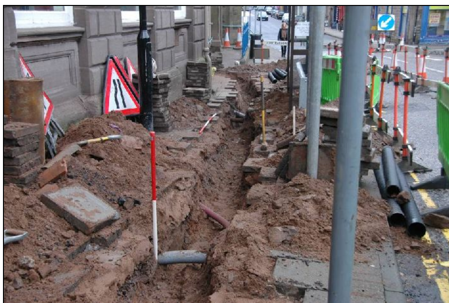
Illus 4: Cable trench, looking W, showing earlier services
