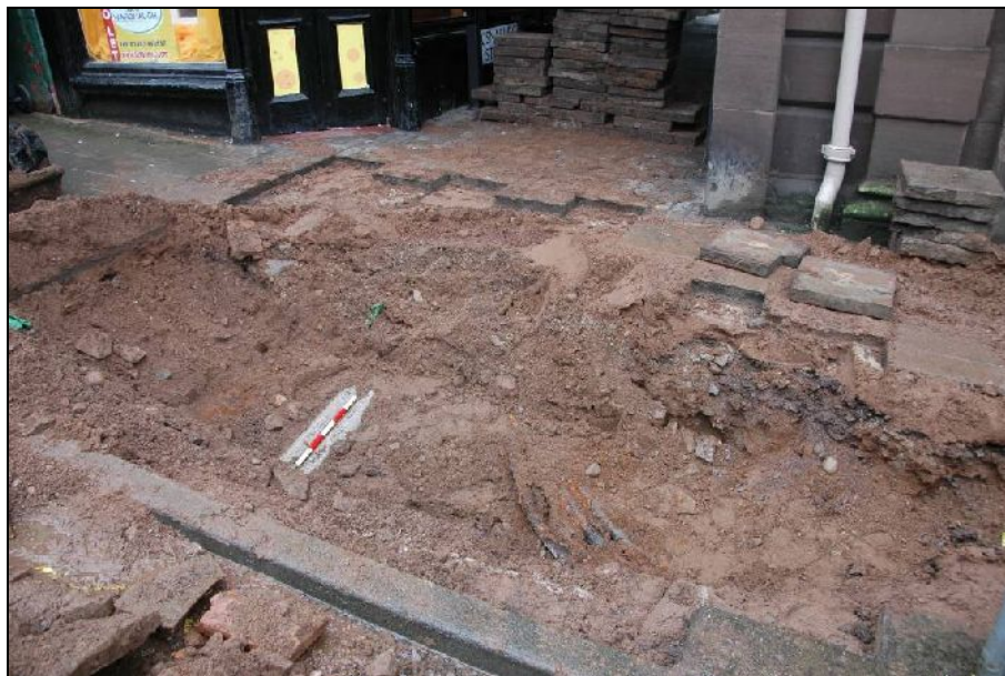
Illus 5: E end of trench at Osnaburg Street, looking S
