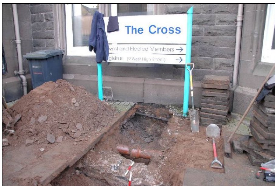
Illus 2: W end of trench showing existing services and stone wall, looking S
