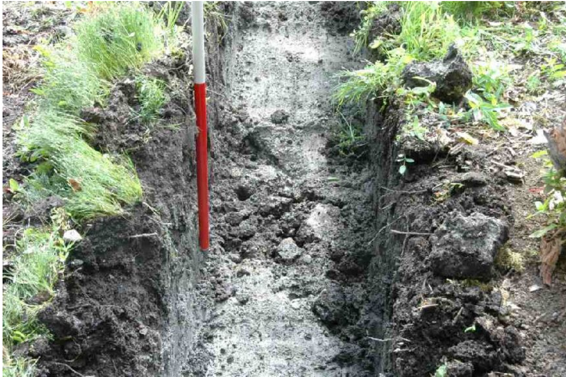
Illus 2 Grey/blue clay in base of trench just W of the boundary fence between the field and the garden.
