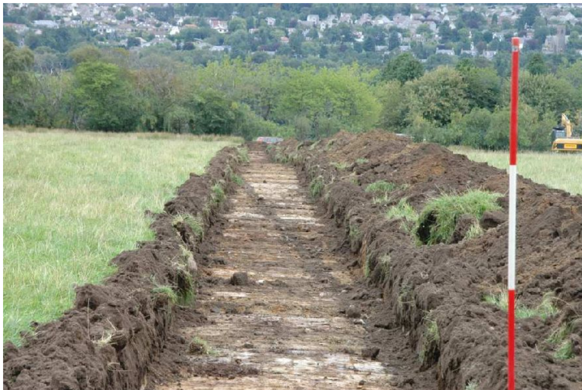
Illus 8 Trench 63 drain
