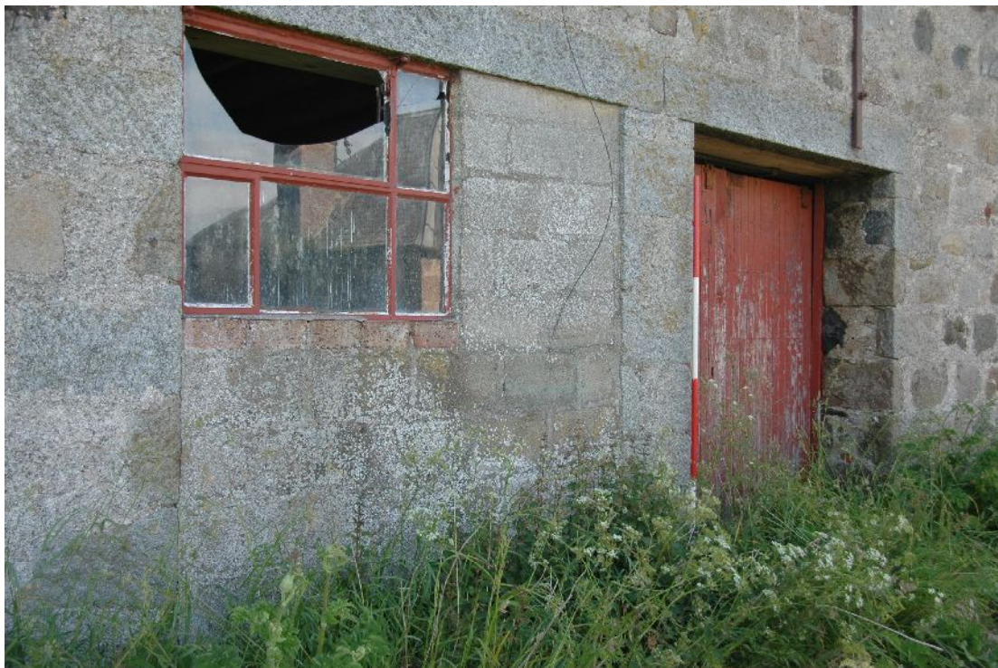
Illus 5 Blocked cart bays (D13, D14) in W wall of W range
