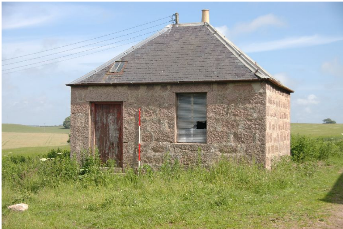
Illus 8 Bothy external view of S elevation
