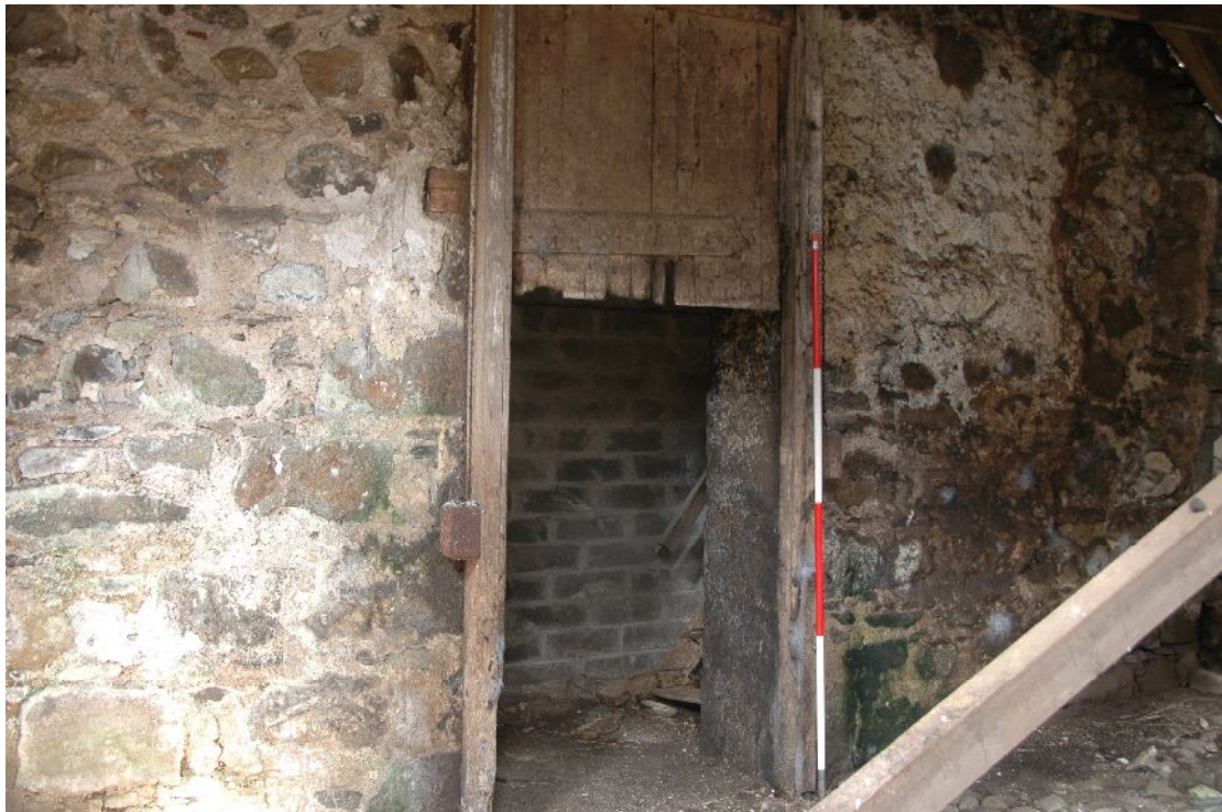
Illus 3 Door D16 with wooden shutter from loft above and metal counter-weight to LHS of door
