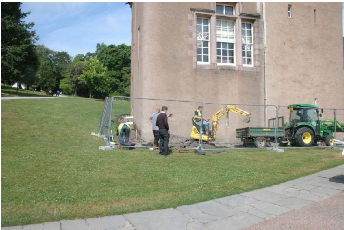
Illus 1 SW corner of tower showing position of the works.
