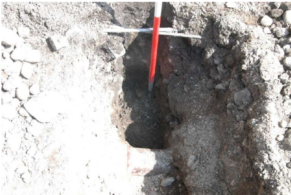
Illus 6 Trench 2 showing depth of wall foundation
