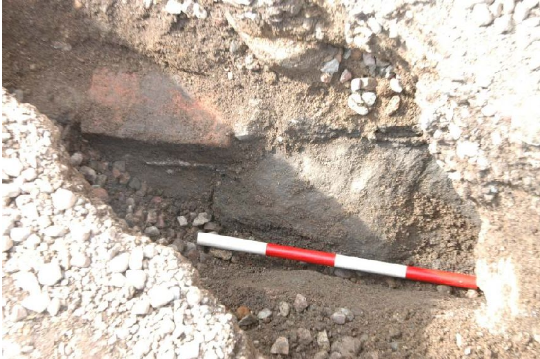
Illus 7 V shaped stone drain below new pipe trench
