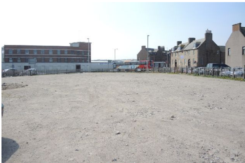
Illus 3 Site before machining looking to W sector at junction of St Peter Street and Erroll Street
