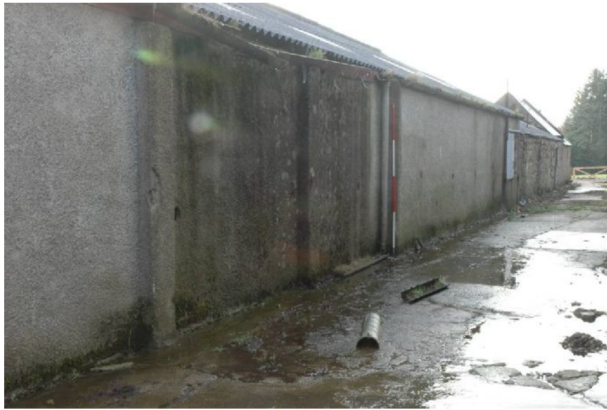
Illus 9 B2 Looking S along W wall. Ranging rod marks point where wall changes thickness (F4) The differences in roof height and material are visible.
