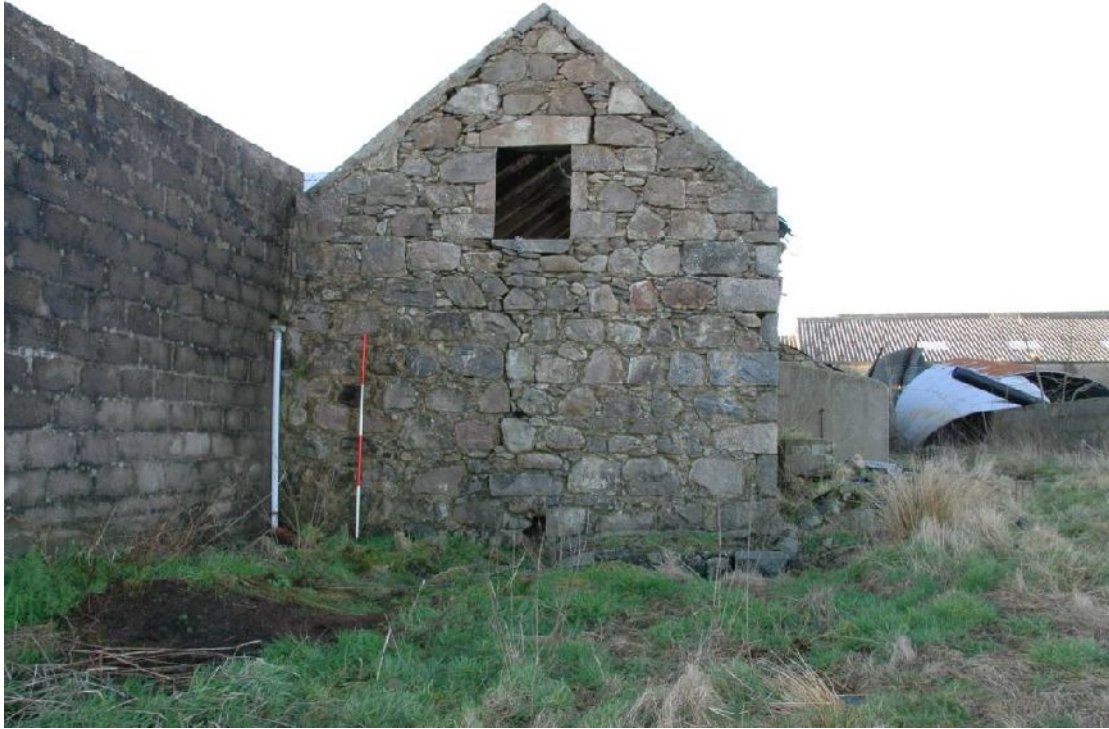
Illus 24 E gable of mill (4B) with wheel shaft hole (F2) in centre of base of wall.
