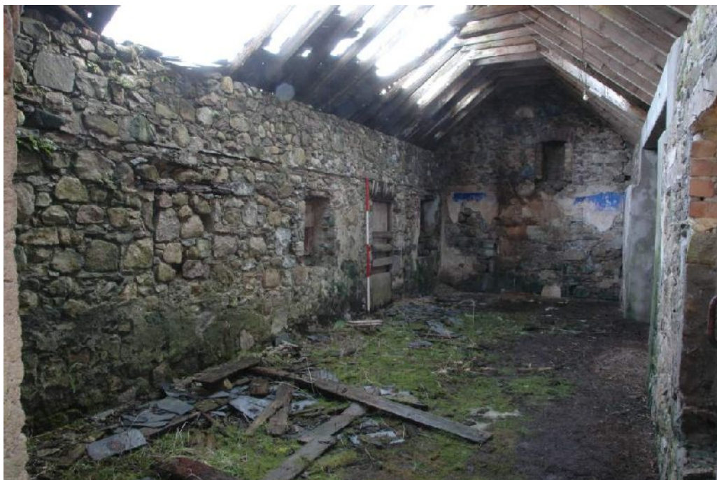
Illus 20 4A: Interior view looking E, showing back (N) wall).
