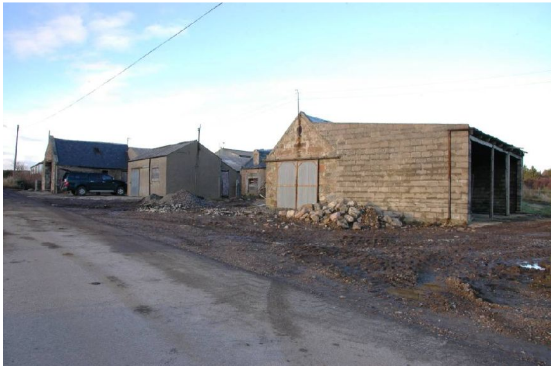
Illus 1 The site, general view looking N from the road
