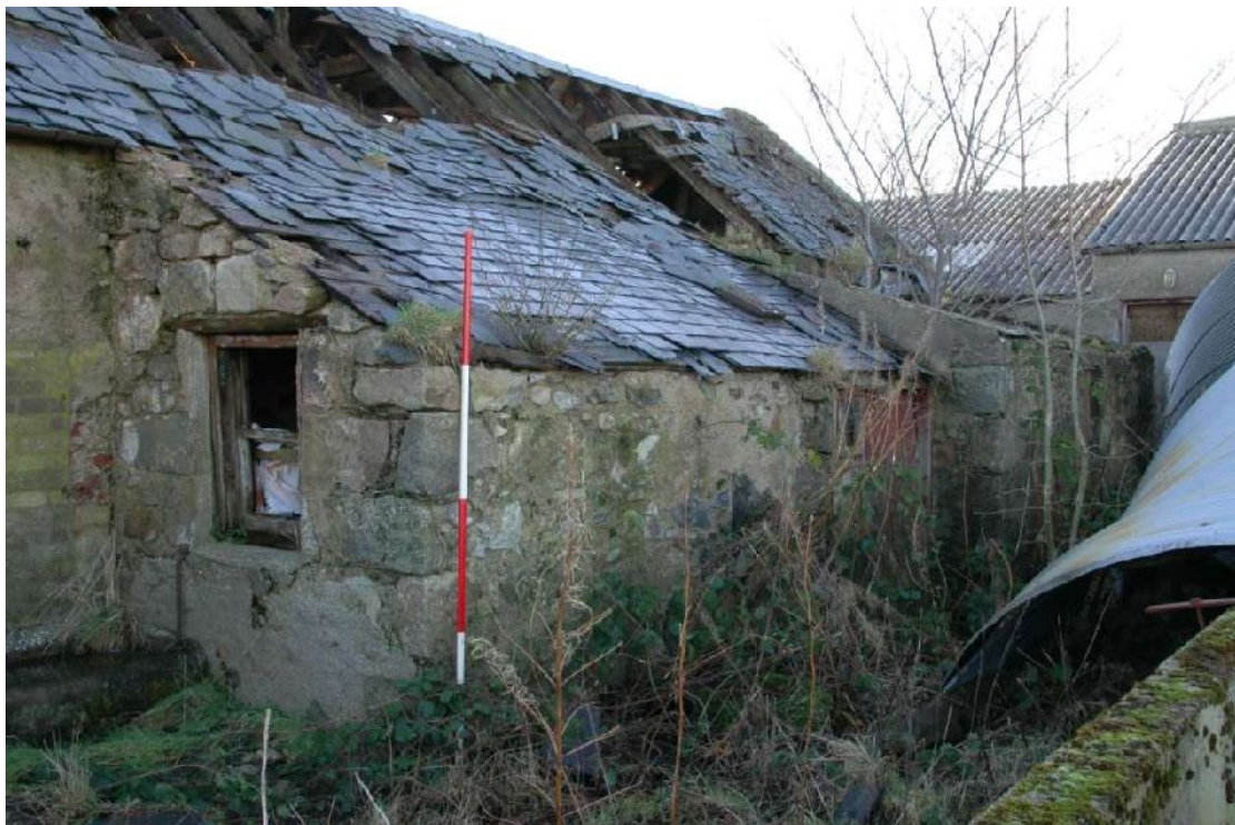
Illus 34 Buildings B9 and B 10 looking SW
