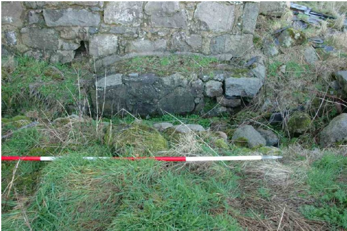
Illus 25 Detail of mill wheel pit and wheel shaft hole (F2)
