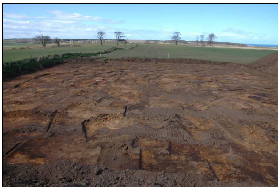
Illus 4: Hard standing and turbine base, looking NW.
