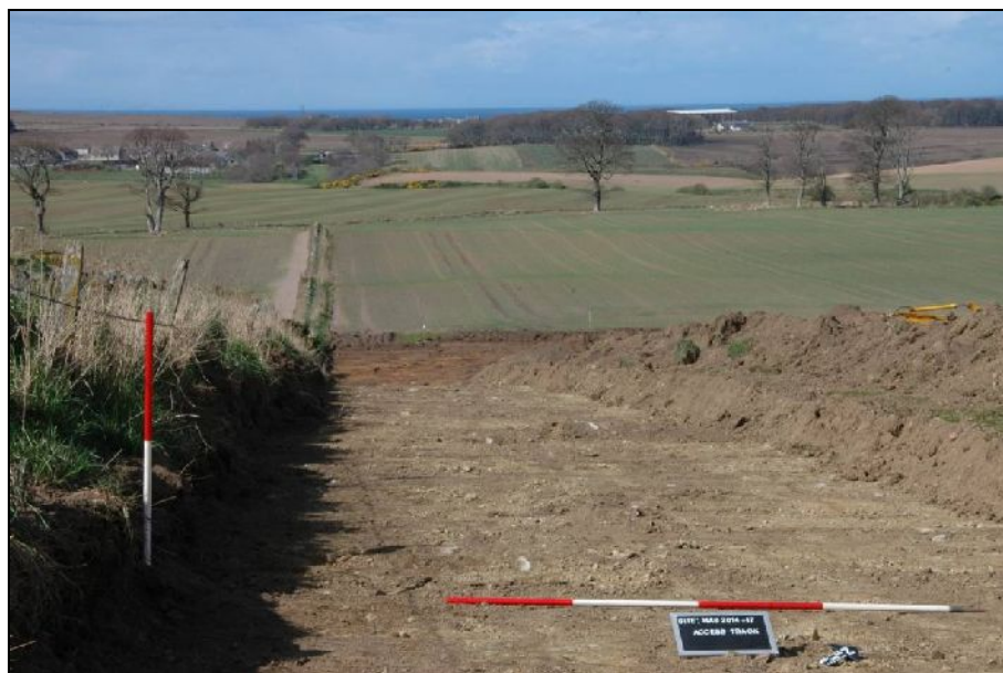
Illus 3: Access track, looking N to turbine location.
