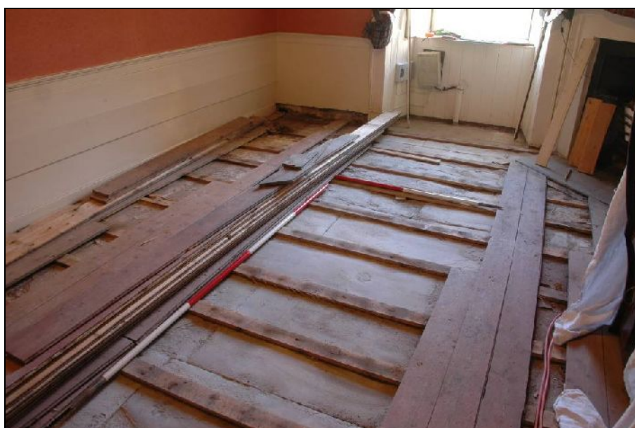
Illus 4: General view of room, looking W.
