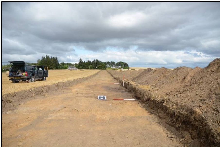
Illus 4: Cable trench with F1 in foreground, looking E
