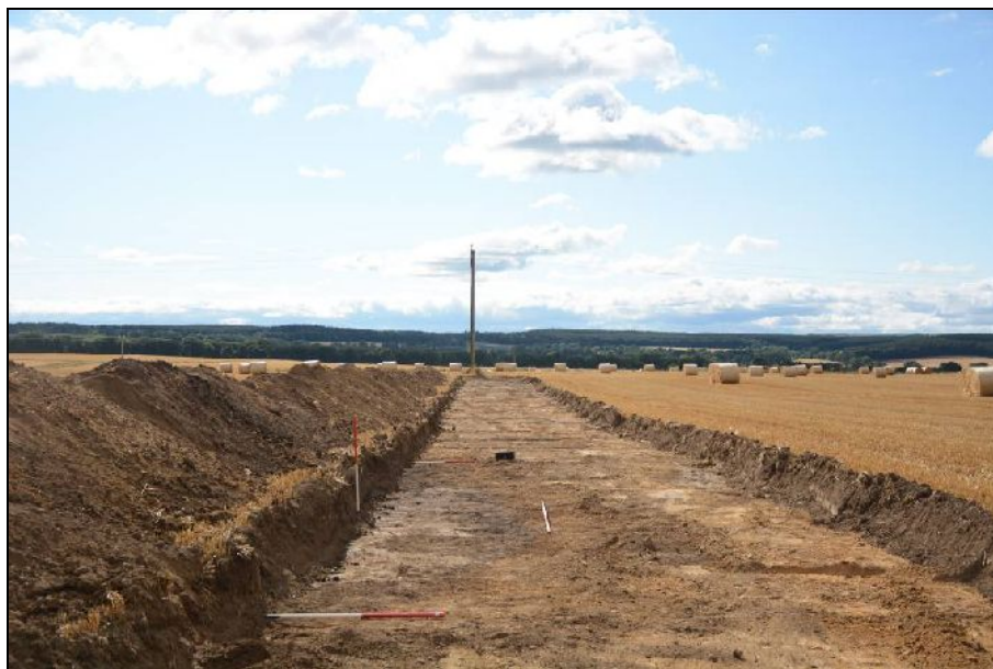
Illus 6: Cable trench and F1, looking W
