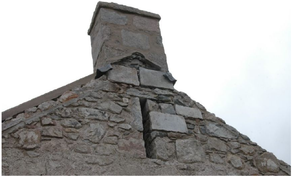
Illus 6 False chimney in N end gable E range, East Court.
