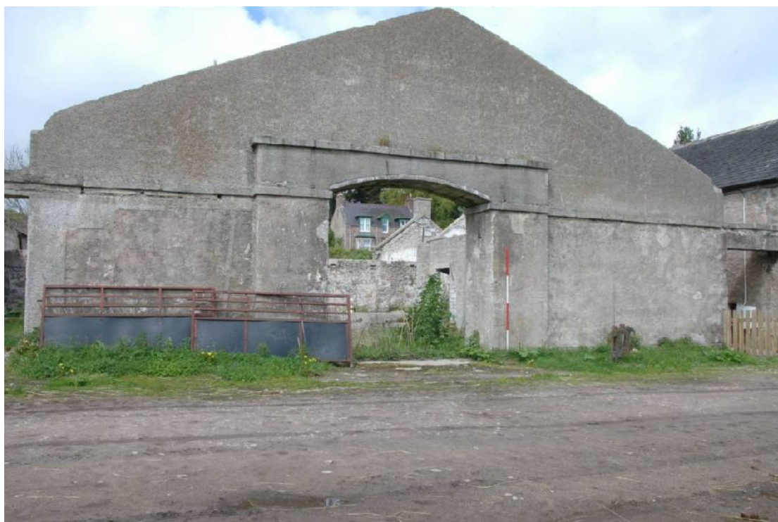
Illus 4 S wall of East Court showing the original 19 th -century stone wall with concrete above from the 20 th century infill.
