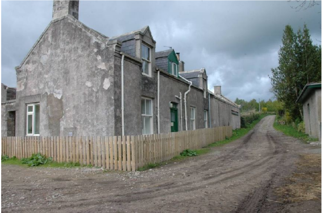
Illus 7 The house, looking NW
