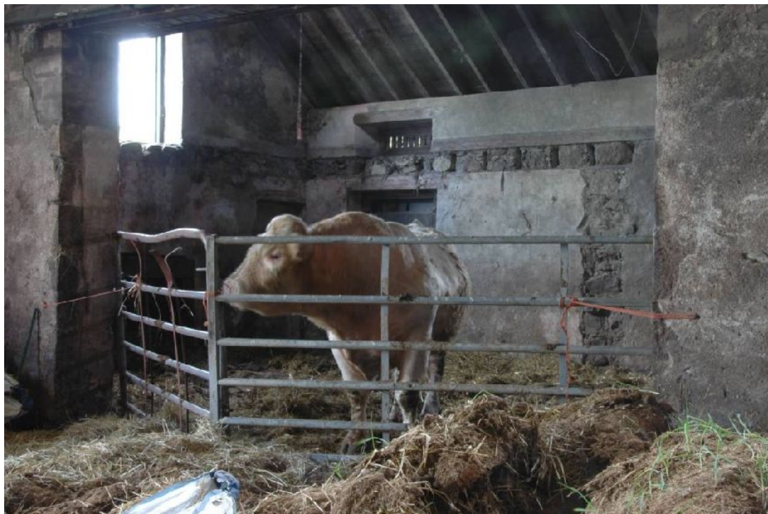
Illus 14 Looking through D30 to S end of interior of West Court W Range. On wall to LHS blocked door and central fireplace visible. On far wall raggle of loft floor and of internal partition wall of bothy.
