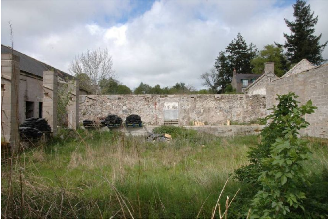
Illus 9 Looking N across East Court to S wall of N Range, some of blocked windows visible.
