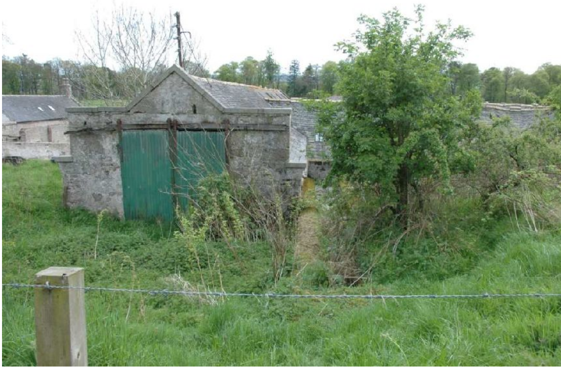
Illus 17 Mill from the N showing false front at gable. Lade visible on RHS.
