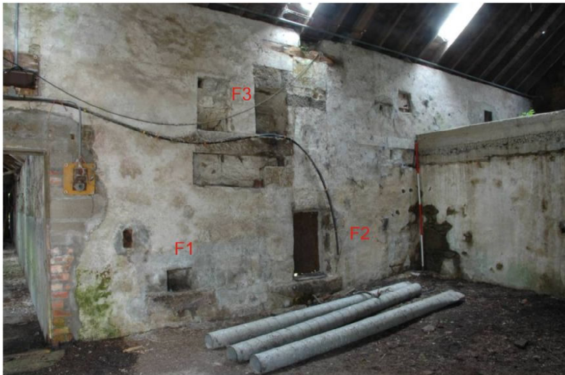
Illus 20 Inside of mill showing inner face of W wall with blockings F1-F3
