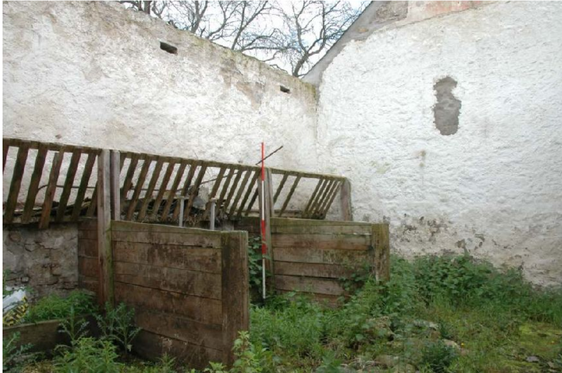
Illus 8 Tied cow stalls with vents above, in central part of East Court, E range.
