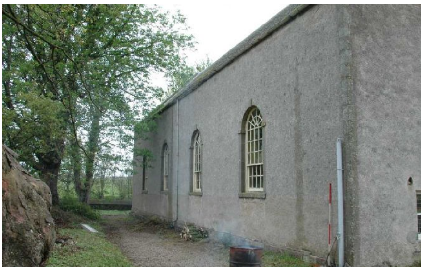
Illus 13 Looking W along S wall
