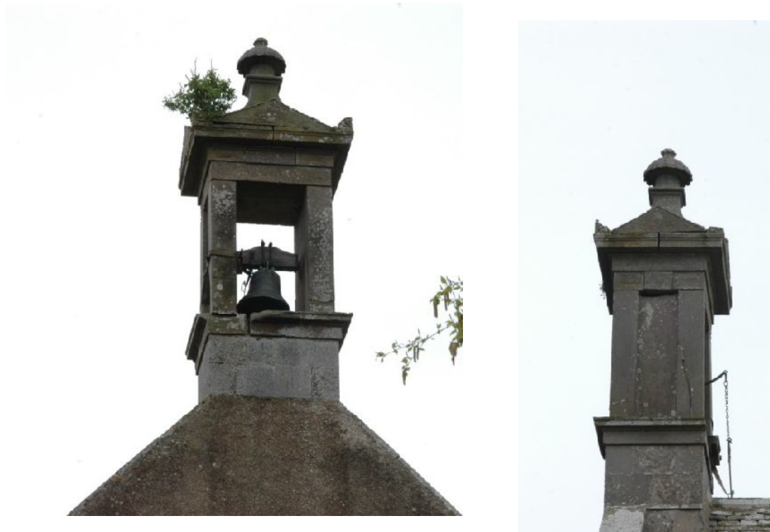
Illus 5 Bellcote from E (above) and from N (RHS).
