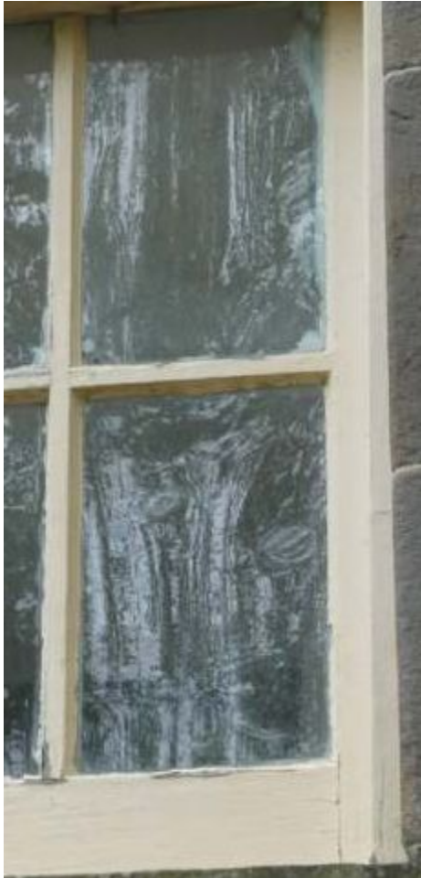
Illus 15 Detail of window W1 in S wall, bottom E panes to indicate glass ripples and bubble
