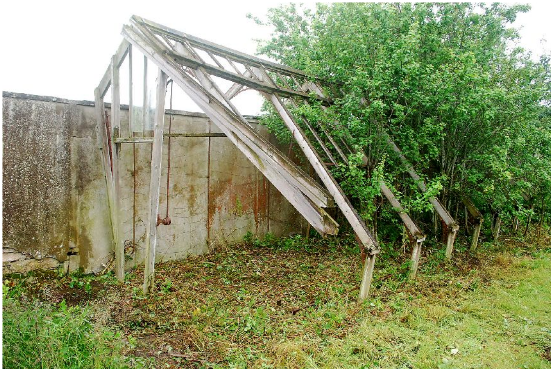
Illus 22 Overgrown state of glasshouse in 2009 showing N gable with winding gear (Photograph R Grant).
