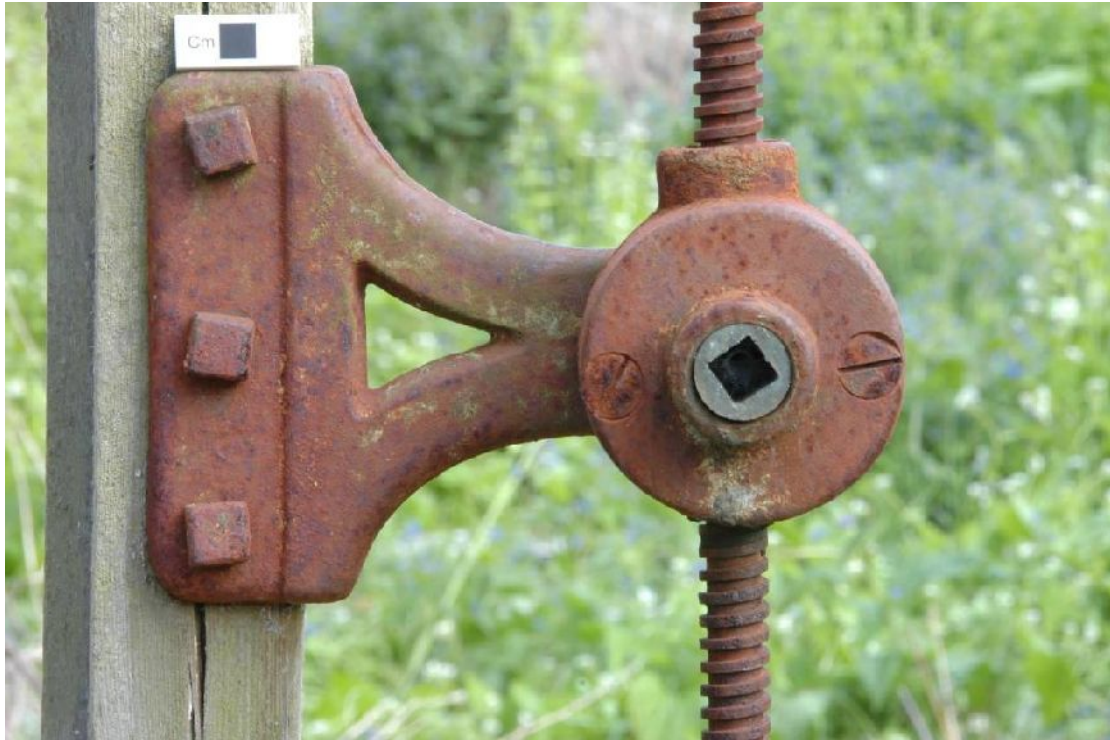
Illus 18 Ratchet at bracket (G) and threaded rod (F). Winding handle appears to be missing
