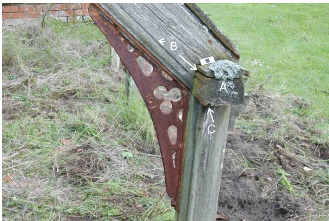
Illus 8 Detail of bracket between vertical wall post and rafter, also showing the horizontal timber (A) that ran along the top of the wall posts. Note the glazing grooves (B) for the sloping glass in the rafter and in the LHS face of the horizontal timber. Note also the glazing groove (C) in the base (LHS) of the horizontal.
