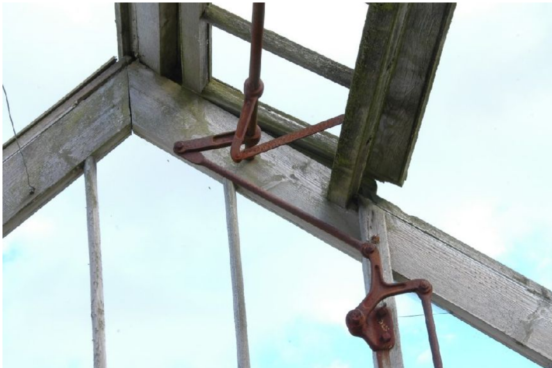
Illus 19 Detail of upper levers (C) and (E) connected by rod D. window lever (A) in front of (C). rod (B) at top of mechanism
