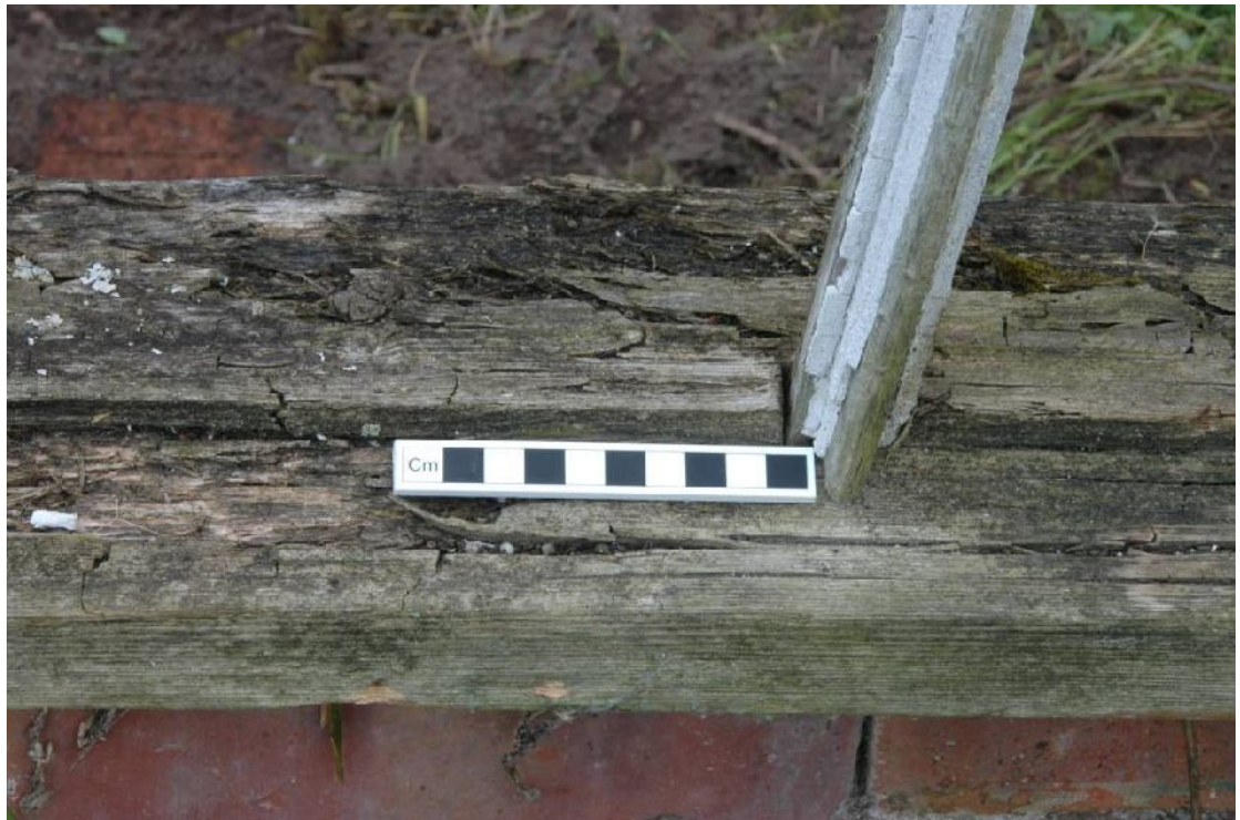
Illus 14 Detail of base of glazing bar mortised in wall plate in SE gable
