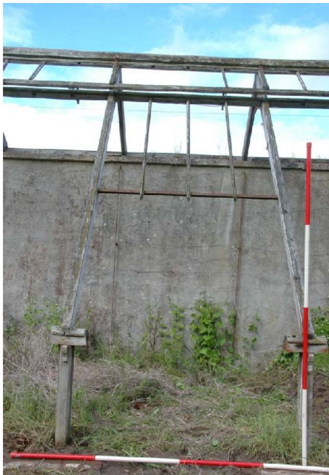
Illus 13 Bay 4 from S end showing glazing bars
