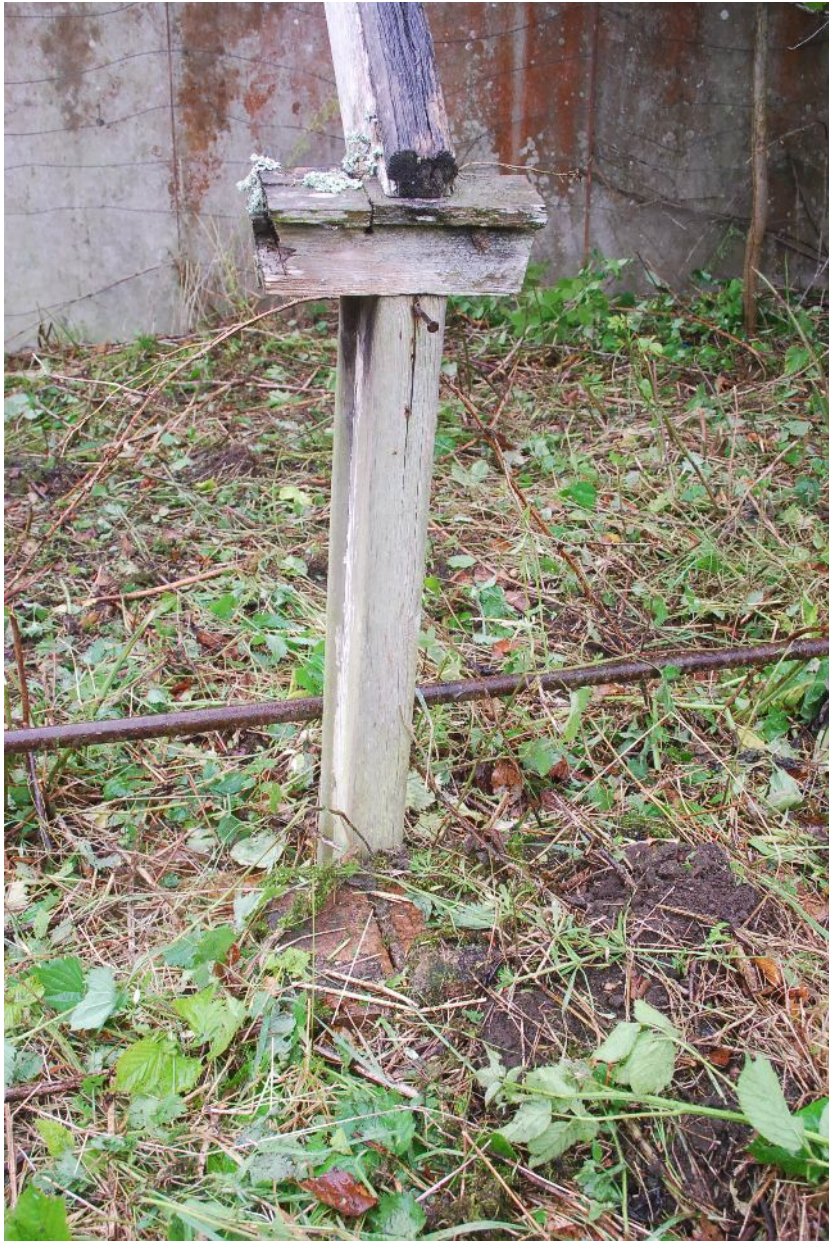
Illus 26 Horizontal metal rod for opening the lowest (vertical) windows. (Photograph R Grant).
