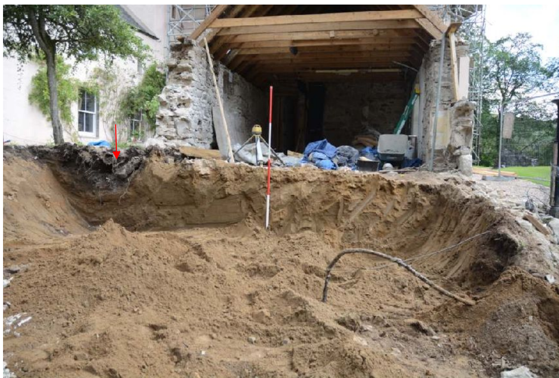
Illus 5 S wing, looking E, showing the excavation of the bank and the foundation for the replacement of the W gable. Red arrow shows cut for a modern ceramic drain.
