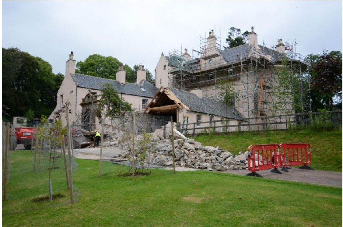
Illus 3 View of the castle from the SW showing the S wing with the W gable removed
