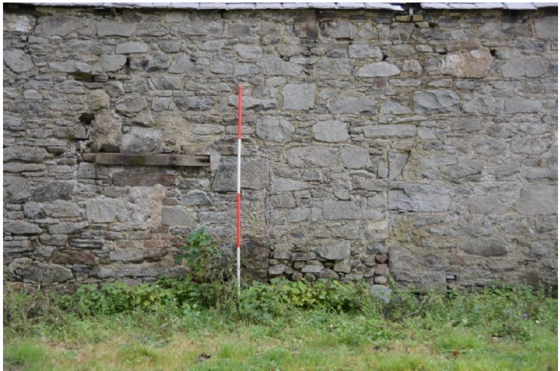
Illus 11 W wall W range. Blocking F1 and timber F2; possibly associated with the horse mill
