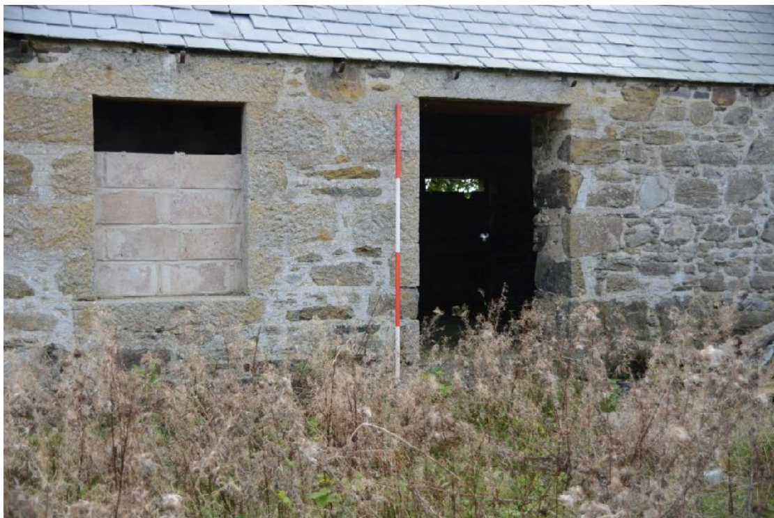
Illus 16 D9 and W4 in the E range with dressed granite lintel and rybats.
