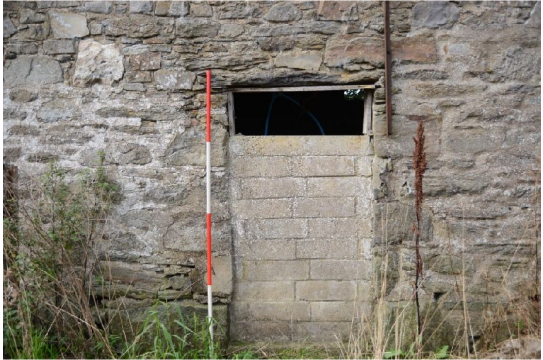
Illus 15 D17 in the W range with stone lintel and rough rybats
