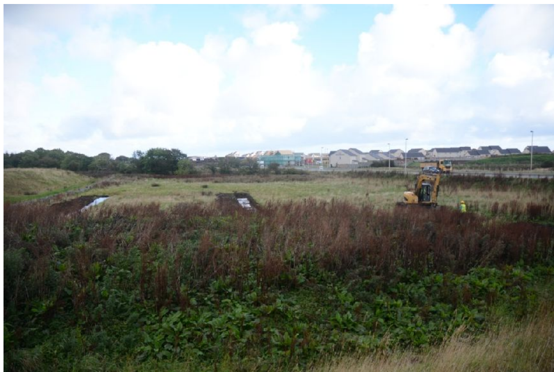
Illus 8 Trenches 1 and 2 looking N from topsoil bund
