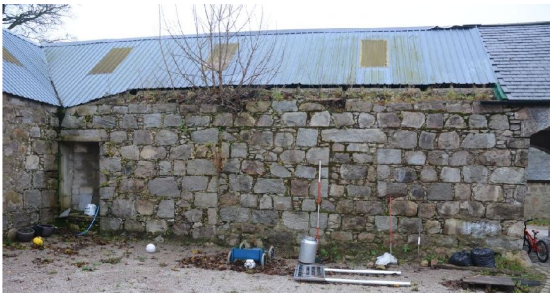
Illus 15 N wall of South Range. Note blocking F6 to the RHS of ranging rod and vertical break in stonework c.2m to LHS of ranging rod.
