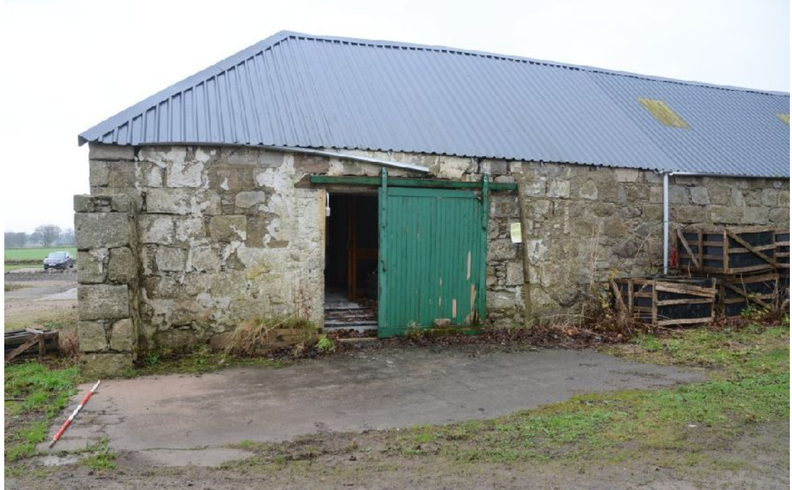
Illus 12 Eastern East Range. Horizontal Ranging rod lies across former doorway. Note concrete floor and raggle of render extending to RHS of green door.
