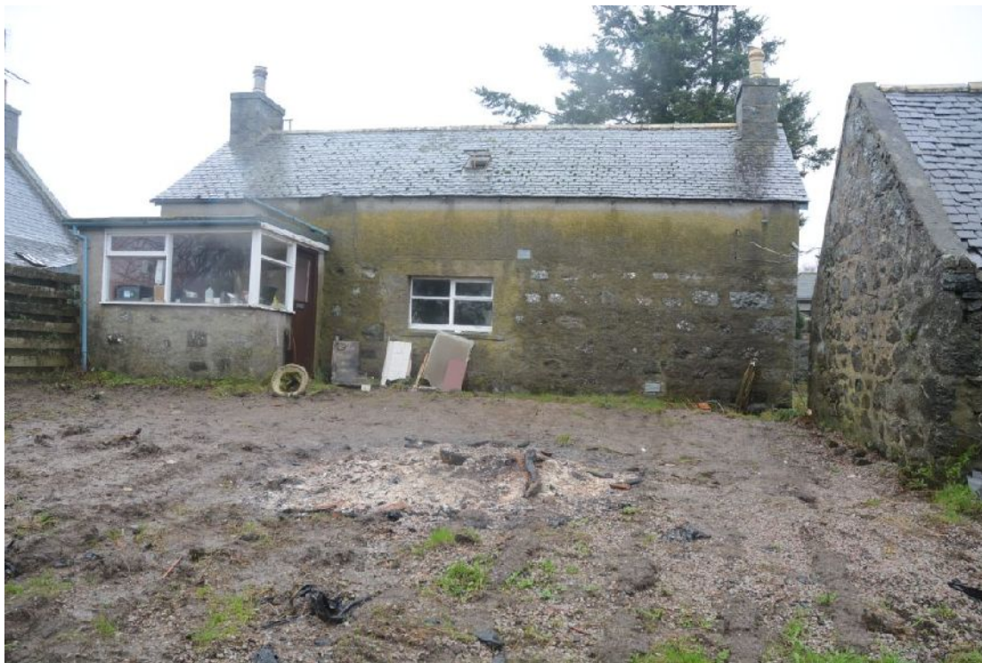
Illus 16 North wall of house showing raised wall, modern window and modern outshot.
