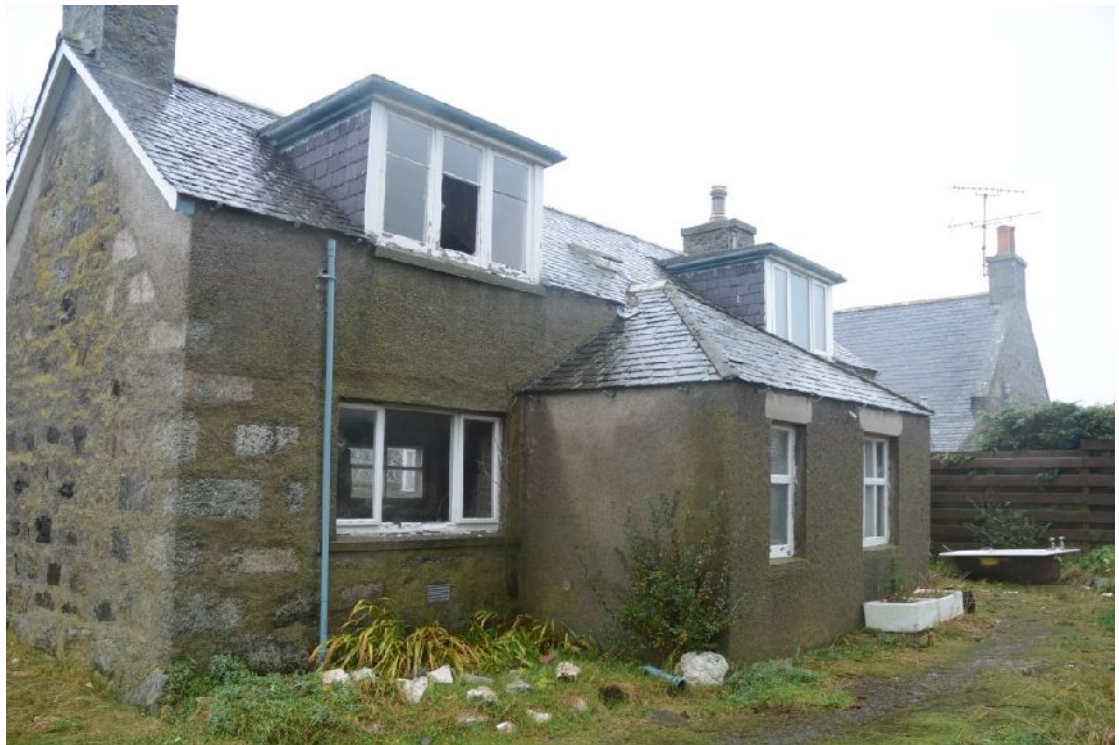
Illus 15 South and West walls of house, showing raised walls and gable, modern windows, dormers and outshot.
