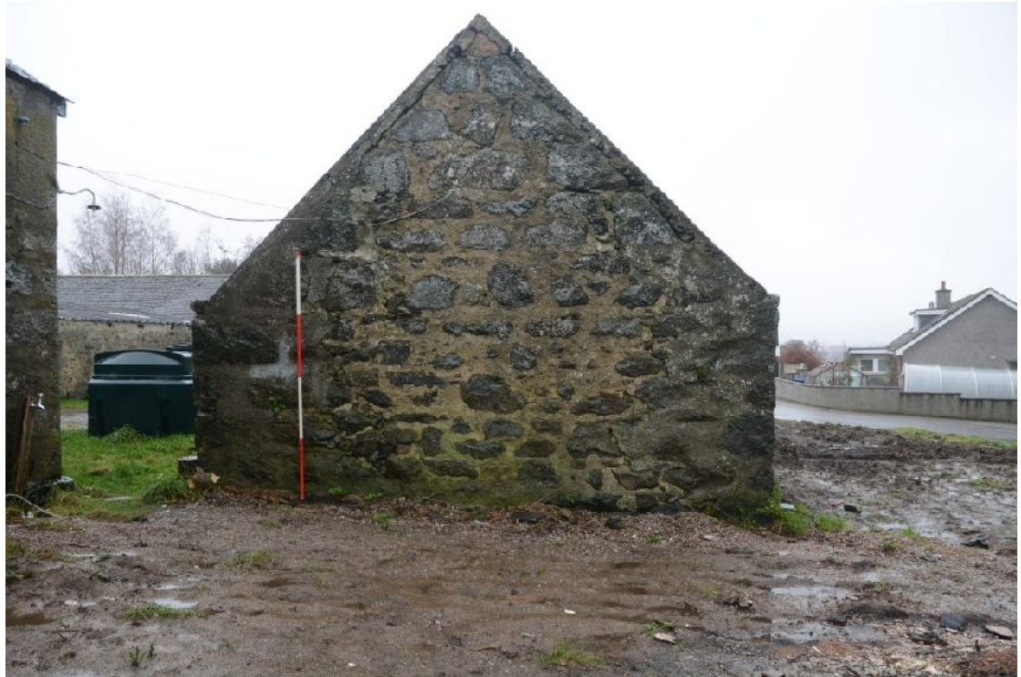
Illus 7 E gable. Note large well placed stones at apex and slight raising of wall height with secondary concrete and stone skews
