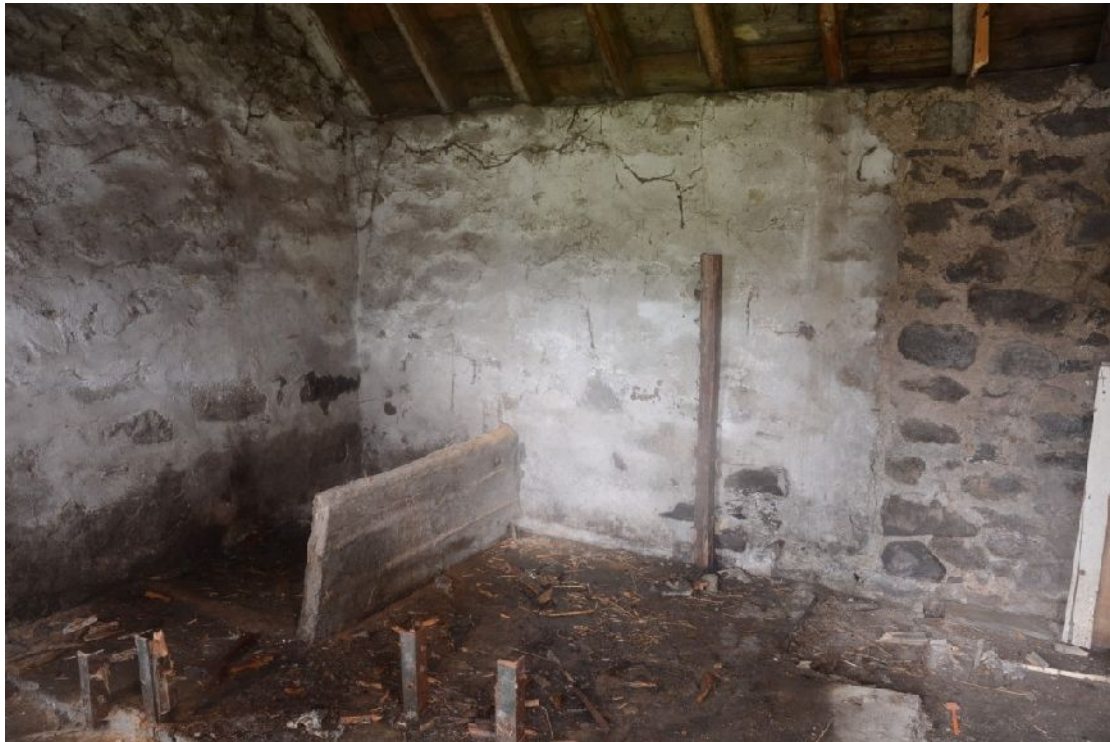
Illus 14 NW interior of E part of building. Note small pen in corner and render suggesting former division into two rooms/ areas.
