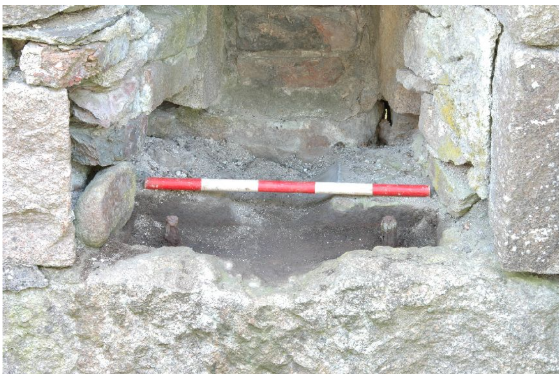
Illus 17 Caie's Mill, Kinellar, Aberdeen
