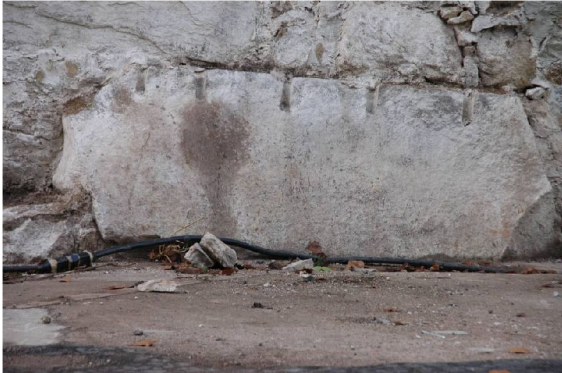
Illus 9 Base stone in garden wall showing quarry drill marks.
