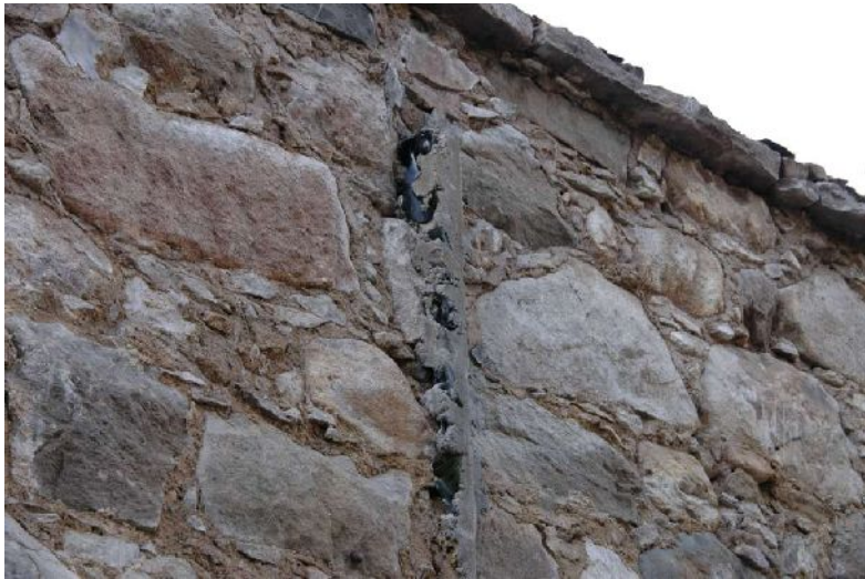
Illus 3 Glass bottle fragments in cement raggle (for position see illus 2: 8)
