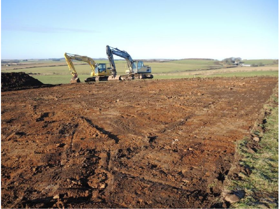
Illus 4 Crane pad after soil strip, looking NNW
