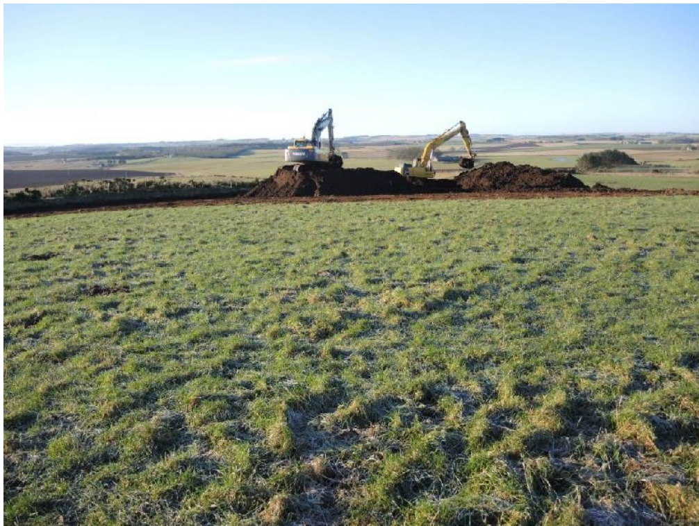
Illus 2 View of crane pad looking W showing open views
