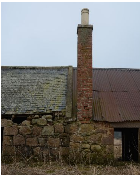
Illus 18 Brick chimney
