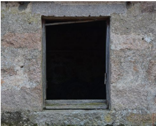
Illus 20 (LHS). Building 3. W5 showing grey granite lintel with quarry marks
