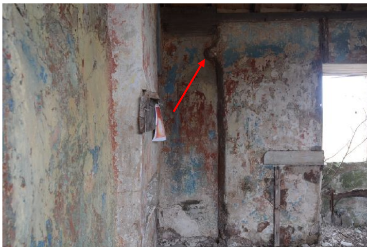
Illus 15 Inside of thick section of E wall of Building 2. Note projecting stone marked by arrow
