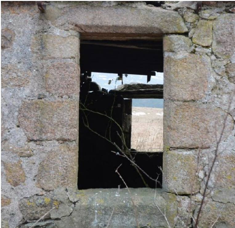
Illus 23 Building 2, W3 showing well dressed chamfered stones at margins.
