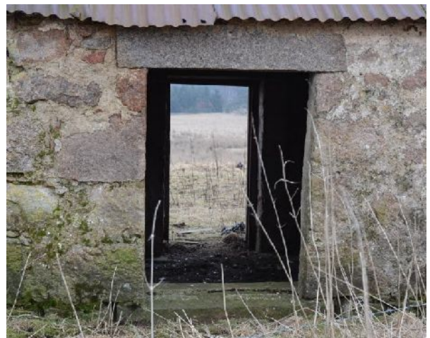
Illus 20 (LHS). Building 3. W5 showing grey granite lintel with quarry marks
