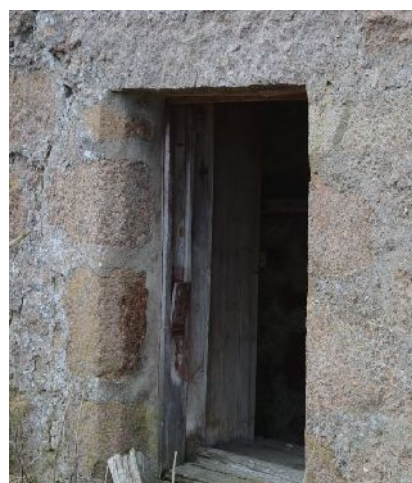
Illus 24 (LHS). Building 3. W4 showing re-use of chamfered stones at sides and lintel but replacement granite sill.
