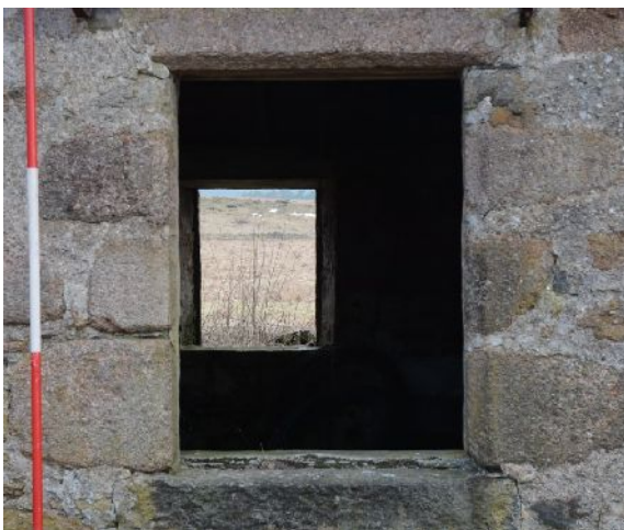
Illus 24 (LHS). Building 3. W4 showing re-use of chamfered stones at sides and lintel but replacement granite sill.
