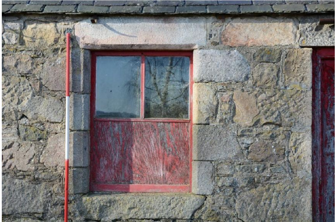
Illus 9 East Building. Window W1 with chamfered lintel and rybats
