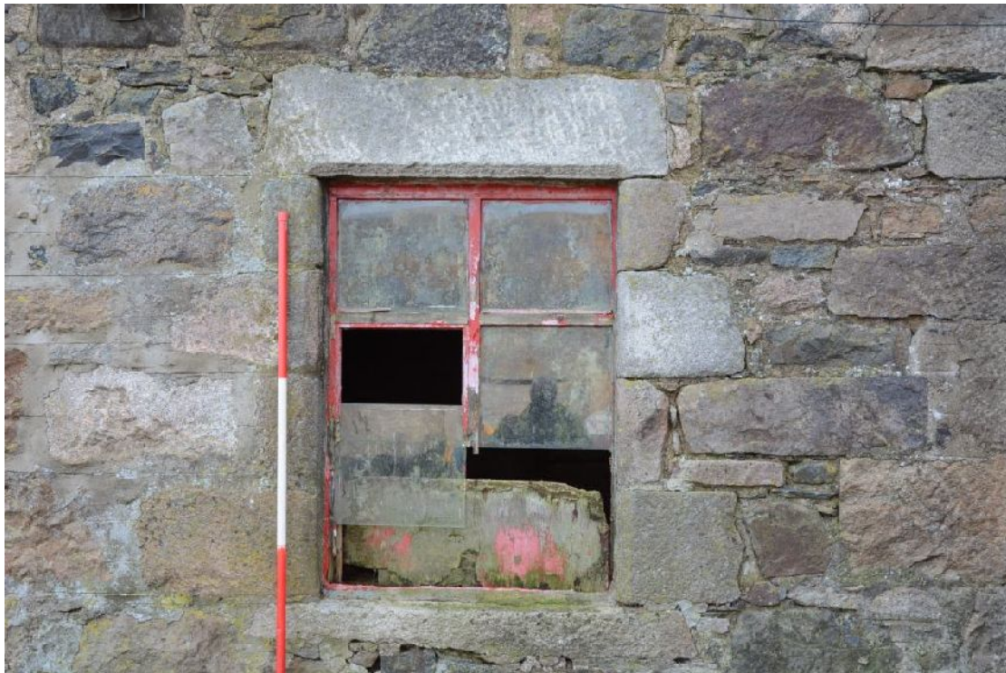
Illus 14 N wall of South Range. Detail of window W5 with chamfered rybats and lintel E wall
