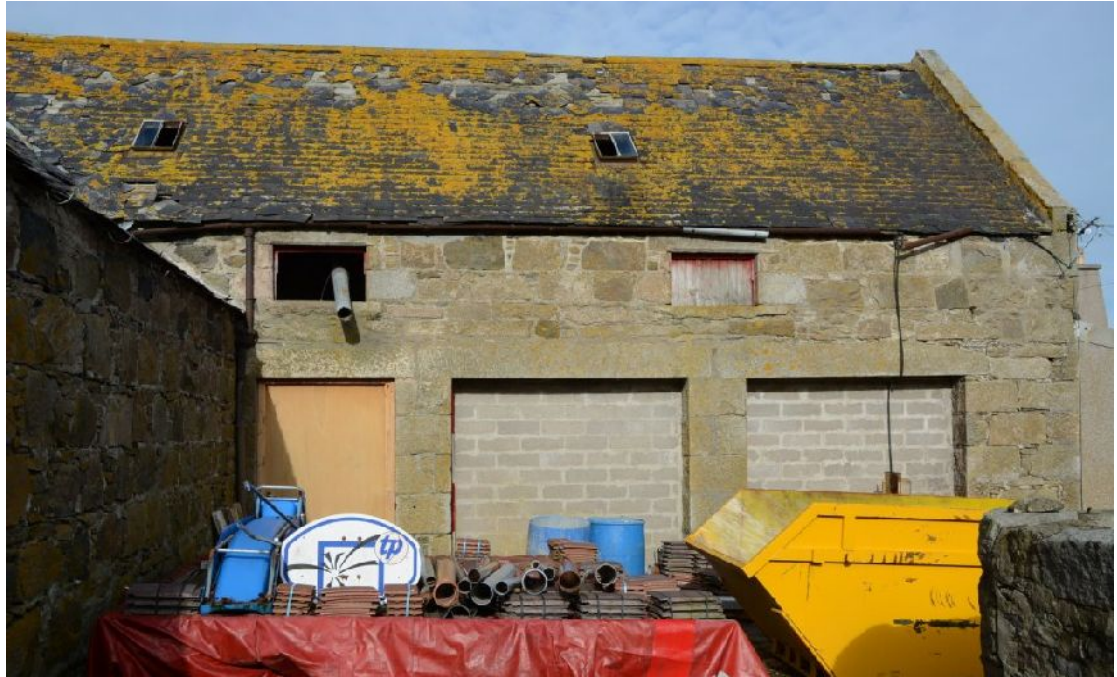
Illus 28 North Range., E end of S wall with cart bays D17, D18 blocked by concrete blocks.
