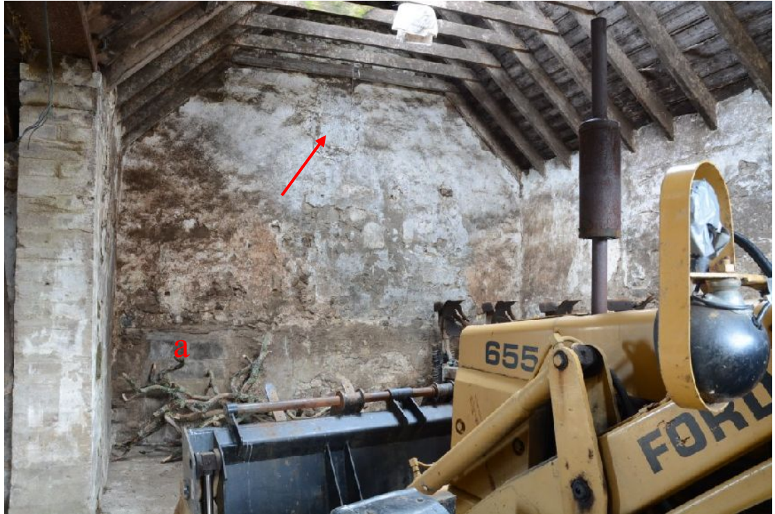
Illus 22 South Range. Interior of E wall. Arrow indicates blocking. 'a' indicates position of former feed bin
