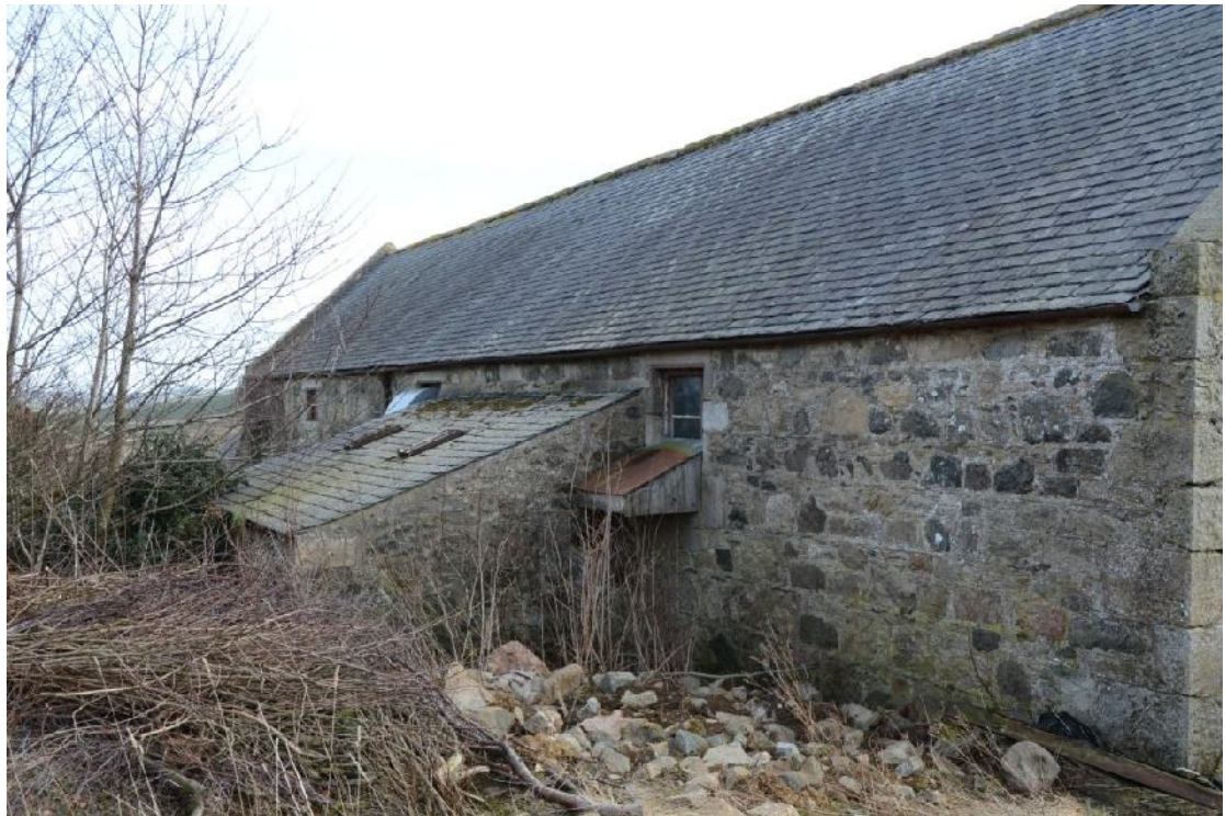
Illus 29 North Range. N wall with windows W8-W10 and engine house. The cover below W8 (RHS) protected the shaft from engine house
