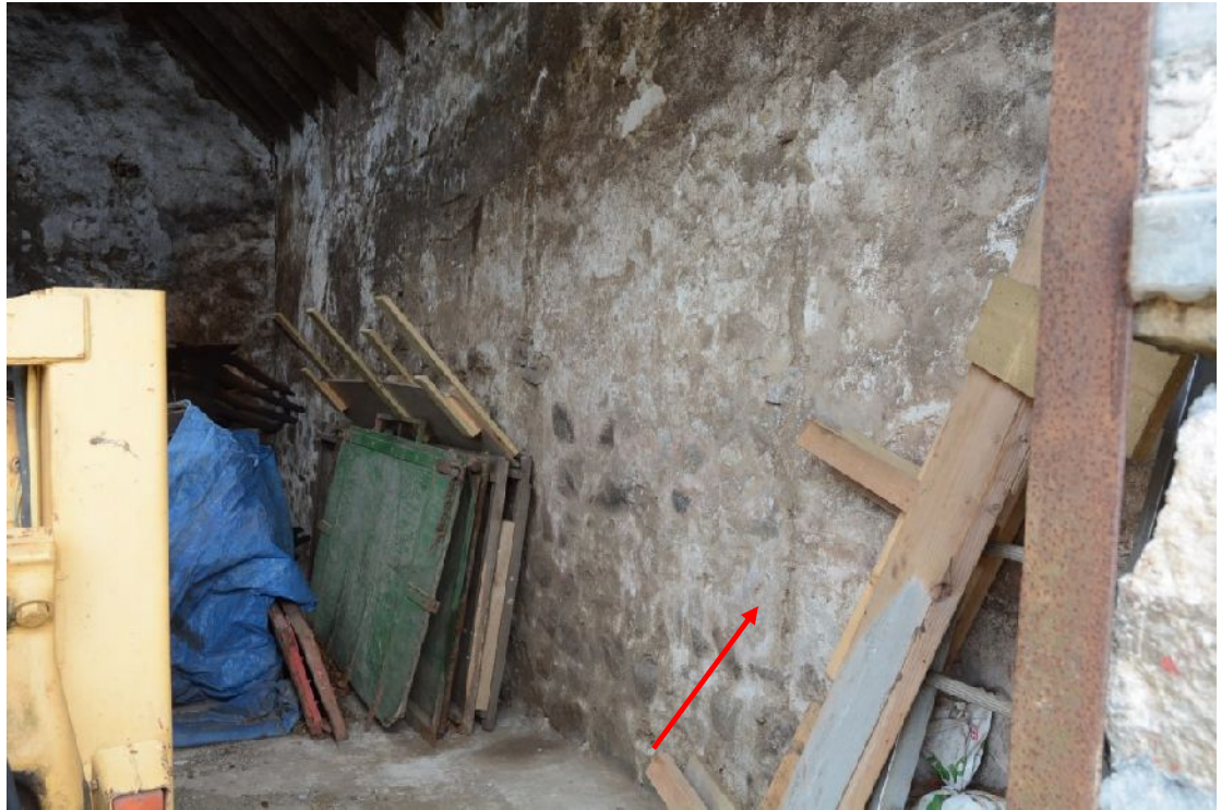
Illus 21 South Range. Inside of S wall Arrow indicates one of scars of former trevises
