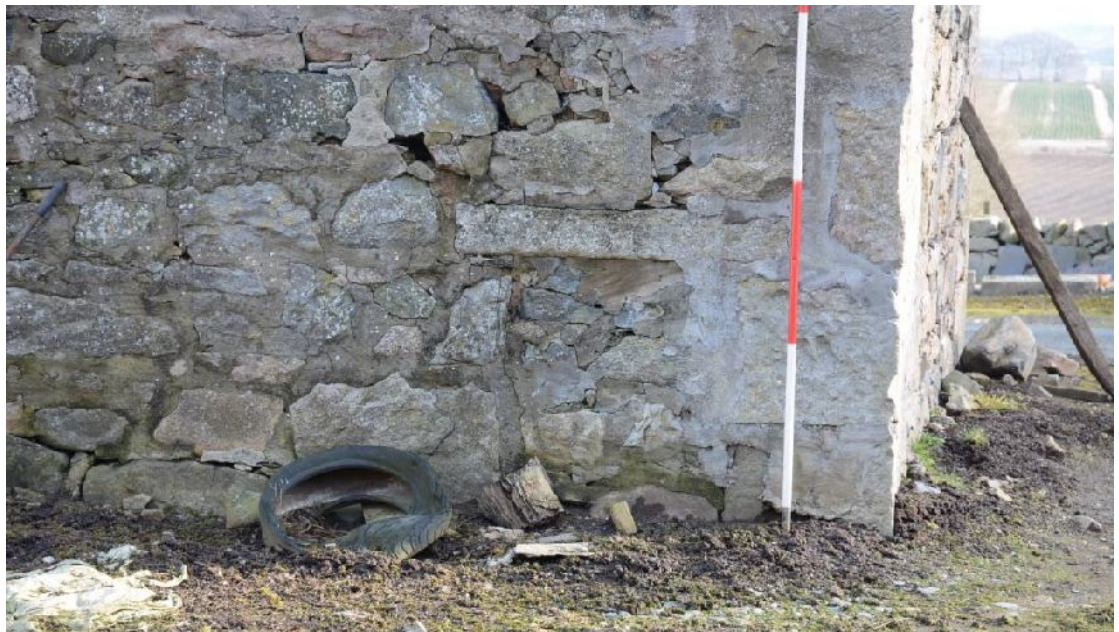
Illus 10 East Building. Detail of blocked opening F1.
