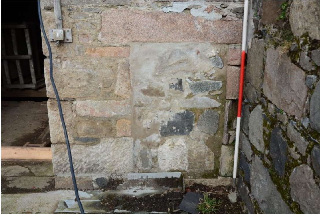
Illus 27 North Range. S wall. Blocked window W5 into lower level straw store
