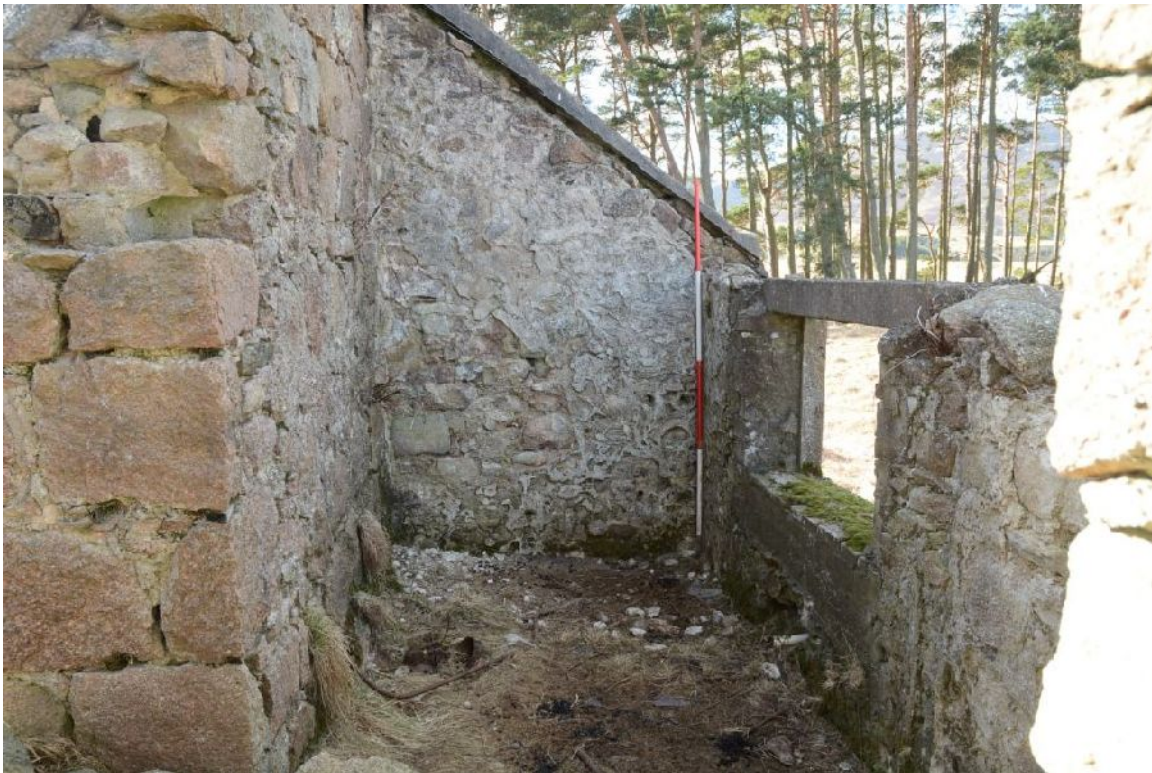
Illus 19 Outshot looking W. D3 on LHS. Raggle of partition on RHS
