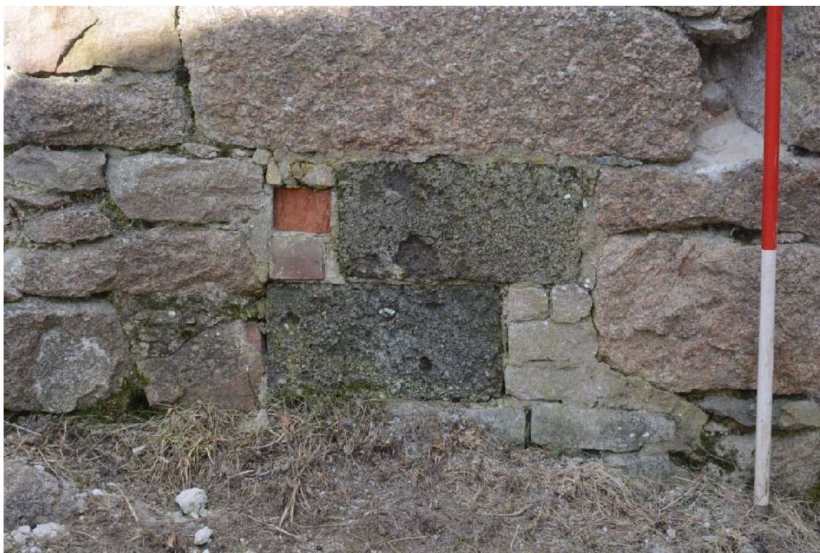
Illus 17 Detail of blocked fireplace at base of F1
