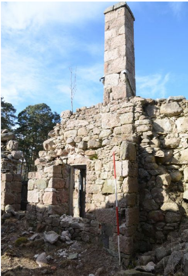
Illus 7 Chimney F1 abutting inside of N wall.
