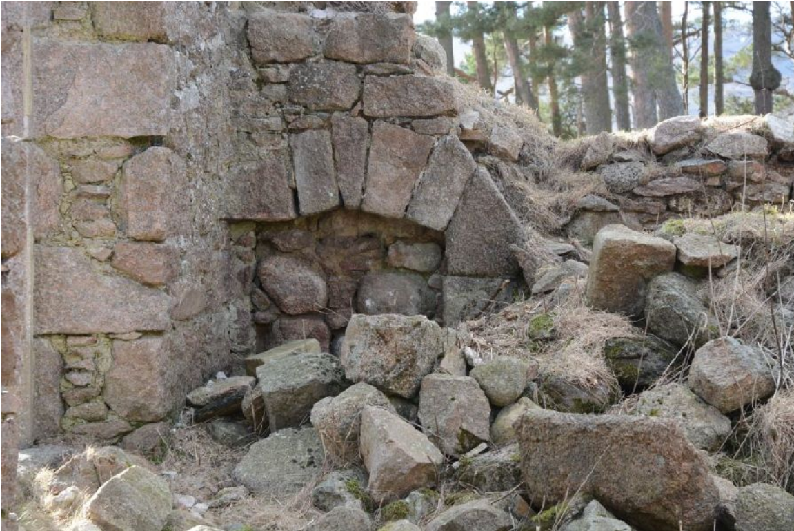
Illus 15 Detail of F2 at W end of building. Note the slightly smaller blocking of W3 partly hidden by F2.
