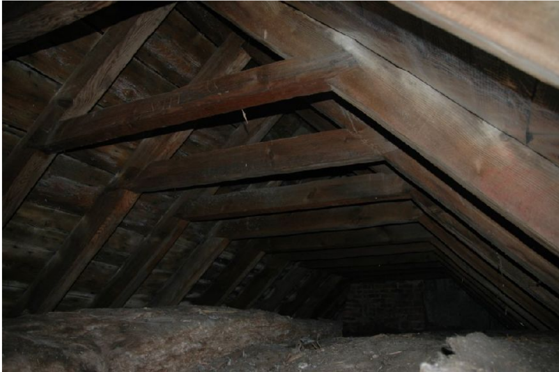
Illus 14 View of tower roof looking through hatch (looking N)
