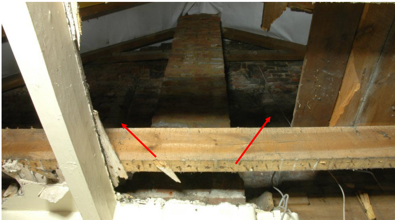
Illus 72 Kitchen, looking up at inside of S gable, showing secondary brick chimney built across brick-blocked earlier opening (red arrows mark sides of blocked opening)
