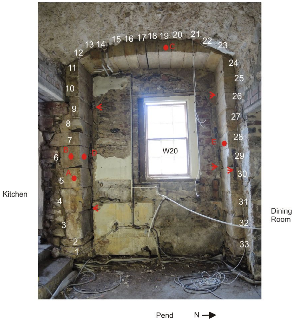
Illus 32 Detail of inside of W (street) pend arch after removal of plaster. Red dots indicate position of mason's marks and graffiti. Red arrows indicate the position of pivots (LHS) and receivers (RHS).
