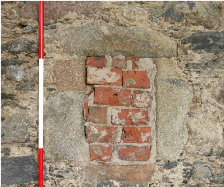
Illus 19 Blocked window W5. Above, as revealed when harling removed. RHS after removal of outer bricks. Bottom LHS debris in the hole behind window; bottom RHS inner bricks being removed.
