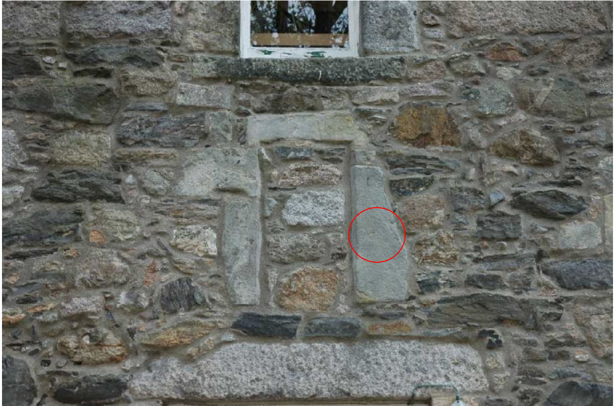
Illus 27 Blocked window F7. Red circle shows mason's mark
