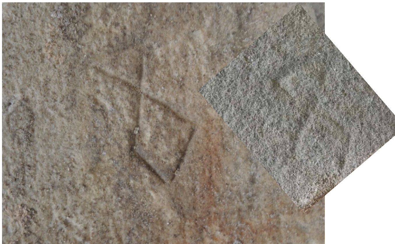
Illus 39 Mason's mark 1, on S side of inner face of W pend arch (Illus 32: Stone 6:B.) Inset: the same mark from W elevation, window F7
