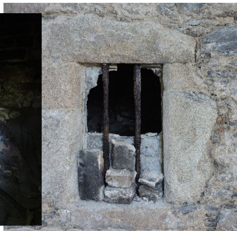
Illus 19 Blocked window W5. Above, as revealed when harling removed. RHS after removal of outer bricks. Bottom LHS debris in the hole behind window; bottom RHS inner bricks being removed.
