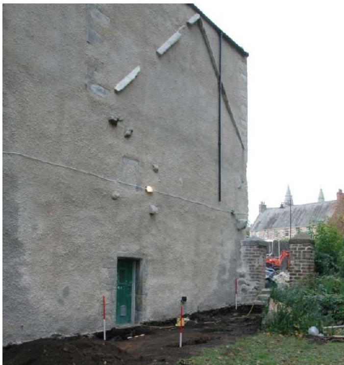
Illus 89 E wall of tower showing roof line of N range. Ranging rods in foreground indicate excavated S wall of N range; rod in background by pillars indicates surviving section of N wall
