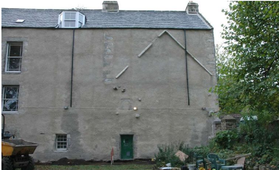
Illus 88 E wall of tower showing line of roof of N range. Ranging rods to LHS of door indicate excavated S wall of N range
