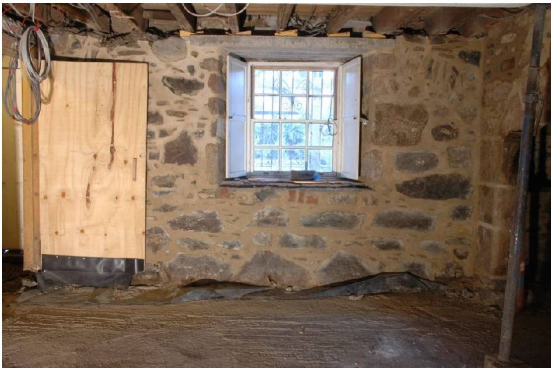
Illus 51 Dining room, E wall. Note voussoir stones to RHS of window as viewed.
