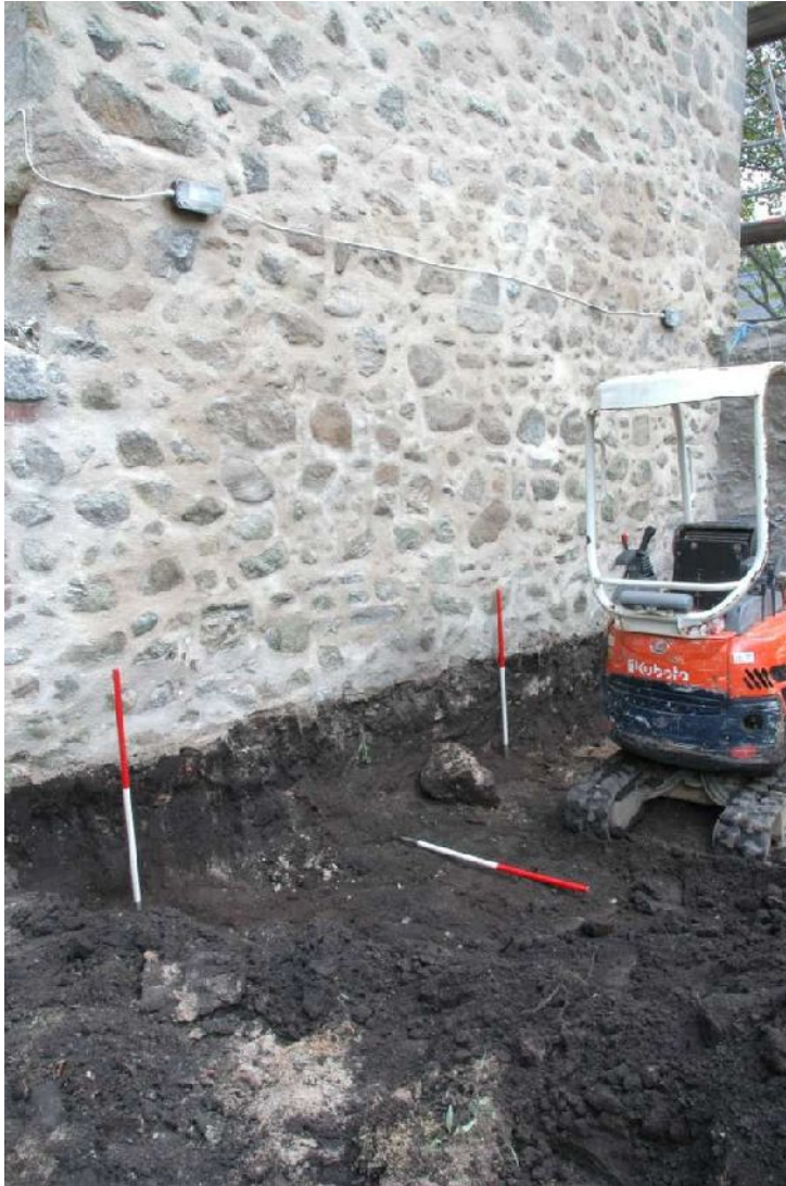
Illus 76 Garage area after soil removed
