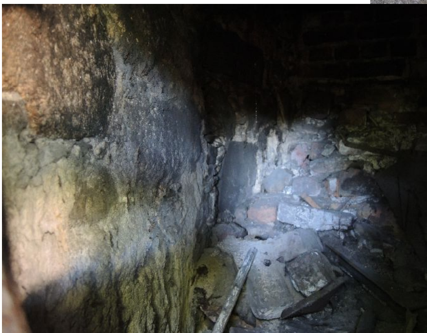
Illus 19 Blocked window W5. Above, as revealed when harling removed. RHS after removal of outer bricks. Bottom LHS debris in the hole behind window; bottom RHS inner bricks being removed.
