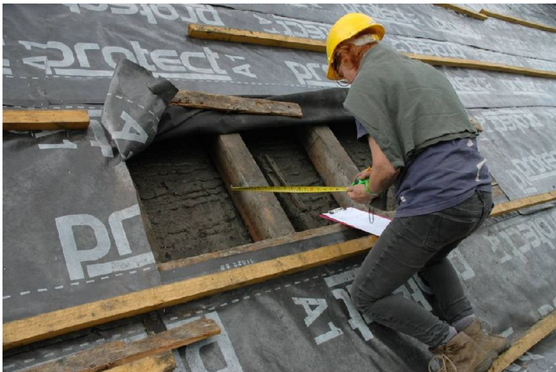
Illus 2 Recording of the roof
