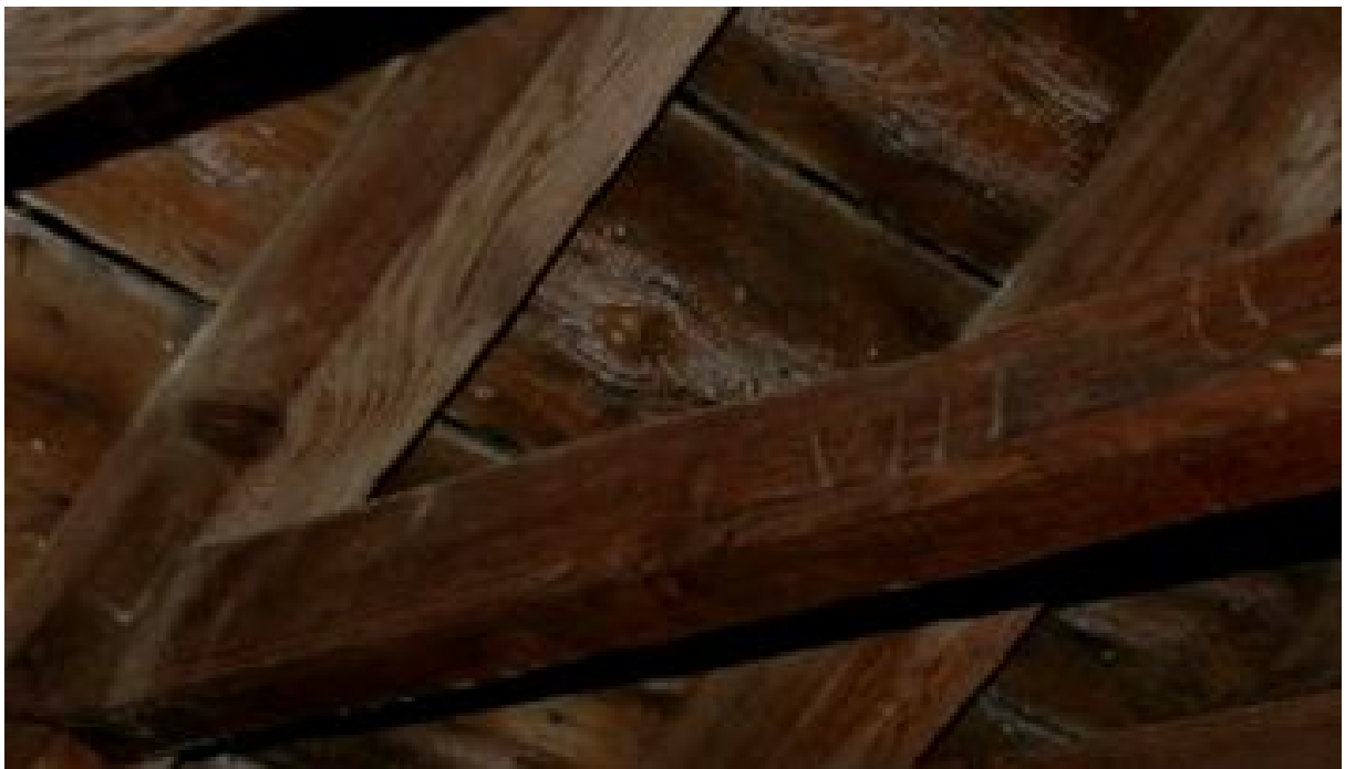
Illus 15 Tower roof, detail of carpenter's mark VIII
