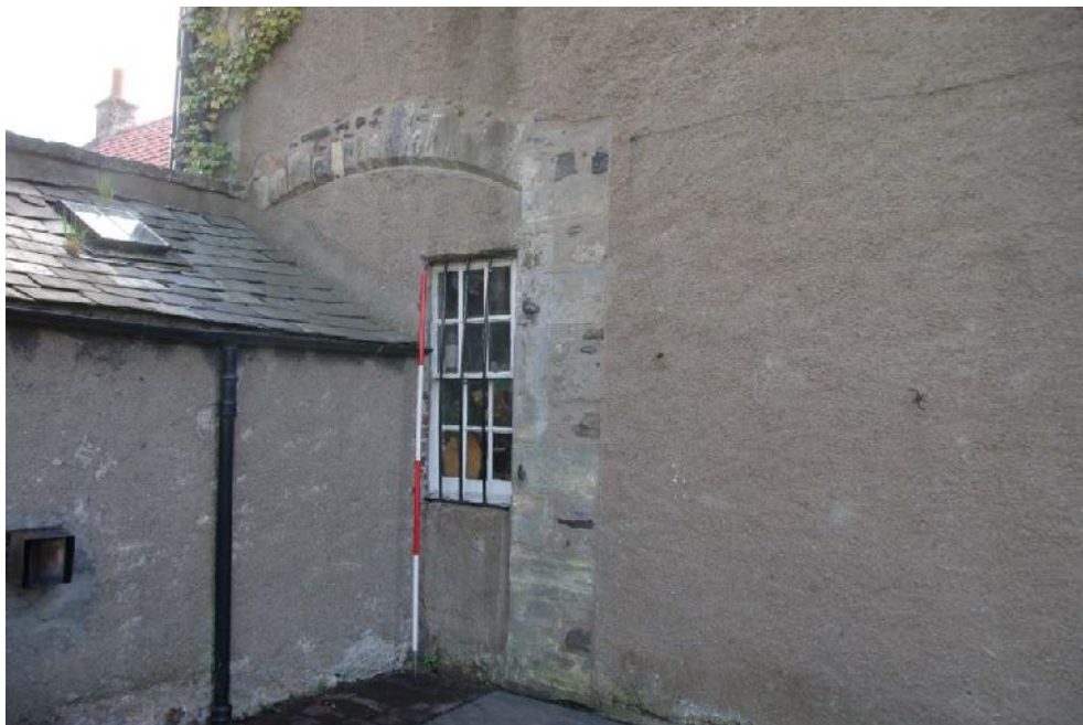
Illus 29 The outbuilding abutting the blocked pend arch.
