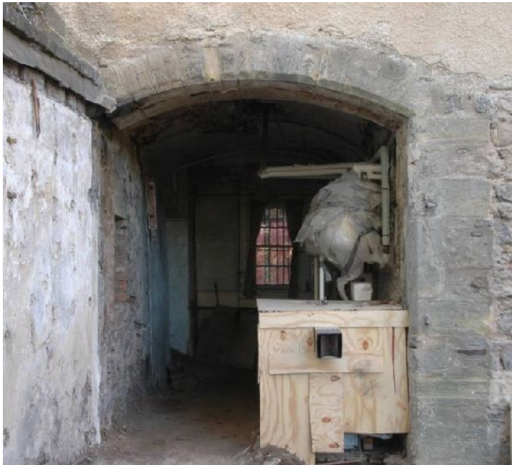
Illus 33 Garden side pend arch after removal of outbuilding, with garden wall at LHS
