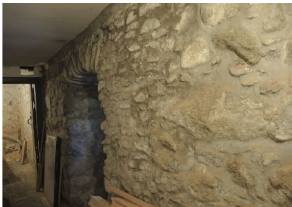
Illus 23 D2 Relieving arch on inside
