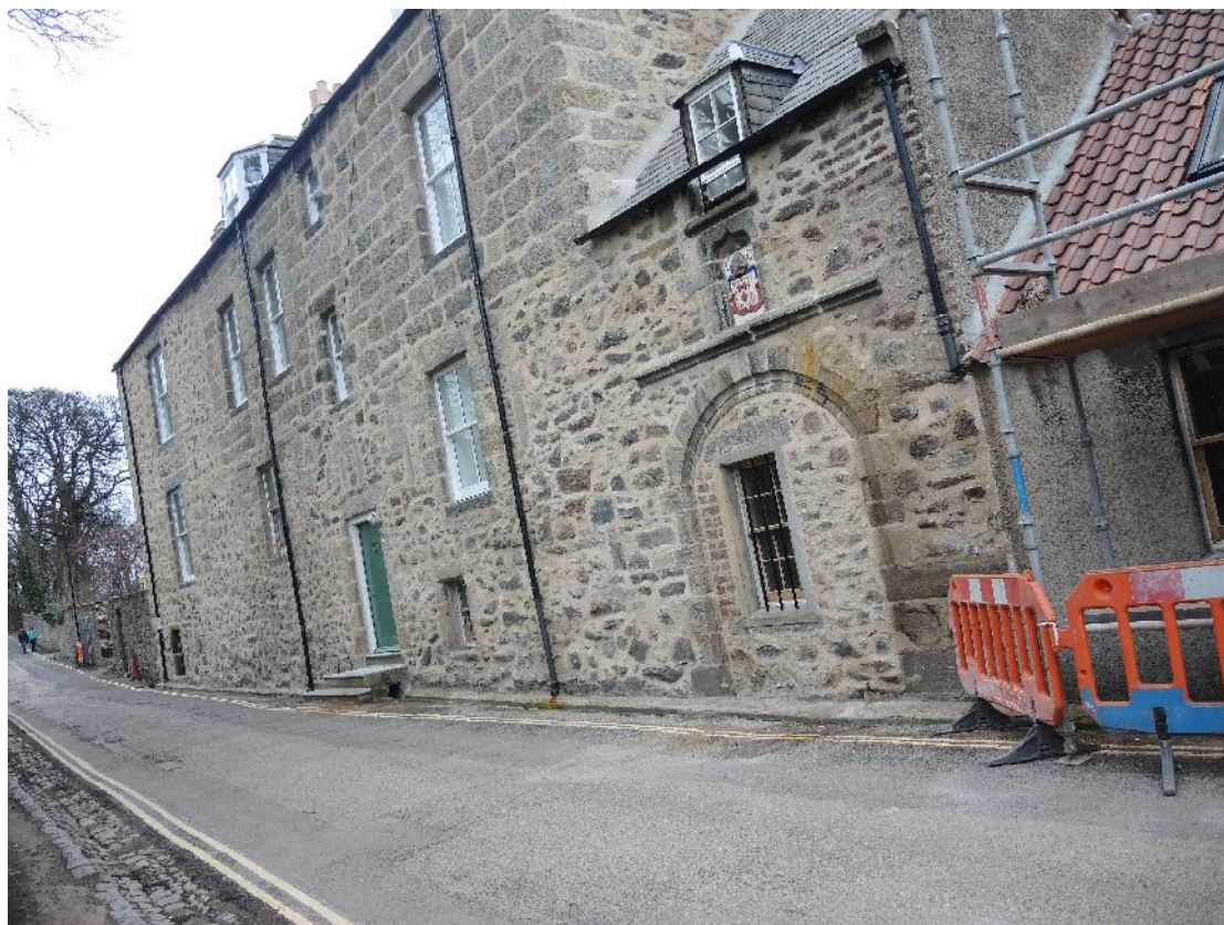
Illus 10 Street elevation showing difference in upper and lower wall
