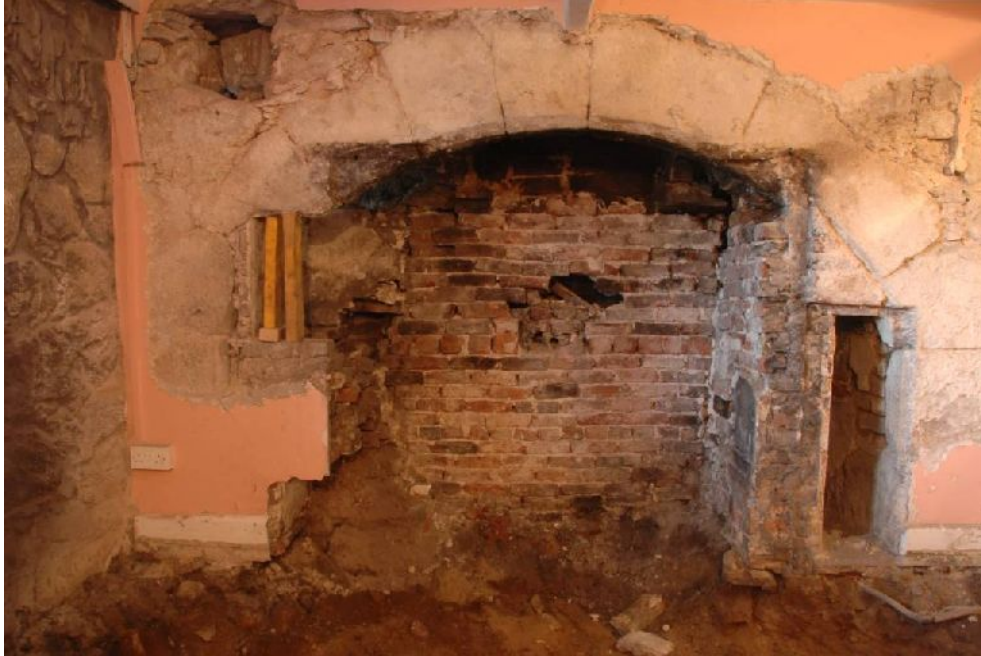
Illus 65 Later fireplace with tiles removed to show brick (F15). F17 to RHS. F20 by prop to LHS.
