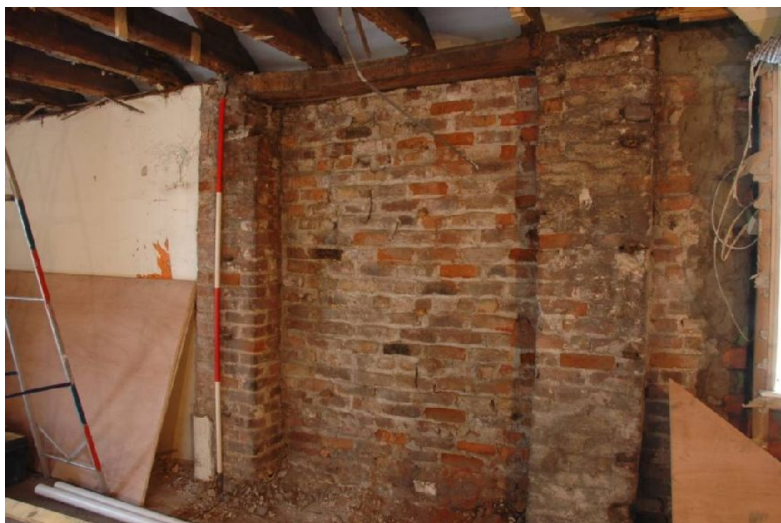
Illus 71 Kitchen. Brick-blocked wide door (F11) in street (W) wall, with wooden lintel
