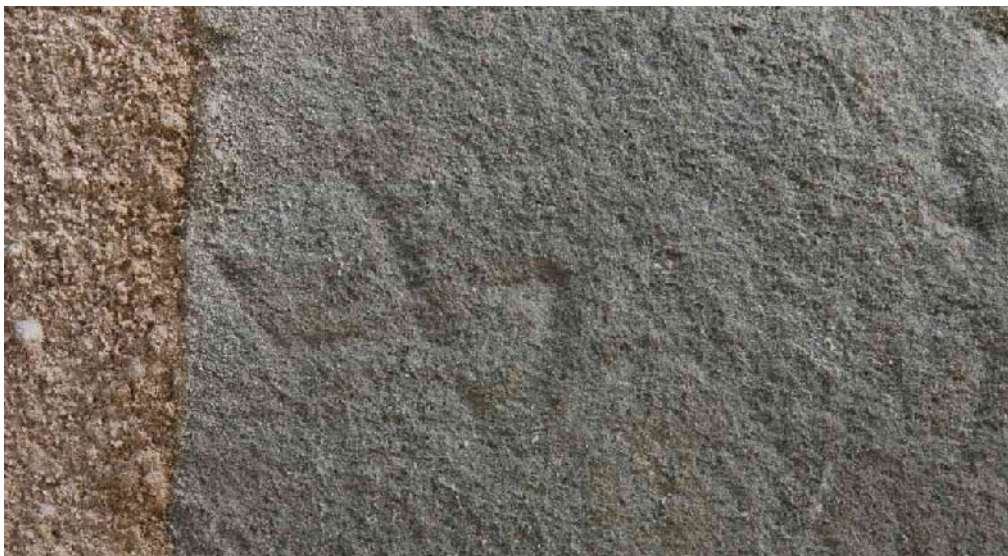
Illus 28 Detail of mason's mark on window F7
