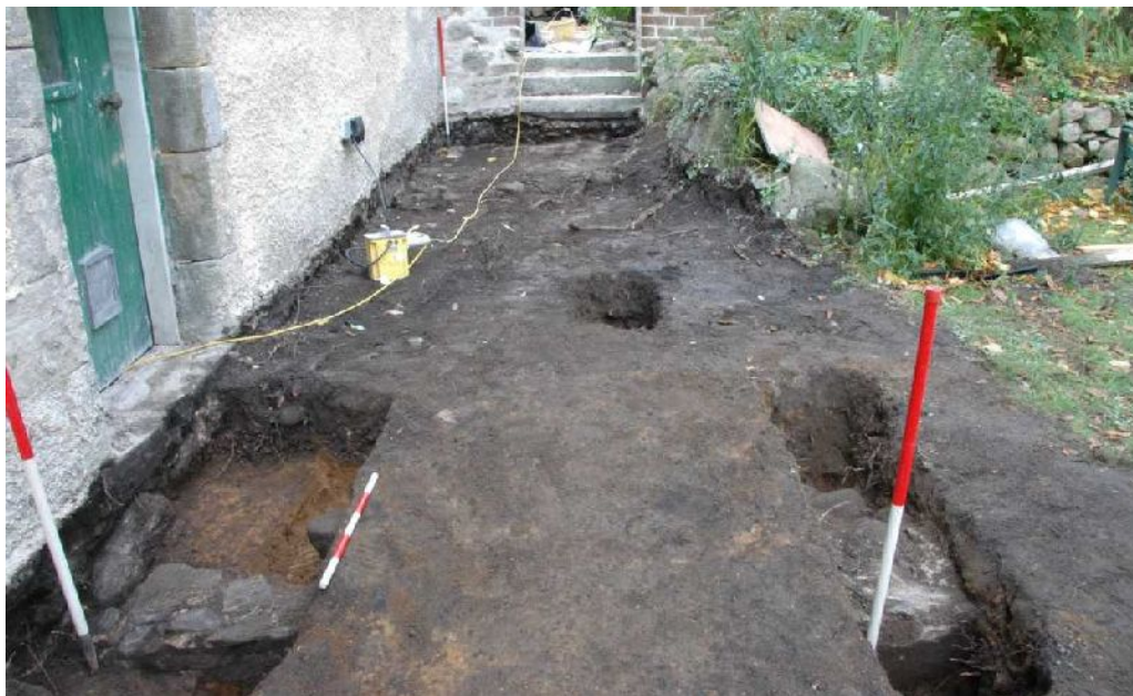
Illus 82 Sondages 2 and 3 showing foundations of S wall of N range (by ranging rods). Ranging rod in background shows surviving line of N wall of N range.
