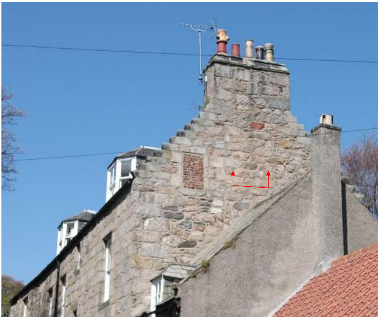
Illus 11 S gable of W range with blocked window W41 and in centre to RHS of window, the more regular blocks of old chimney marked by red arrows.
