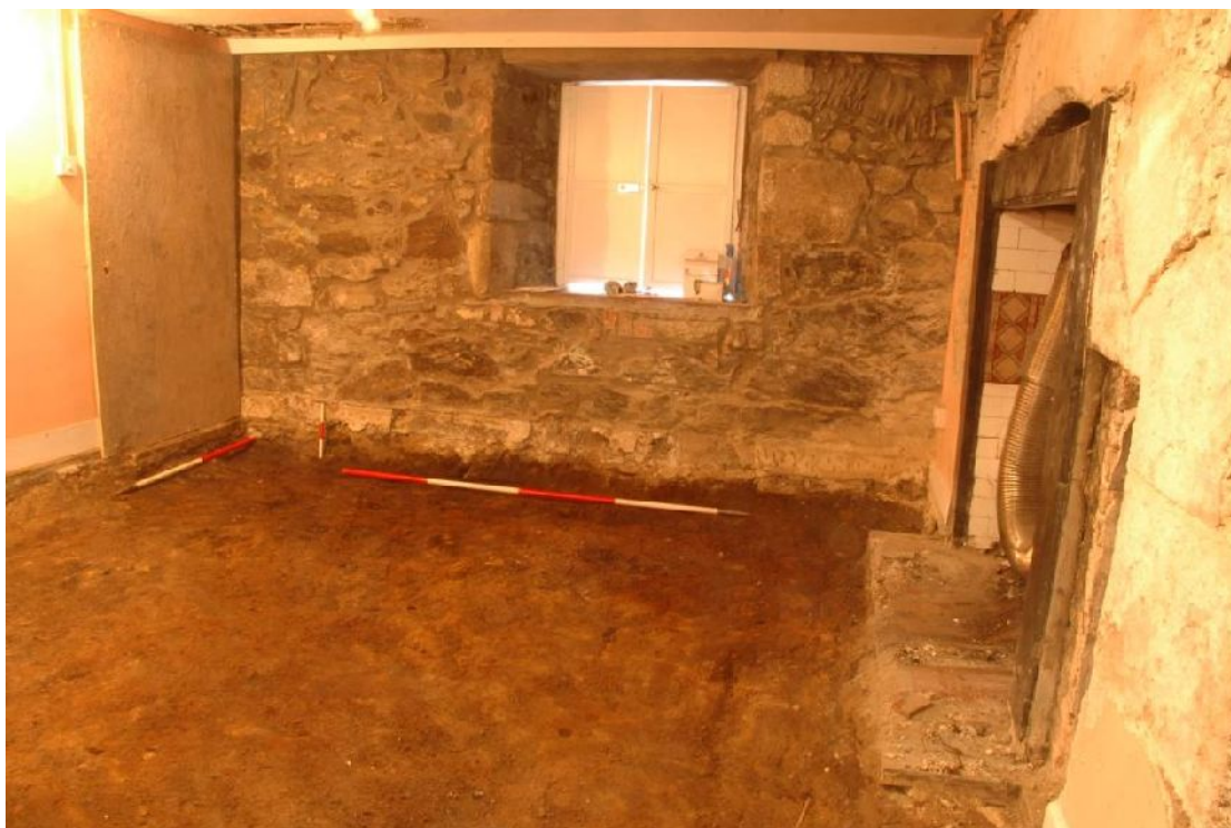
Illus 46 Dining room with floors removed. Patches of dark humic material visible near ranging rods.
