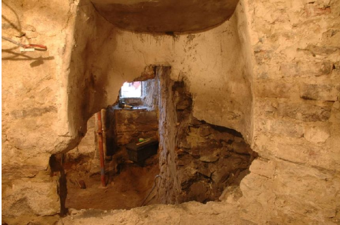
Illus 63 Alcove F16 broken through to fireplace
