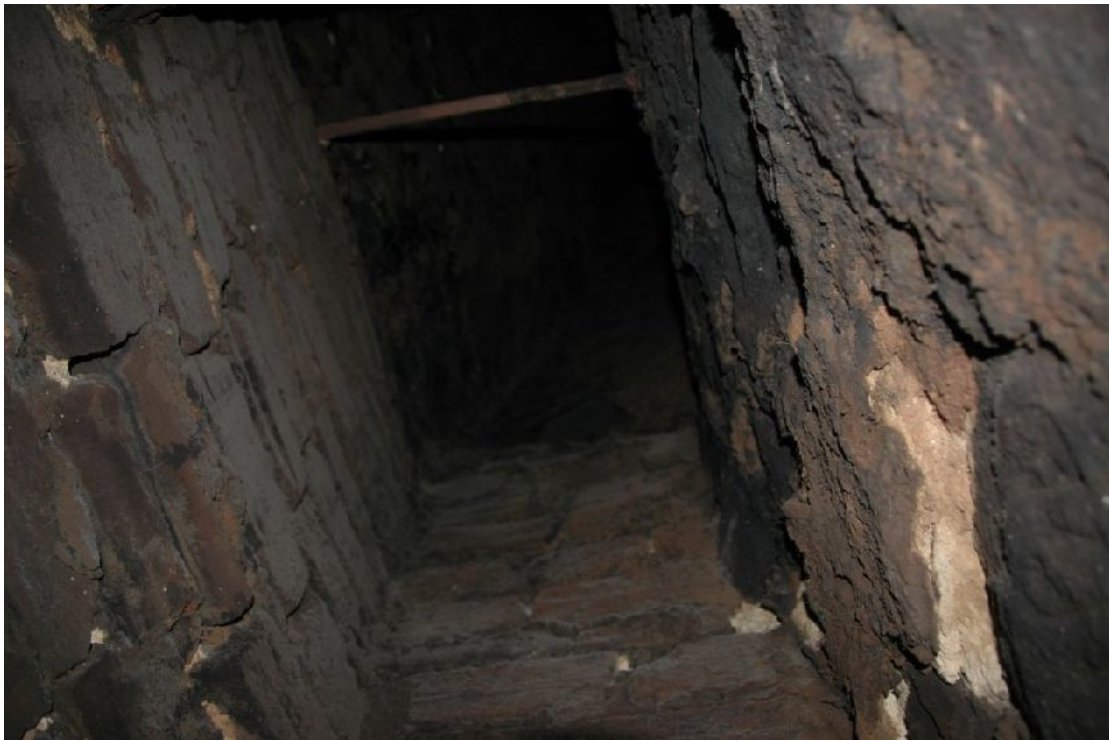
Illus 66 Looking up chimney as narrowed by secondary brick lining
