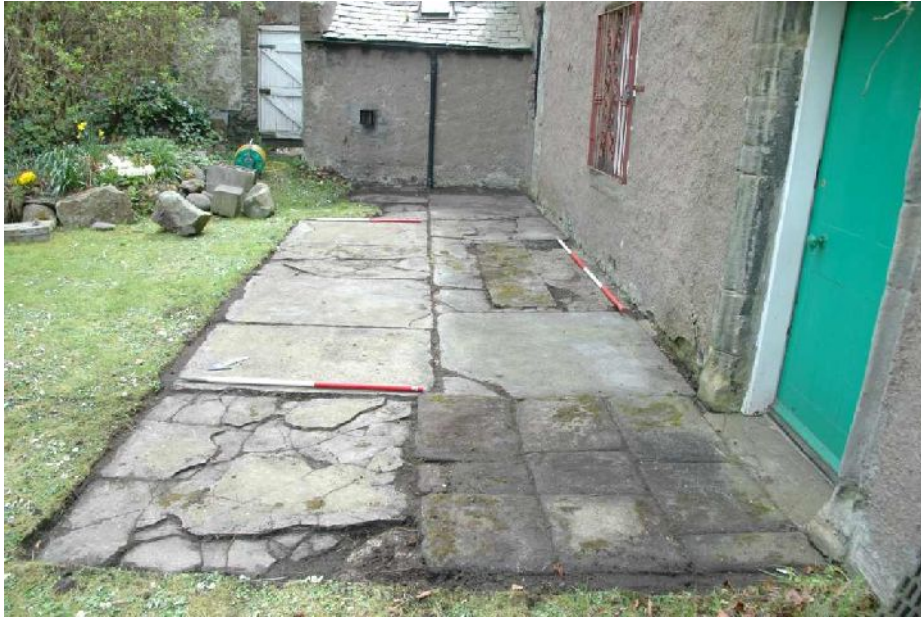
Illus 79 Paving of slate slabs
