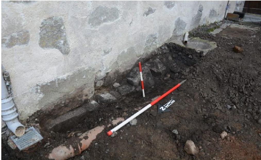
Illus 57 Cross Range W wall. Detail of exposed foundation
