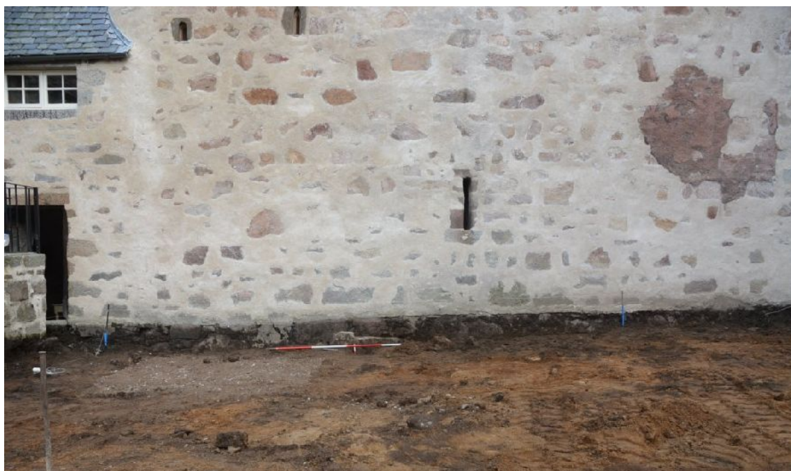
Illus 55 Tower W wall. Ranging rod indicates position of projecting natural boulders.
