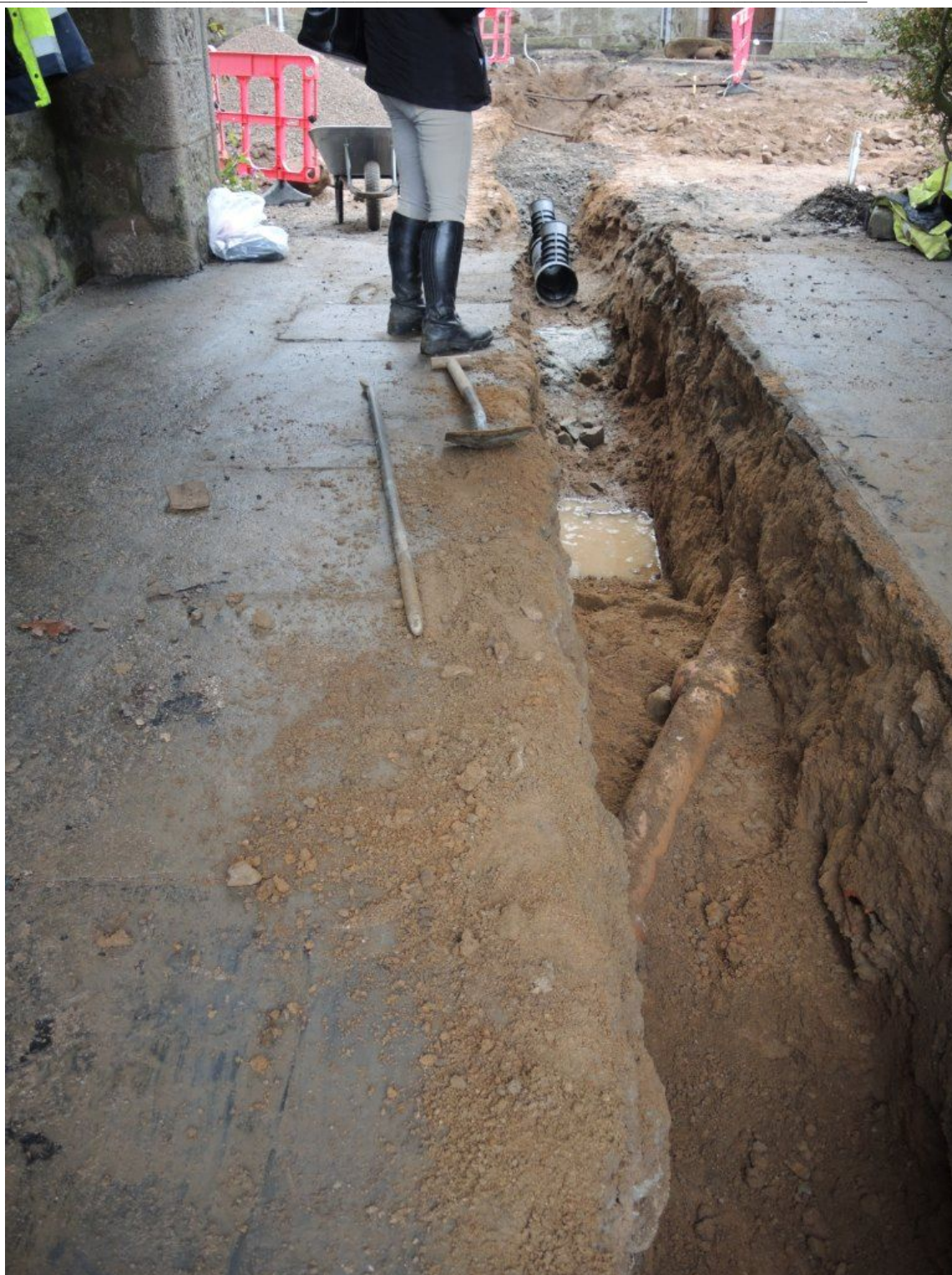
Illus 60 View S through archway showing some of pipes.
