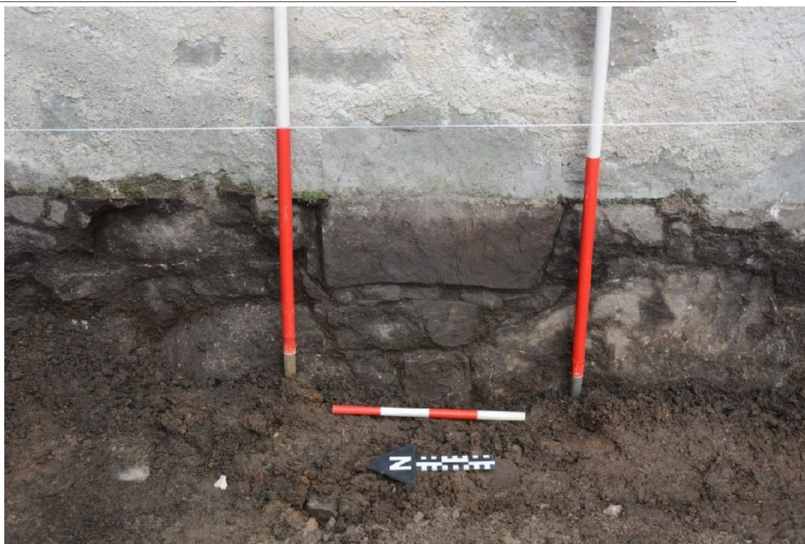
Illus 53 W wall of tower. The two vertical ranging rods flank the possible blocking of drain outlet from intra-mural garderobe. Detail of blocking
