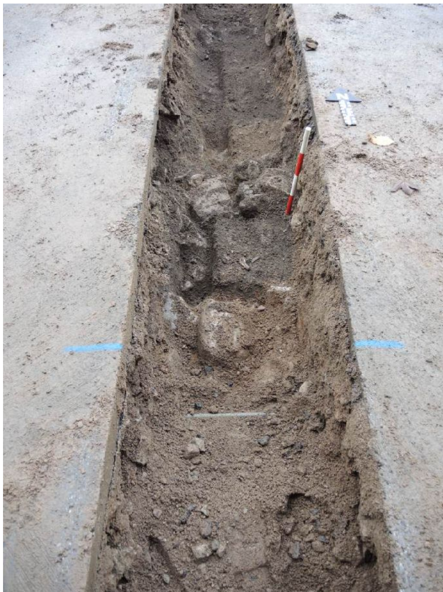
Illus 59 Backfill of pipe cut showing dark fill, possibly backfill of 19 th -century layers.
