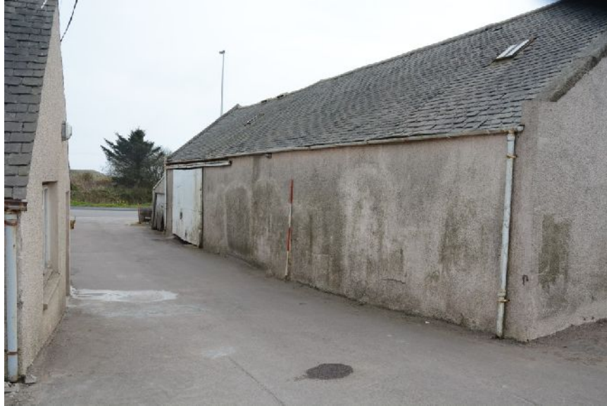
Illus 10 Building 2. S steading. N elevation. (Photo 20)
