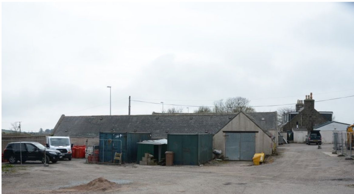
Illus 14 Building 3. N steading. N elevation with house (Building 1) beyond on RHS. (Photo 18)
