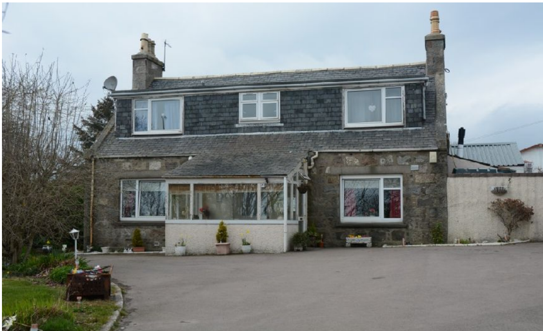
Illus 6 Building 1. House. E elevation (Photo 26)
