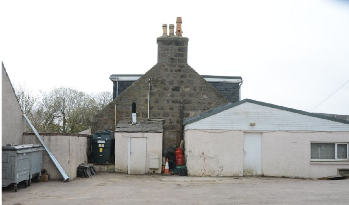
Illus 8 Building 1. House. N elevation. (Photo 30)
