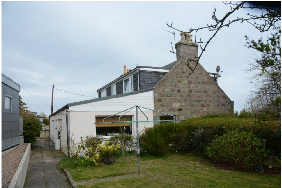
Illus 7 Building 1. House. S elevation. (Photo 28)
