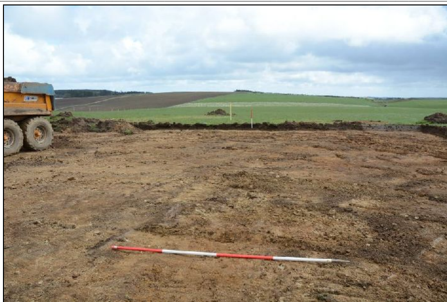
Illus 7: Area of hard standing, looking E. The upright stick E of the hard standing marks the location of the turbine base
