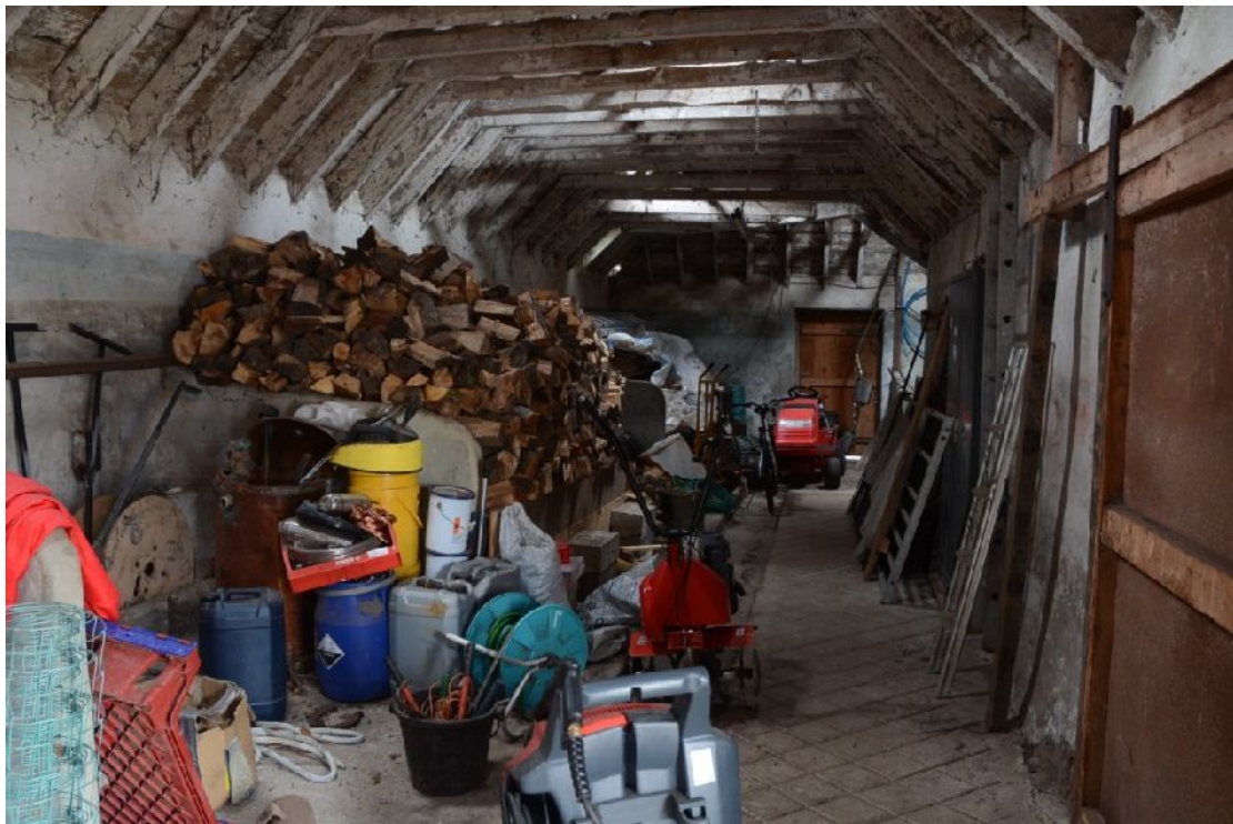
Illus 7 W Range. Interior looking N showing concrete cow stalls.
