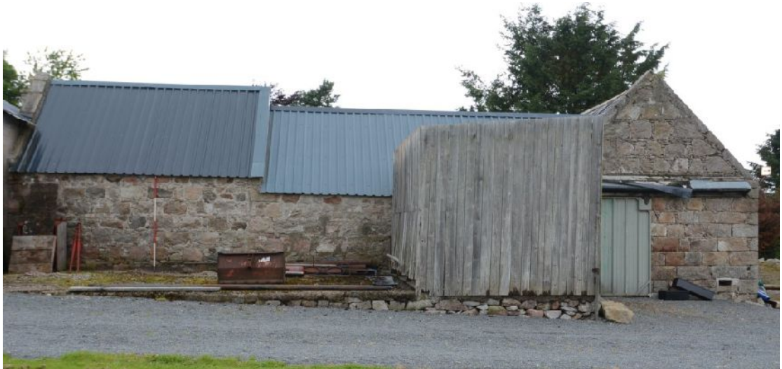
Illus 8 From L to R. E Range, Buildings 1 and 2 and E gable of N Range.
