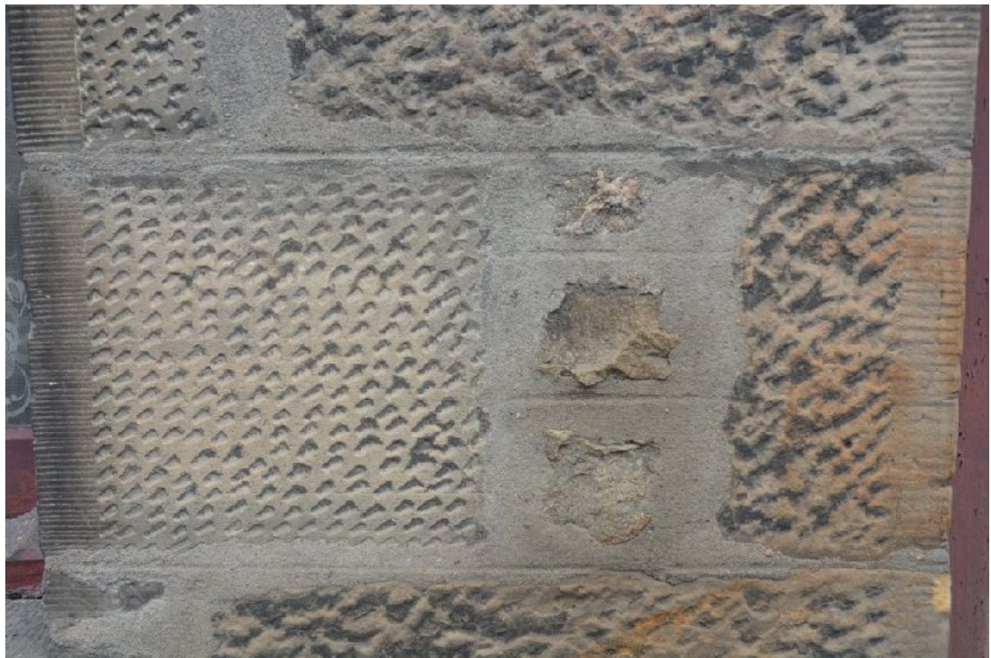
Illus 11 Detail of rybats on W3 (LHS) and D1 (RHS). Note the less weathered and more separated tool marks on window W3.
