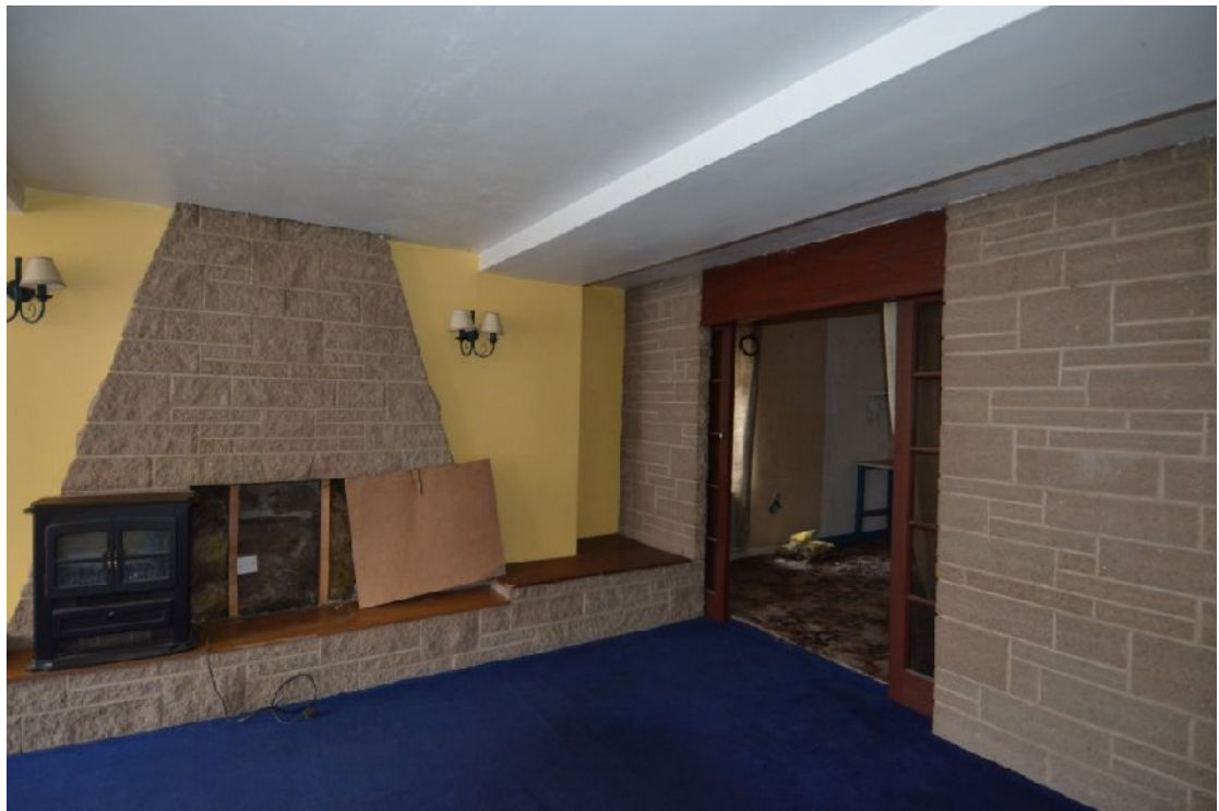
Illus 10 Room 3, looking towards NE corner. Note narrower external wall in corner and the line of original E wall across the ceiling.
