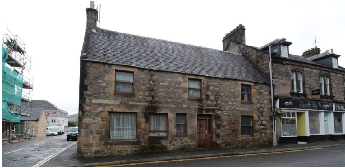
Illus 4 W frontage on New Street
