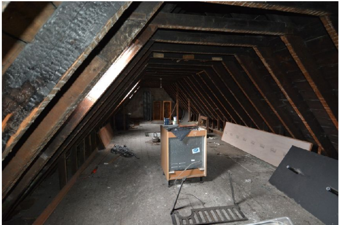
Illus 16 Attic of W wing looking S. Note charring on rafter in foreground
