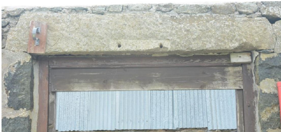
Illus 16 Detail of re-used stone in lintel of door D2
