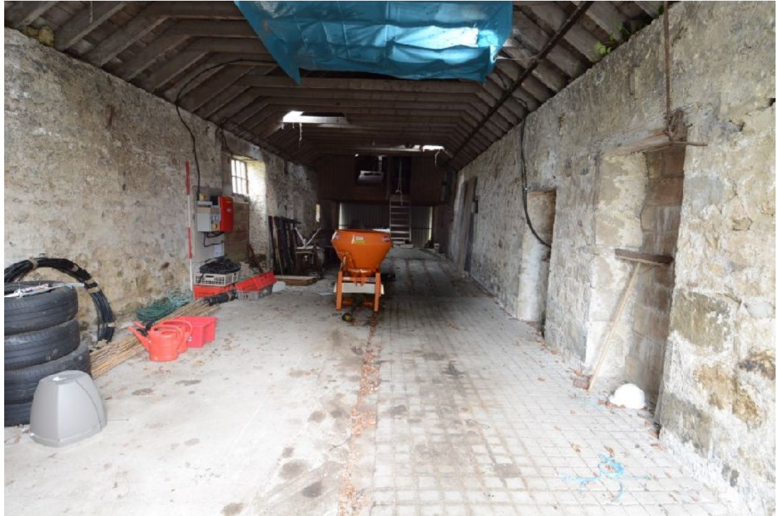
Illus 12 B2 internally looking N. Blocked D11 to RHS
