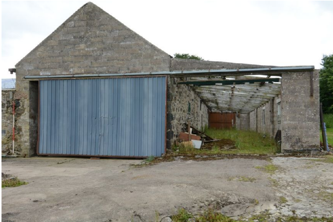
Illus 9 N end of B1 (RHS) and B2
