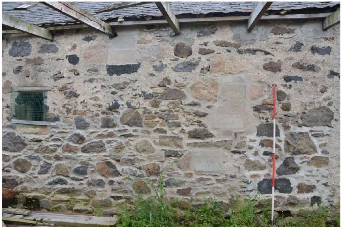
Illus 10 Outside of W wall of B2 (from inside B1). Openings associated with mill from LHS to RHS: F4, F3, F2 and above F1.
