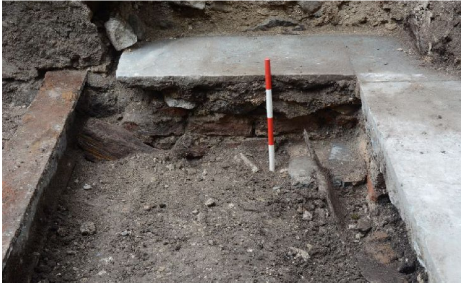
Illus 12 Detail of E end of I-beam slotted into main wall. Note vertical timbers in building rubble infill.
