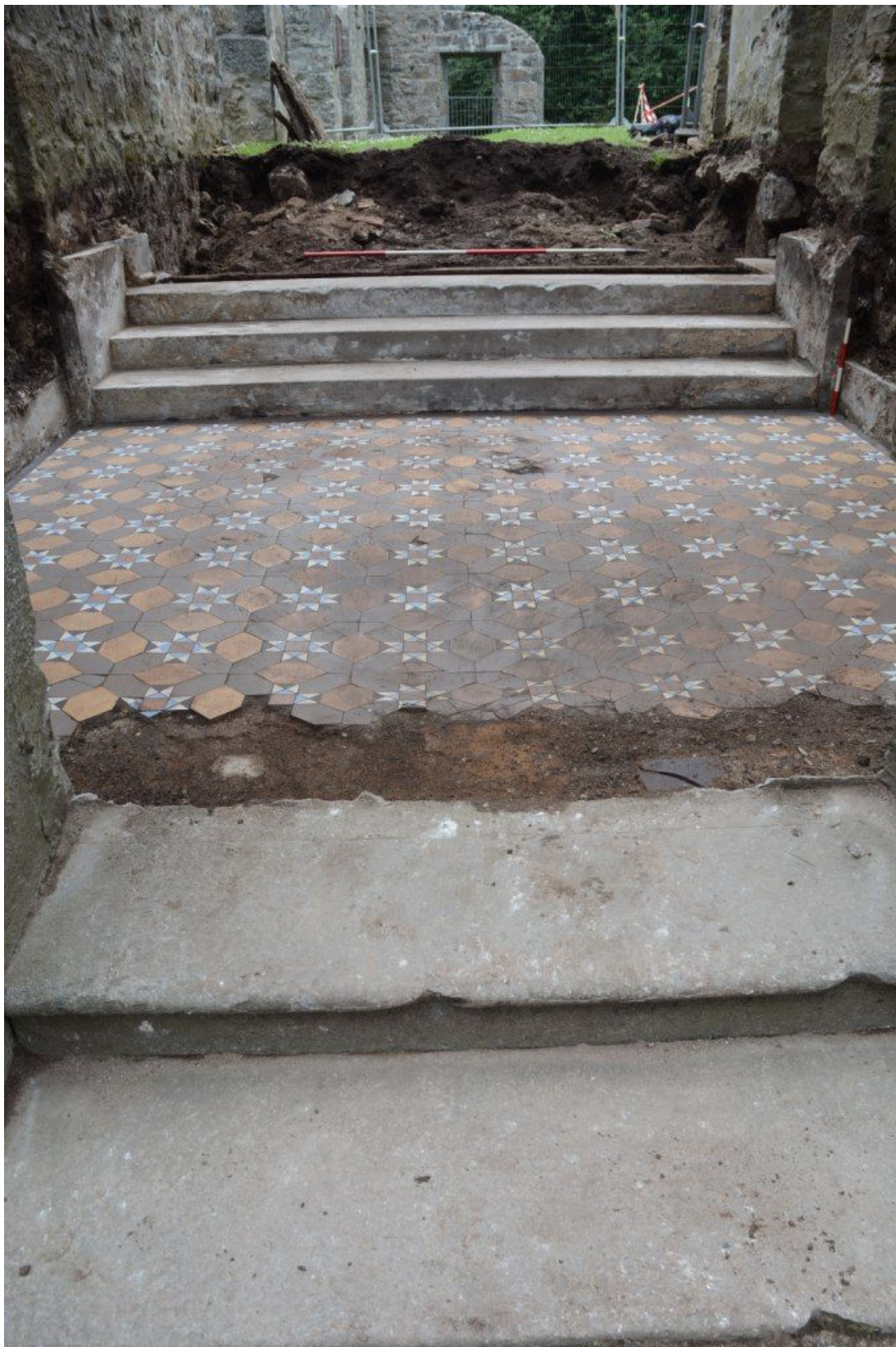
Illus 4 View of tiles in lower area of Entrance Hall, looking N
