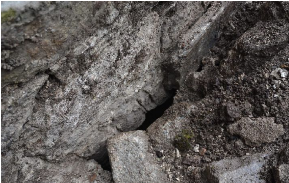
Illus 13 Detail of arch built into base of wall
