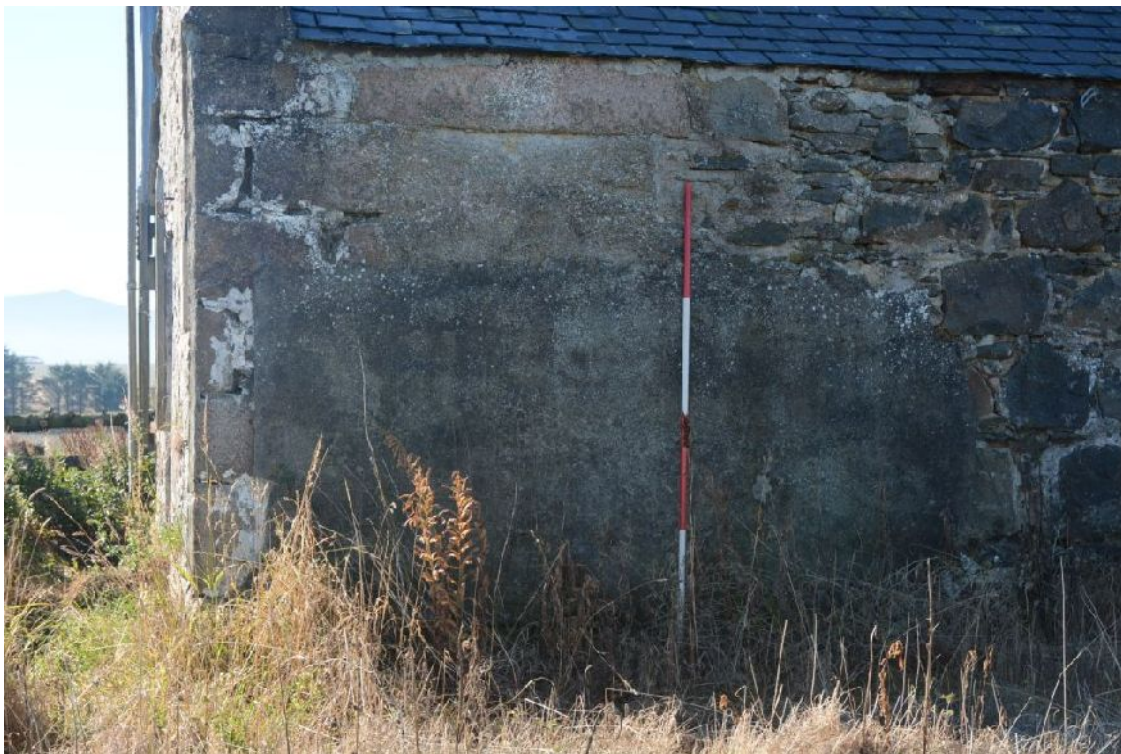
Illus 9 N wall N Range. Blocked opening F4
