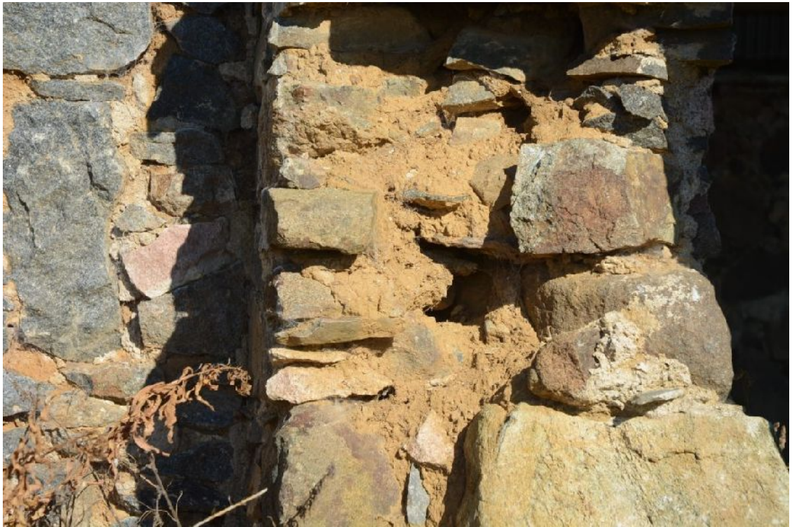
Illus 13 Detail of core of broken S end of wall of W range showing clay binding in core.
