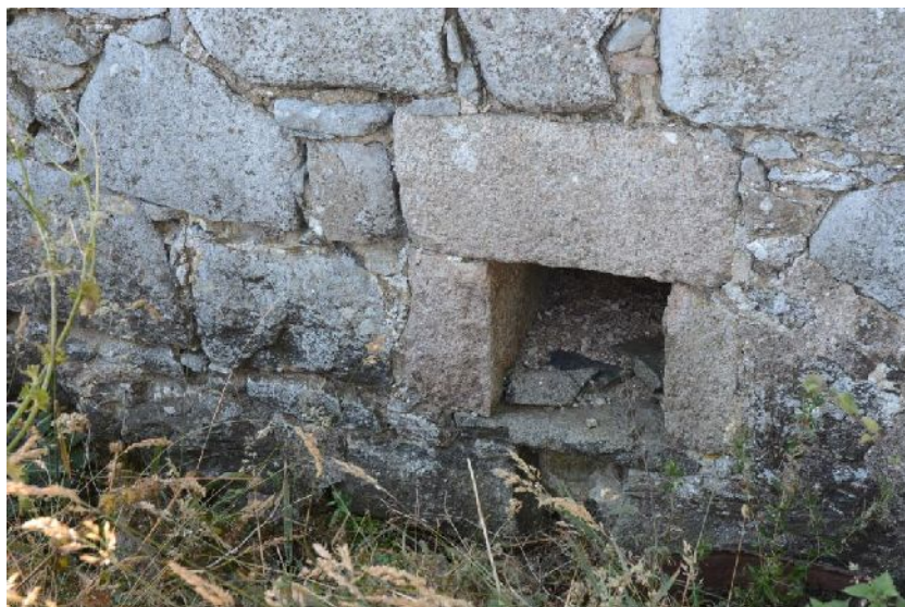
Illus 22 Mill wheel axle hole (F1)
