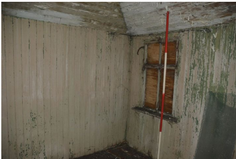
Illus 14 Interior NE extension. B1.
