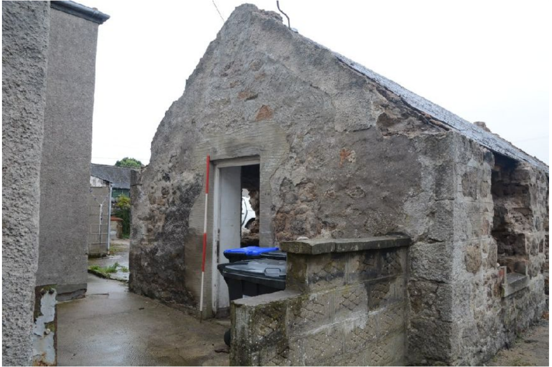
Illus 9 SW gable and secondary door D2
