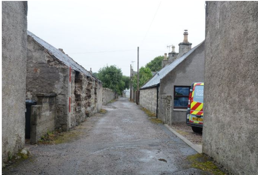
Illus 15 Looking from High Street up lane with cottage on LHS.
