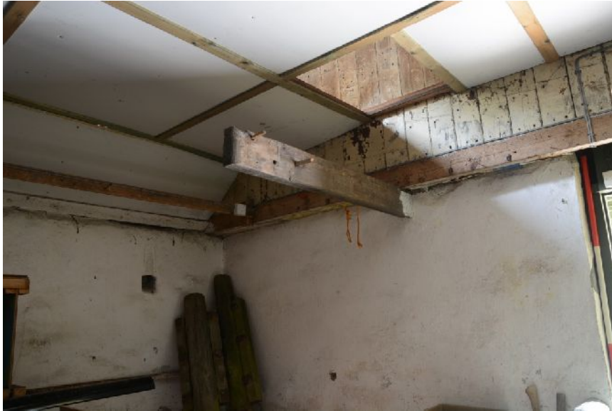
Illus 11 Detail of the timber loft wall and projecting timber.
