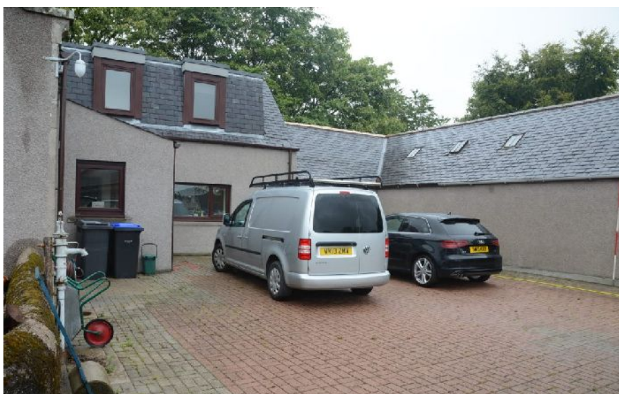
Illus 7 Looking W at extension of house into line of former steading. The steading in the survey is on RHS
