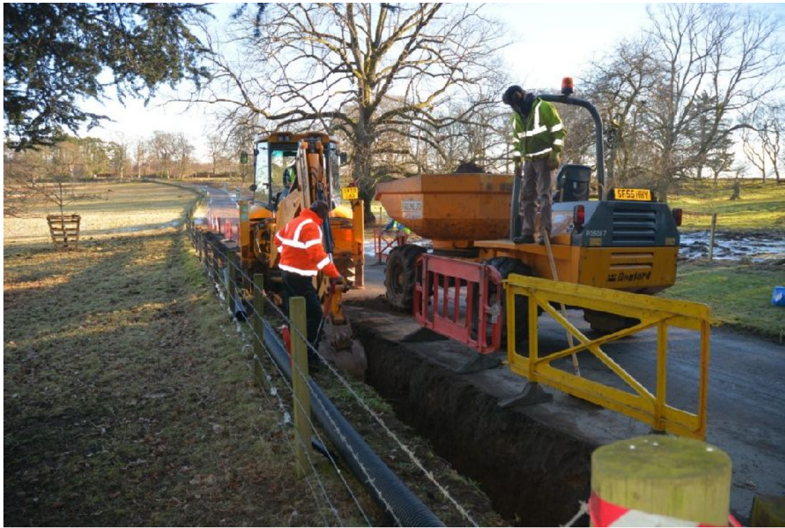
Illus 1 Cutting drain trench 1
