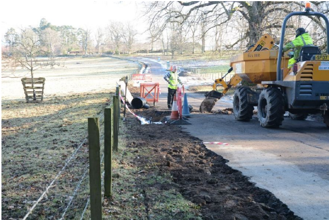
Illus 3 Thin layer of topsoil recovered over gravel in drain trench
