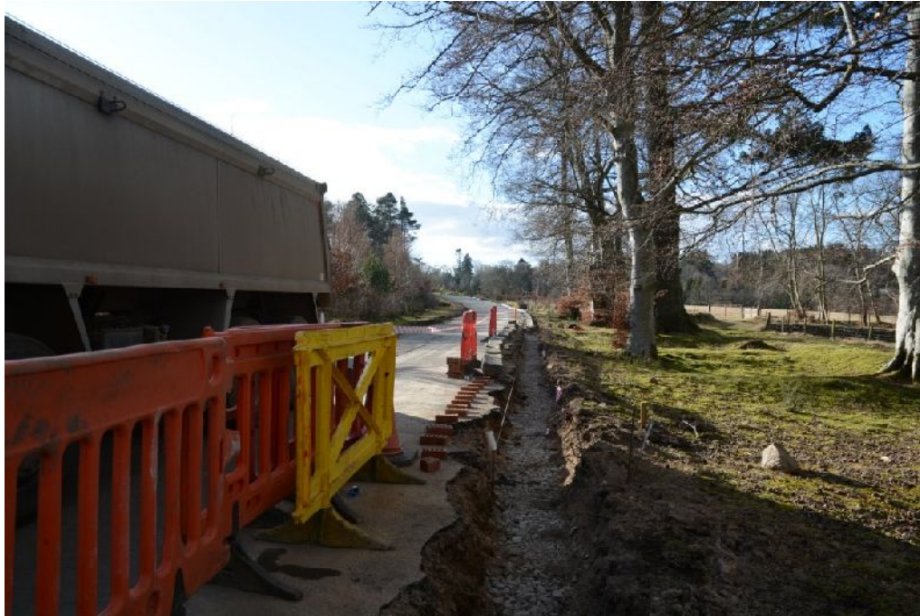
Illus 13 Kerb trench at N side of drive beside rig and furrow (which is just visible to RHS of trees).
