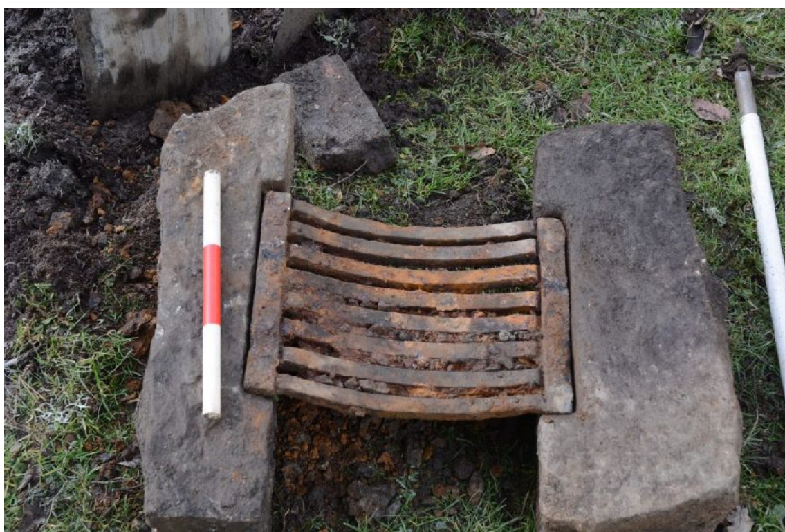
Illus 12 Stone surround and iron grill displaced from drain sump 27
