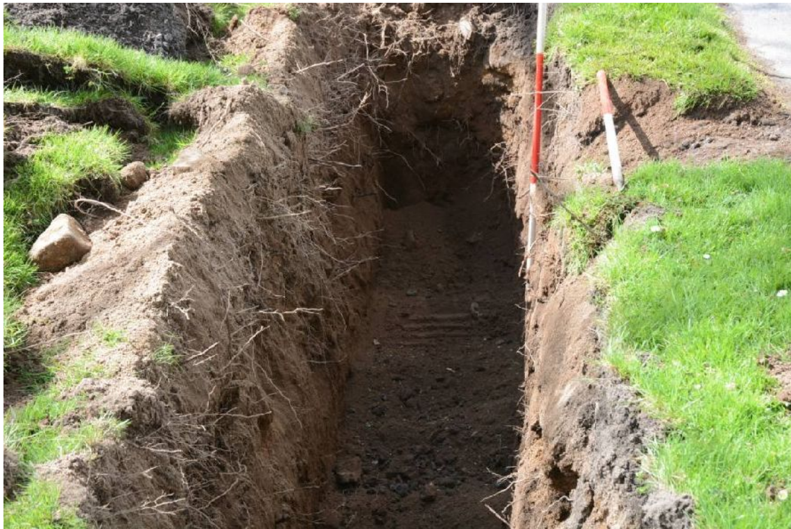
Illus 2 Detail of grip 9 showing depth of build-up.
