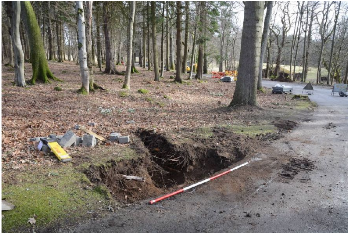
Illus 1 Drain location 5 looking SE
