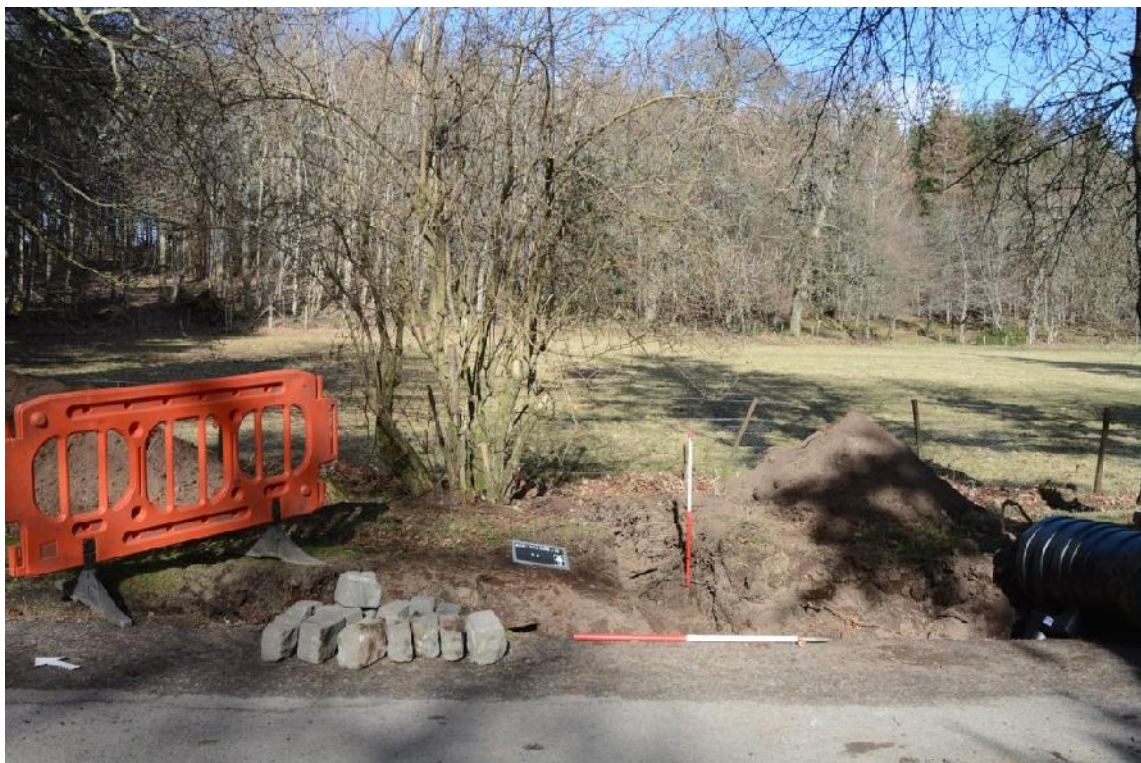
Illus 5 Drain location 14 looking N across Warren Field
