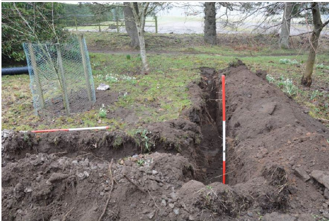
Illus 4 Drain location 1 with Overflow Car Park in background, looking N
