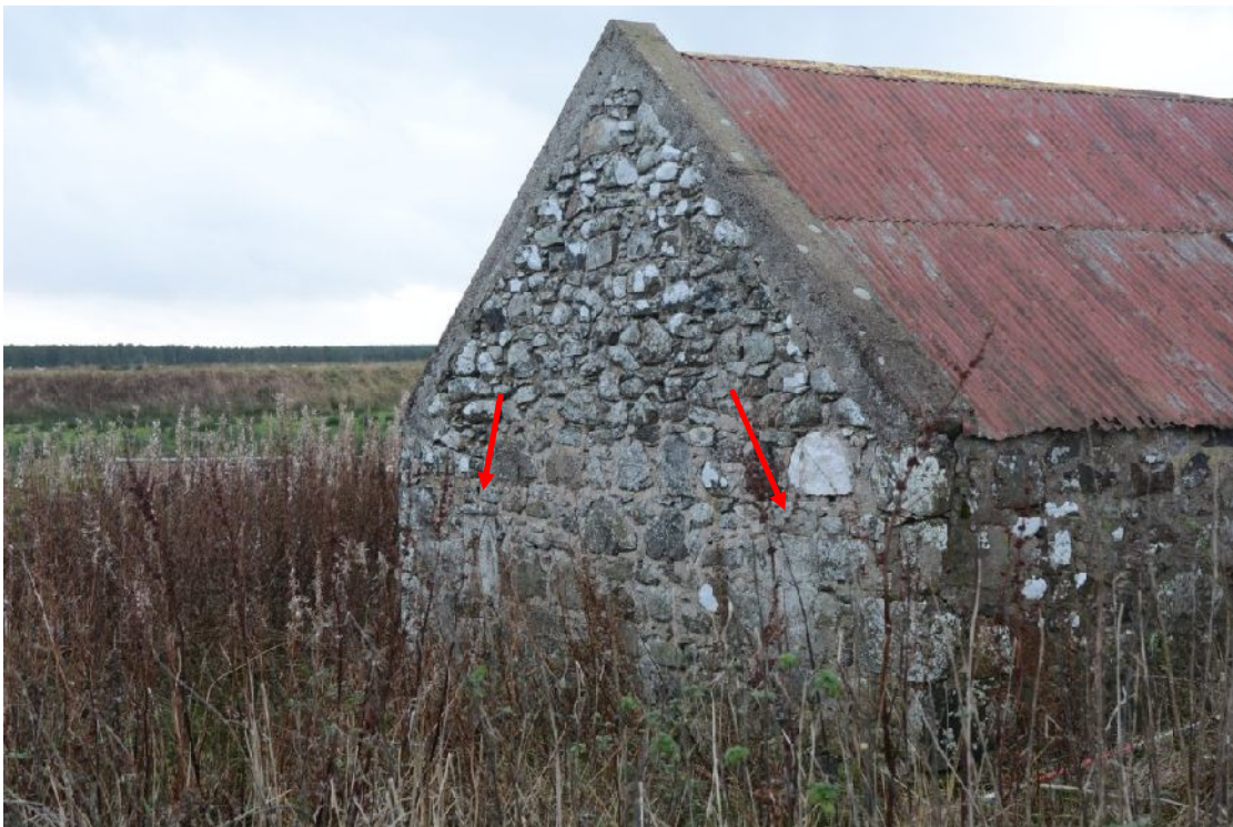
Illus 6 E wall with blockings F1 and F2 (marked by arrows)
