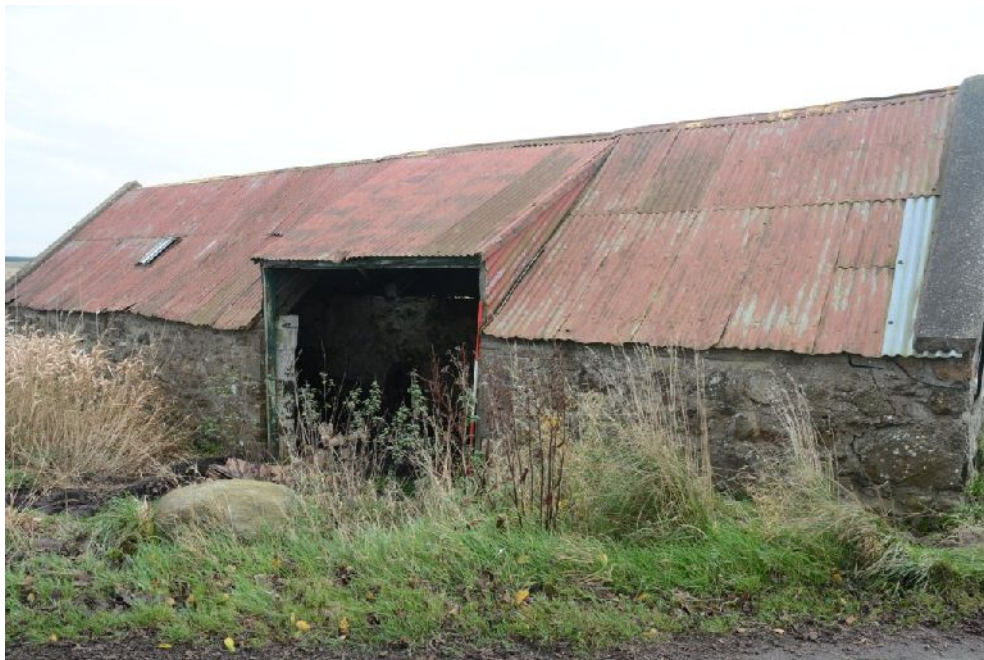
Illus 5 N wall and door D1
