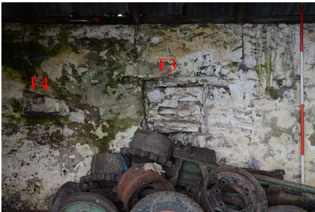
Illus 9 Blocking F3 and slot F4 on inner face of S wall.
