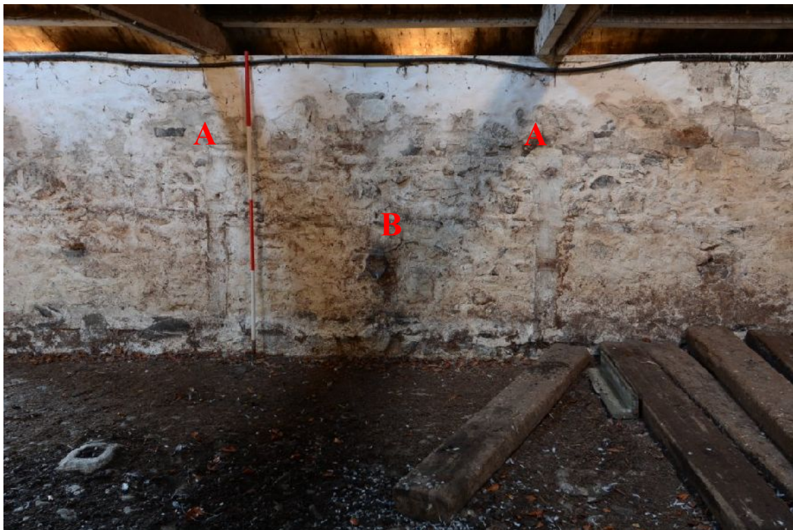
Illus 11 Detail of trevis scars (A) of cattle pens on S wall of N range (For position compare to preceding photograph). Note drinker brackets (B)
