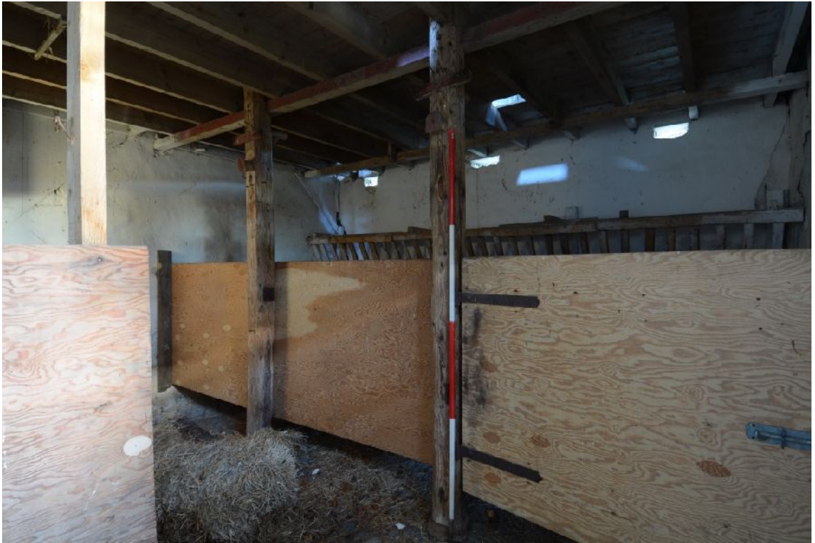
Illus 18 Stable looking E/NE. Although plywood doors are modern, the hind posts of trevises are original. Not hay rack and air vents.
