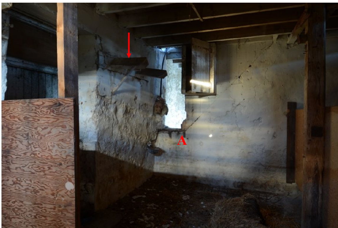
Illus 20 looking NW in stable. Arrow indicates harness supports. A= opening to stair to loft
