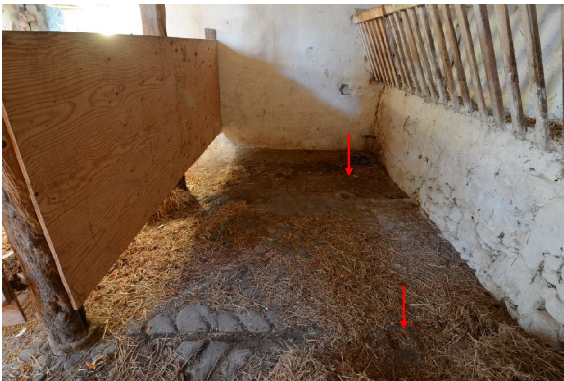
Illus 19 Looking N in stable.. Arrows indicate the central supports of trevises
