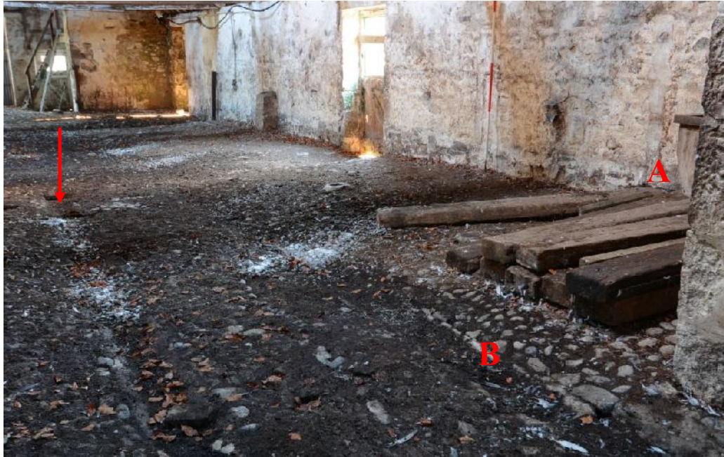
Illus 10 Looking E along centre and S of N range. Arrow indicates drain in cobbles. A= trevis raggles. B= cobbles change at back of stalls
