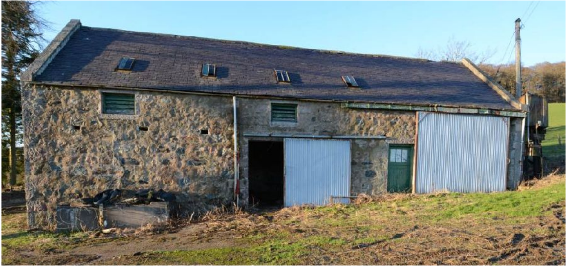
Illus 13 E wall of E range showing cart bay (D3) in centre, windows into loft above (W1, W2) and 3 stable vents
