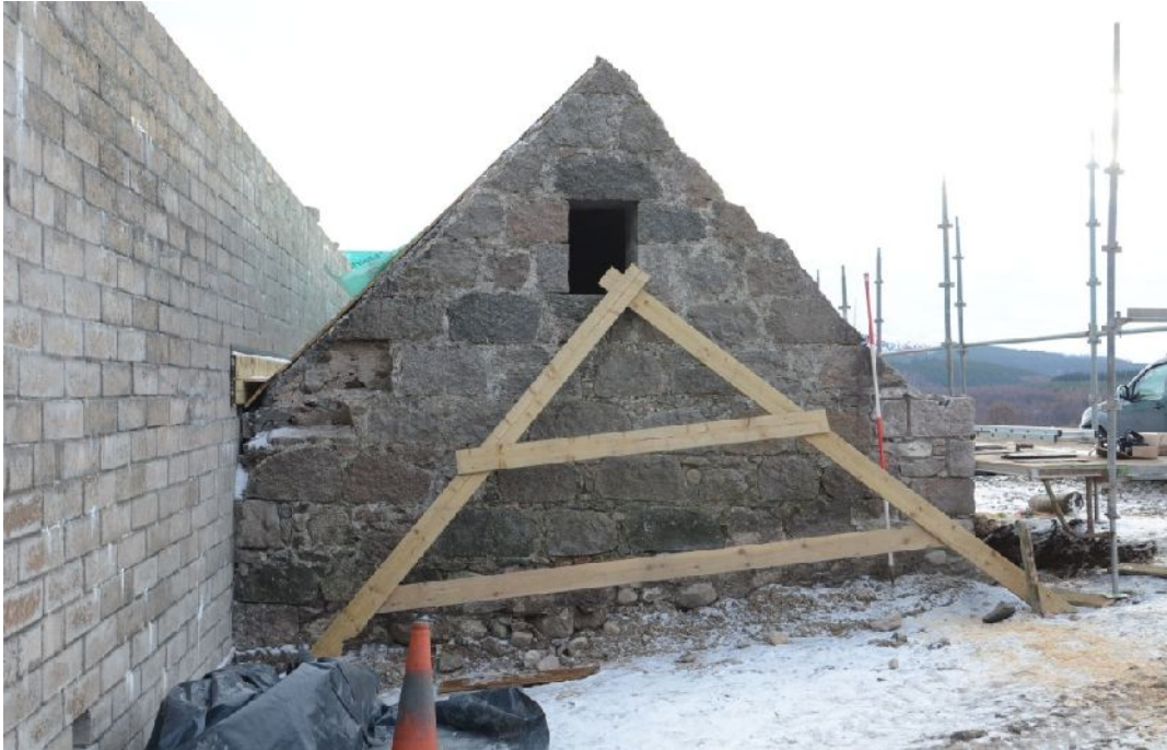
Illus 9 N gable of W range with blockwork infill to E. January 2016
