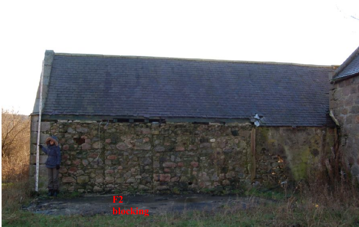
Illus 18 N wall of S range, E of E range.. Note smaller rubble stonework and blocked doorway(?).January 2015 (Photograph courtesy of Acanthus Architects Ltd).
