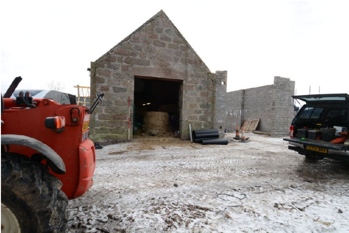
Illus 23 N gable E range January 2016. Note concrete block infill between E and W ranges.
