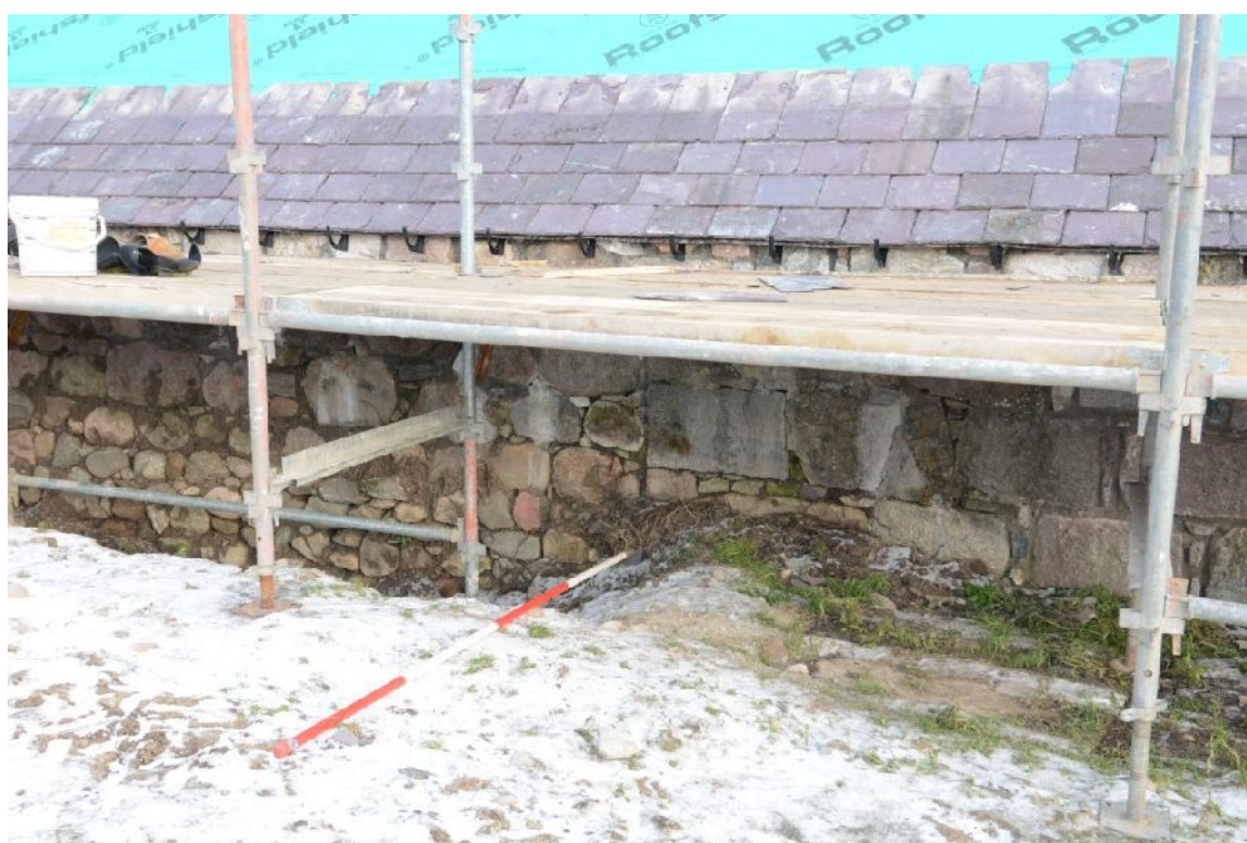
Illus 13 W wall of W range showing difference in stonework at rebuilt section. January 2016
