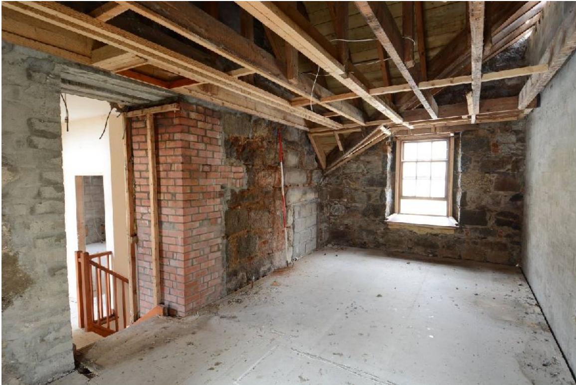
Illus 14 Location of blocked fireplace
