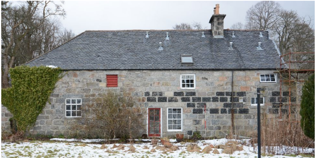
Illus 8 Back (S) wall of Stable (LHS) and No 1 (RHS)
