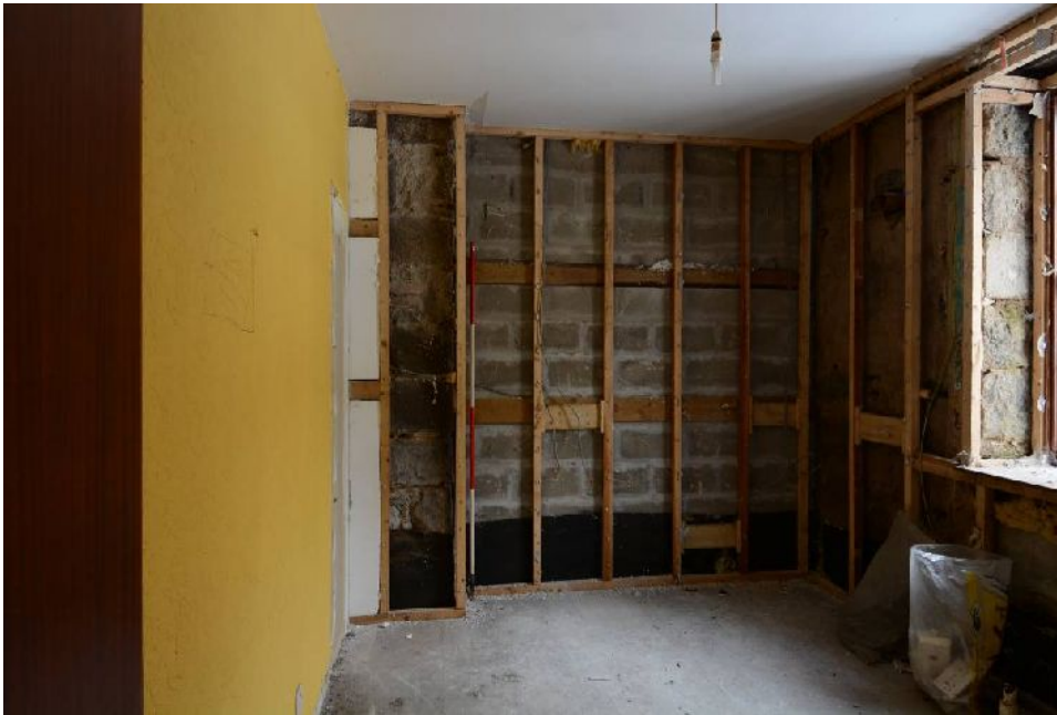
Illus 12 Concrete blocking at ground floor between No 1 kitchen and stable
