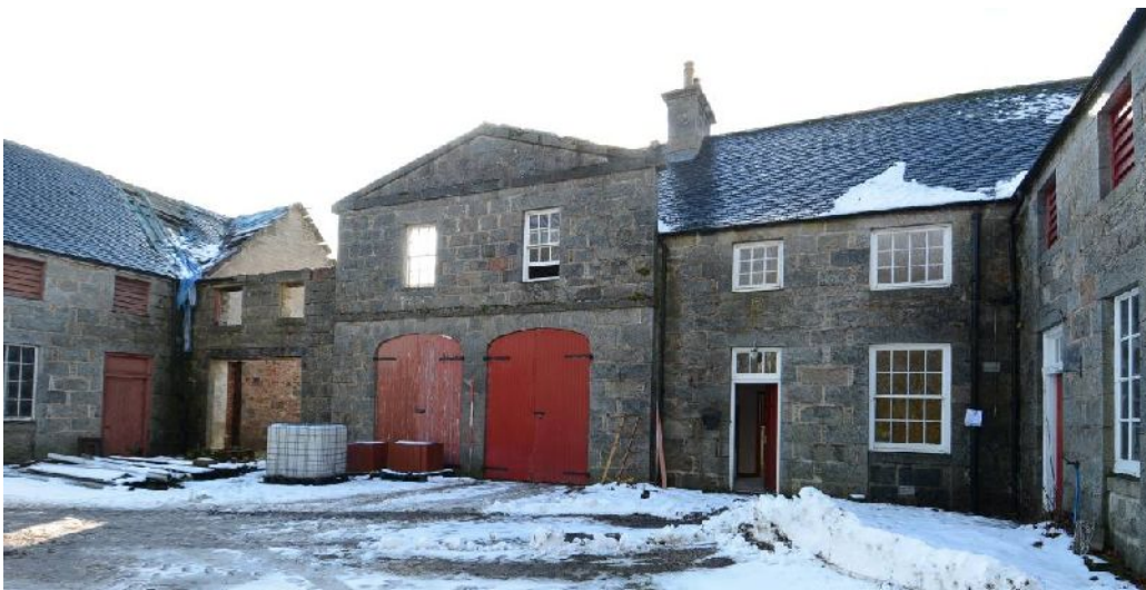
Illus 5 Front of building
