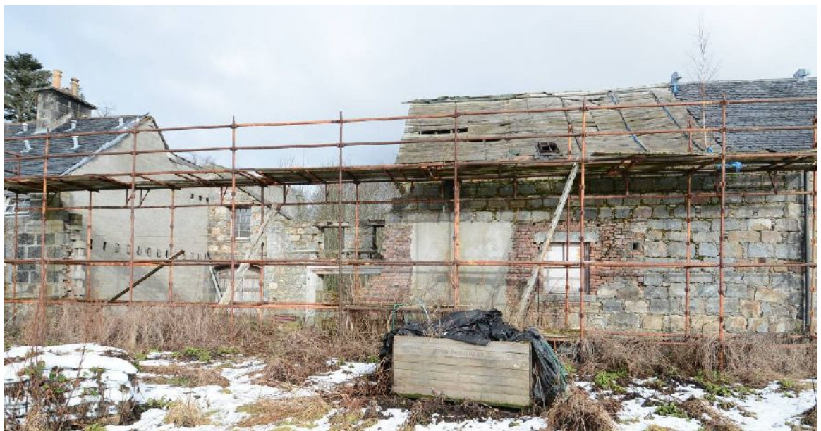
Illus 9 Back (S) wall of range adjoining No 2, showing brick infill
