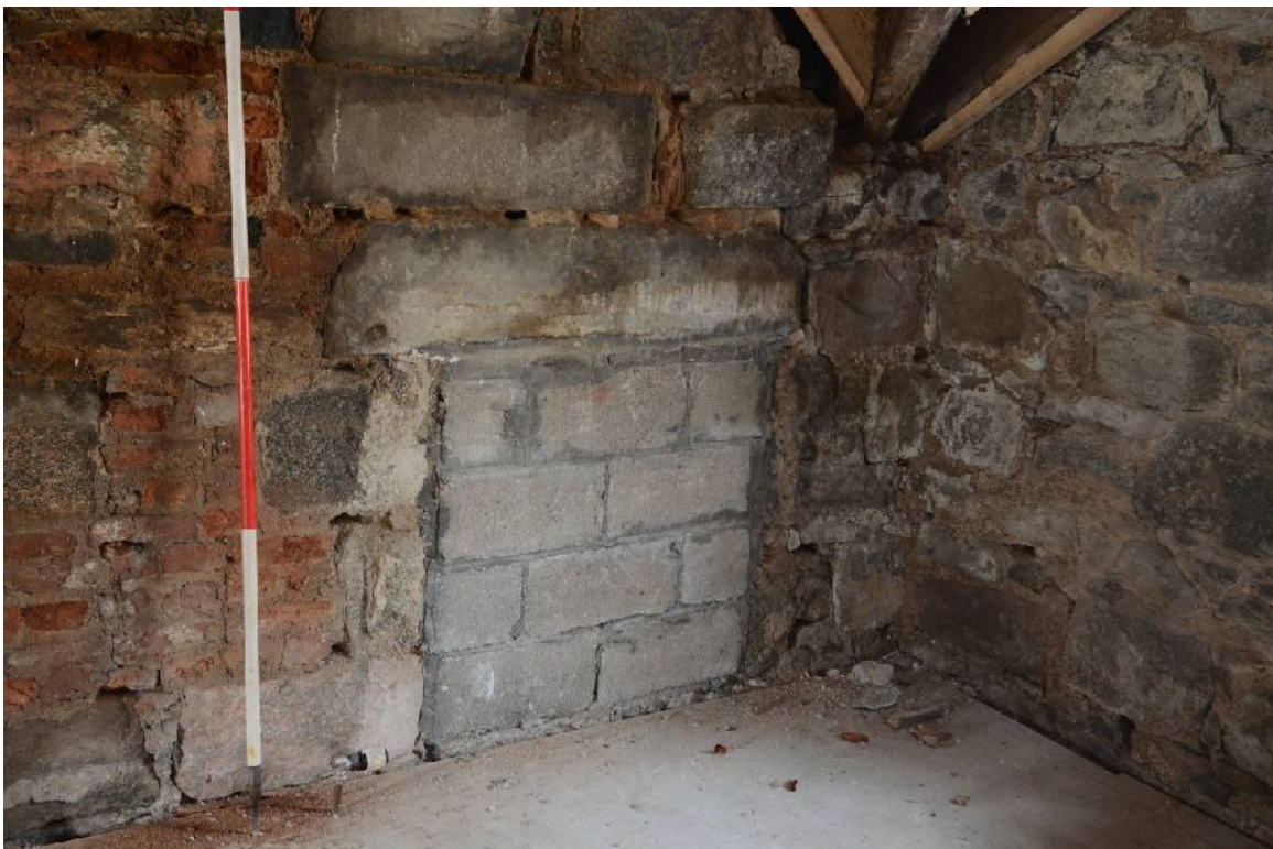
Illus 15 Detail of blocked fireplace
