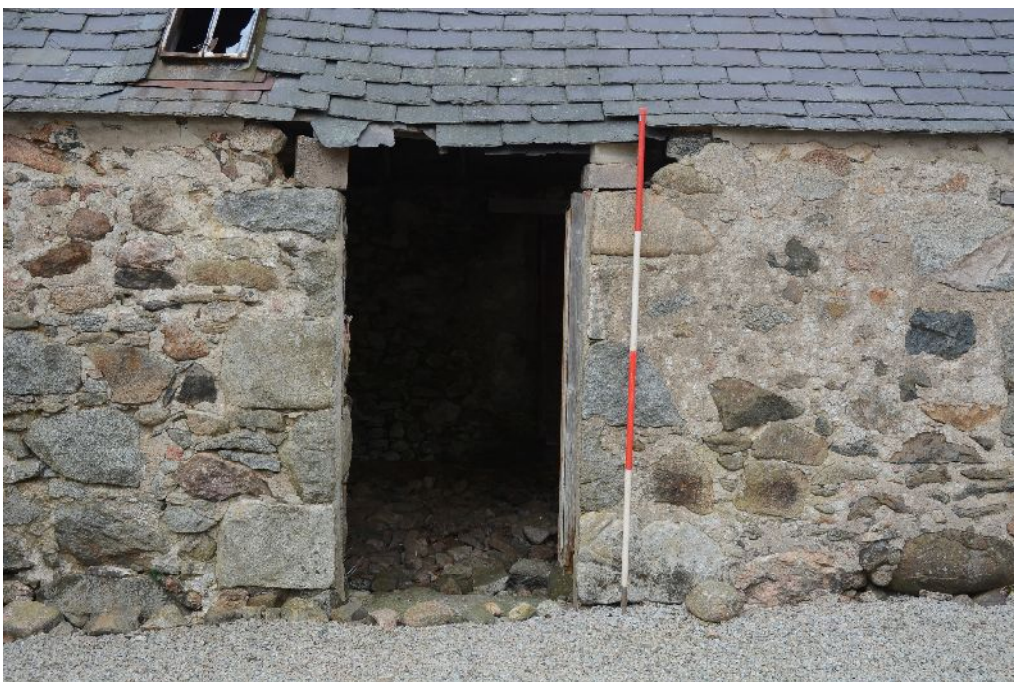
Illus 8 Wall 2. D3. Note buff coloured stonework
