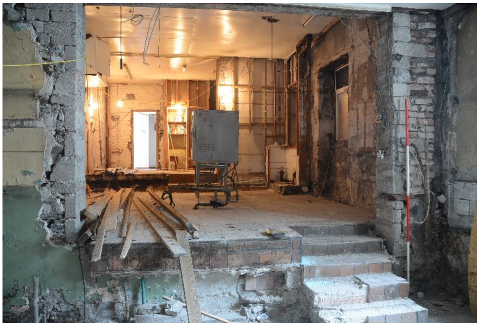
Illus 11 Ground floor looking N from servery to kitchen
