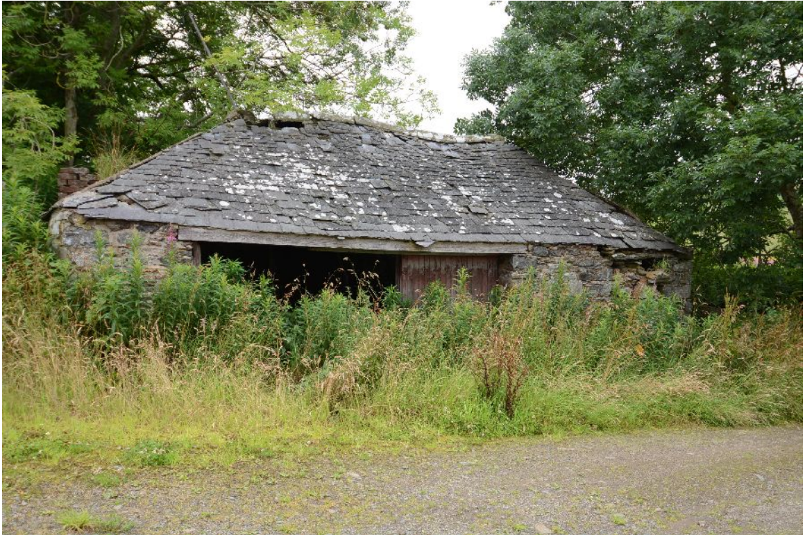
Illus 23 Building 3 S wall
