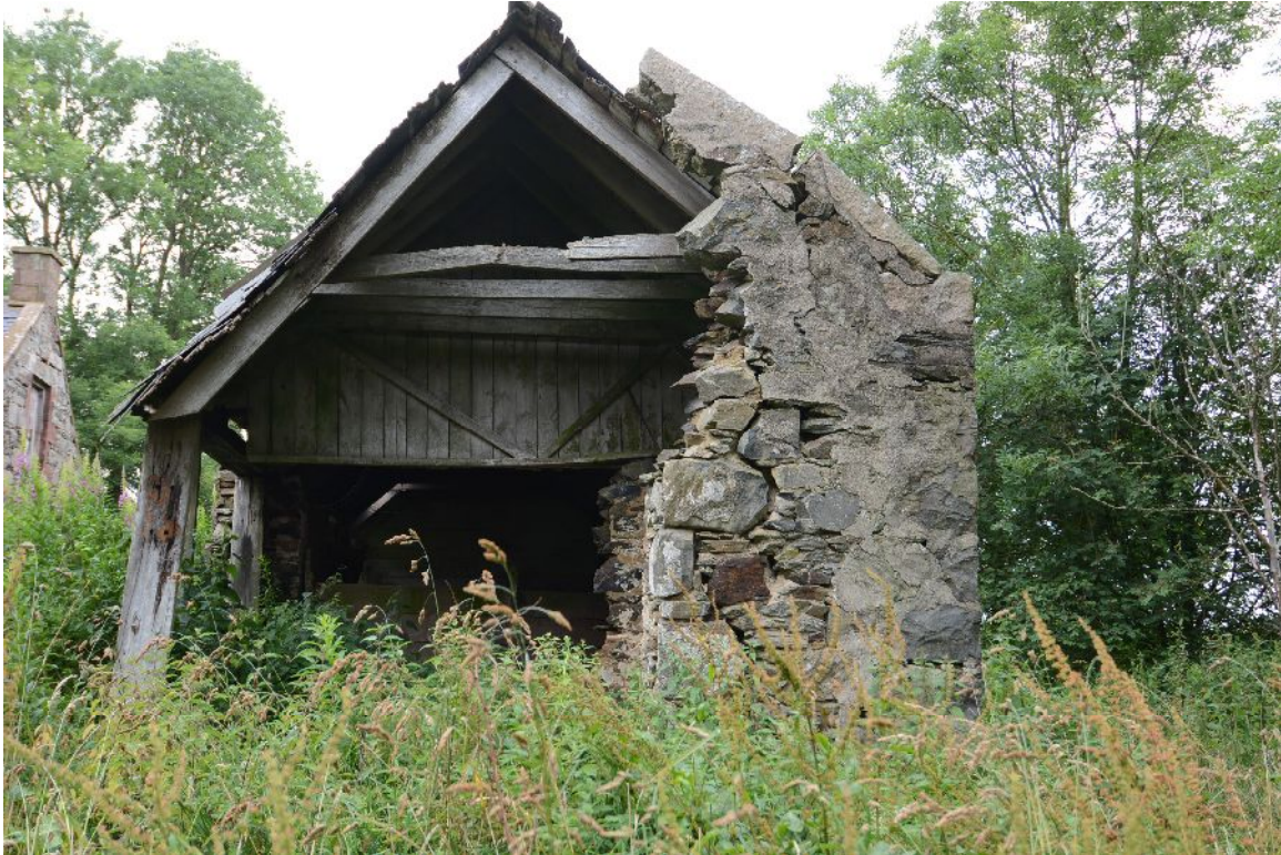
Illus 22 Building 2 S wall
