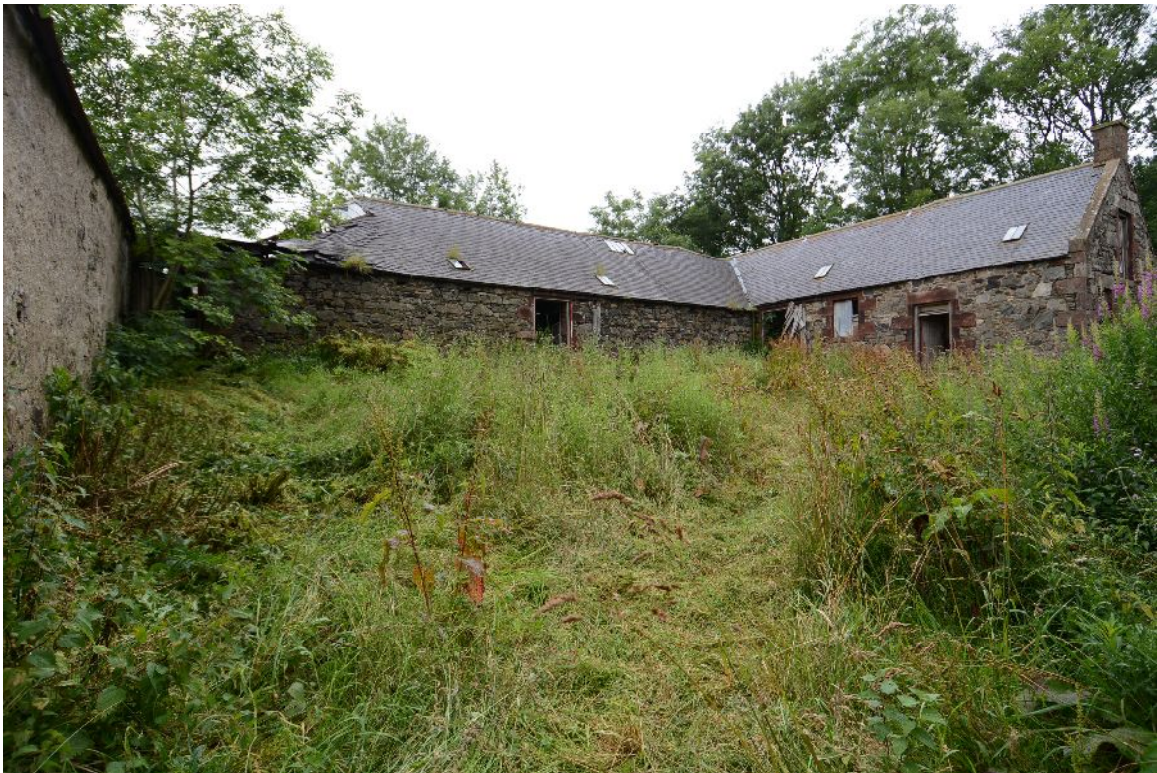
Illus 6 B1, looking WNW into court
