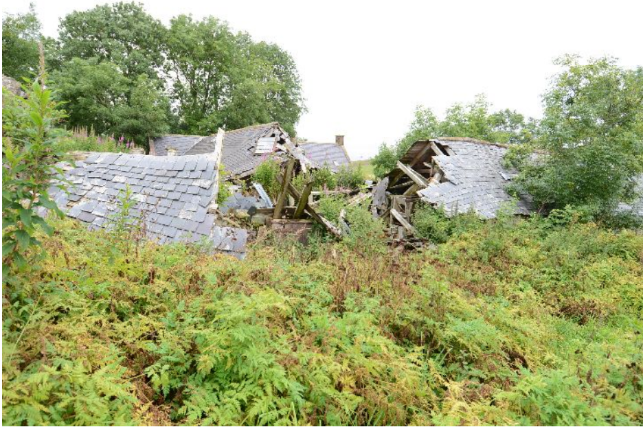
Illus 19 SW corner of Building 1
