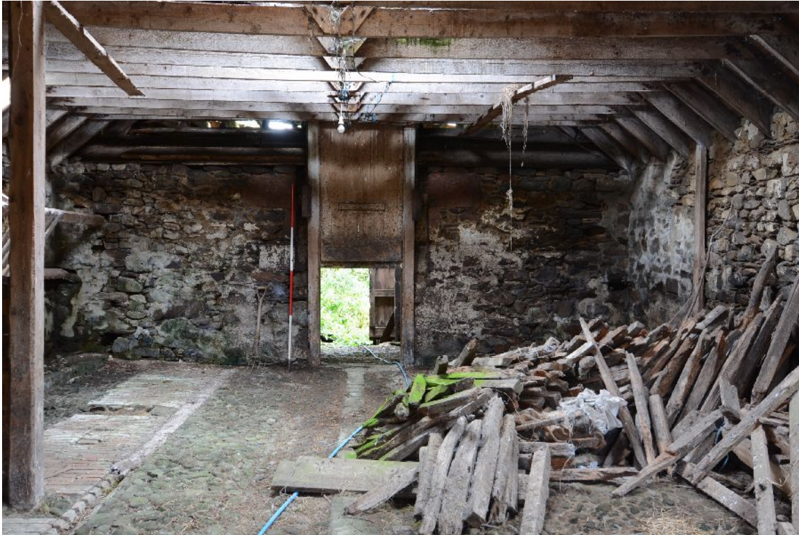
Illus 17 Sliding door at N end W Range, note counter weights at level of top of ranging rod
