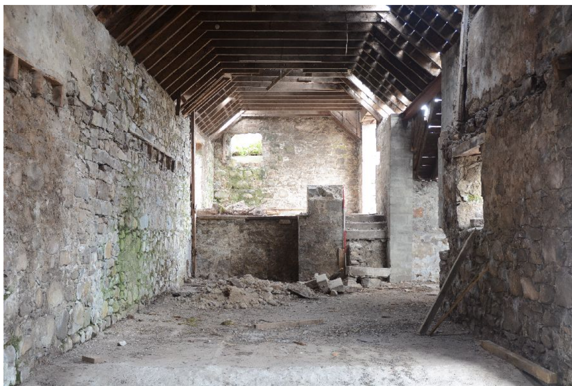
Illus 20 Building 1. W Range looking N towards B1c
