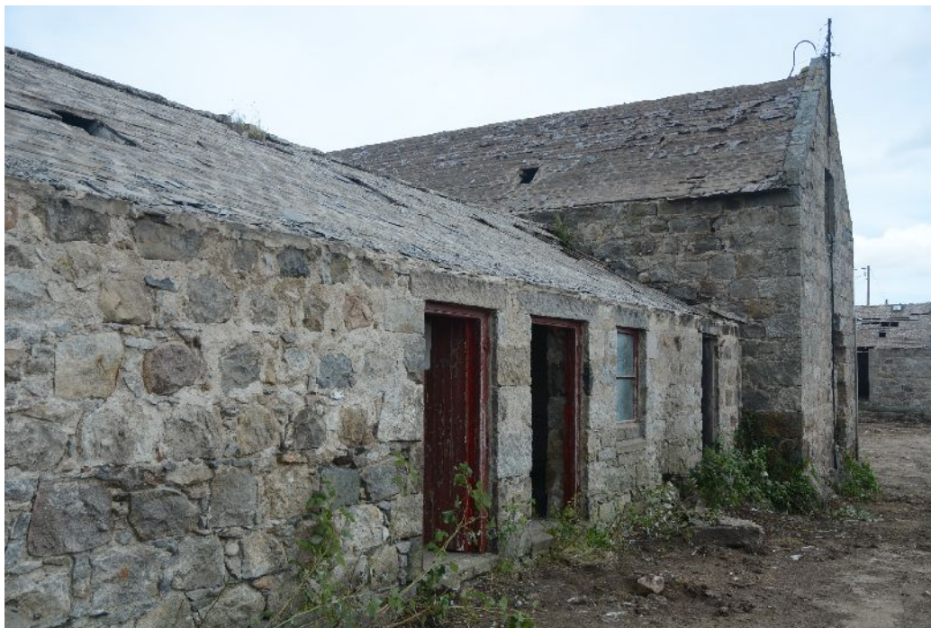
Illus 22 Building B1a abutting W wall of W Range of Building 1
