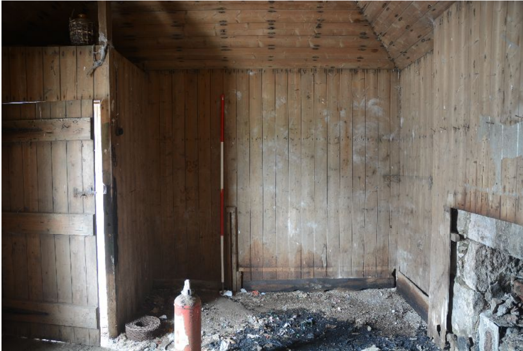
Illus 27 Bothy Interior, looking N. Ranging rod stand beside grooved timber- possibly for box bed. Door to lobby on LHS
