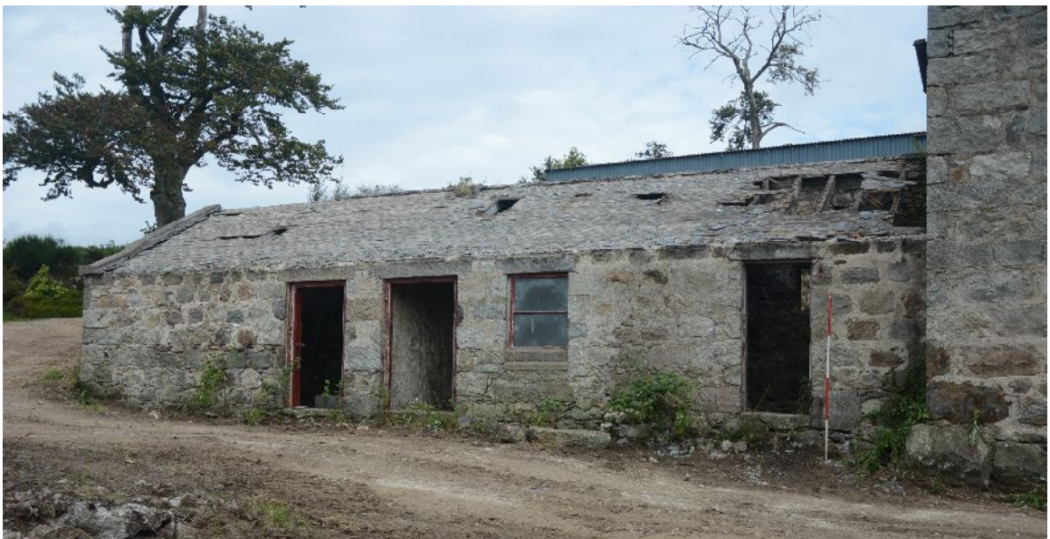
Illus 21 Building B1a looking N. S elevation
