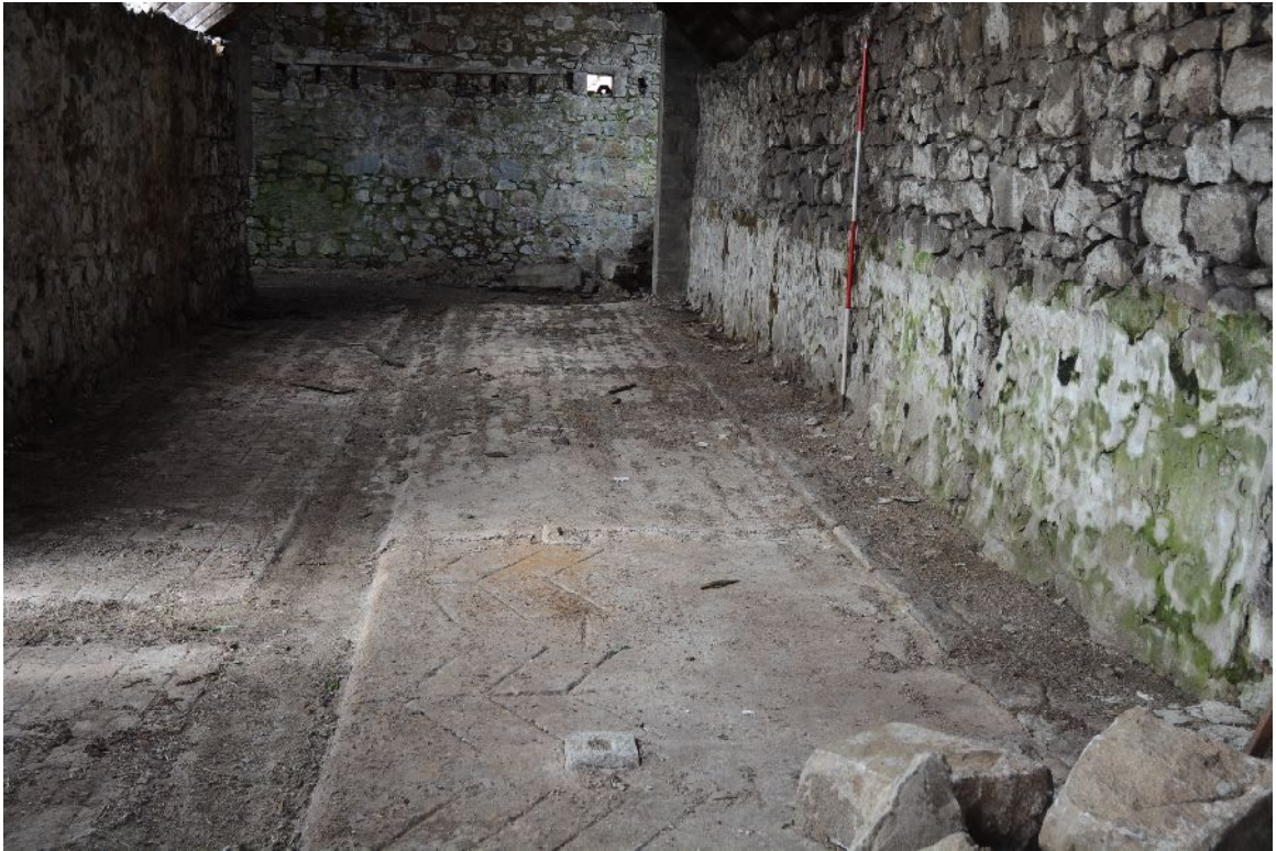
Illus 18 Building 1. Interior of N range. Scars of trevises of double cow pens on wall (RHS). Drains in floor behind cattle (LHS) and trevis post end stubs (centre foreground).
