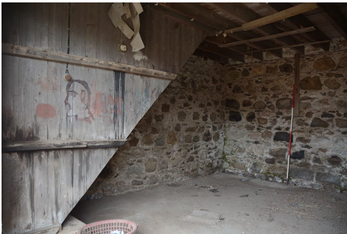
Illus 33 Building 3. N cart bay with underneath of stair on LHS
