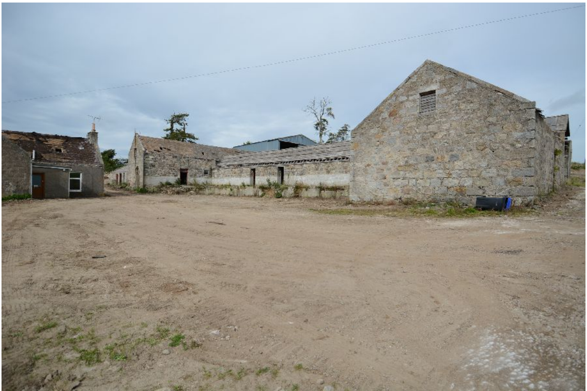
Illus 10 Building 1, general view looking NW (Farmhouse on LHS)
