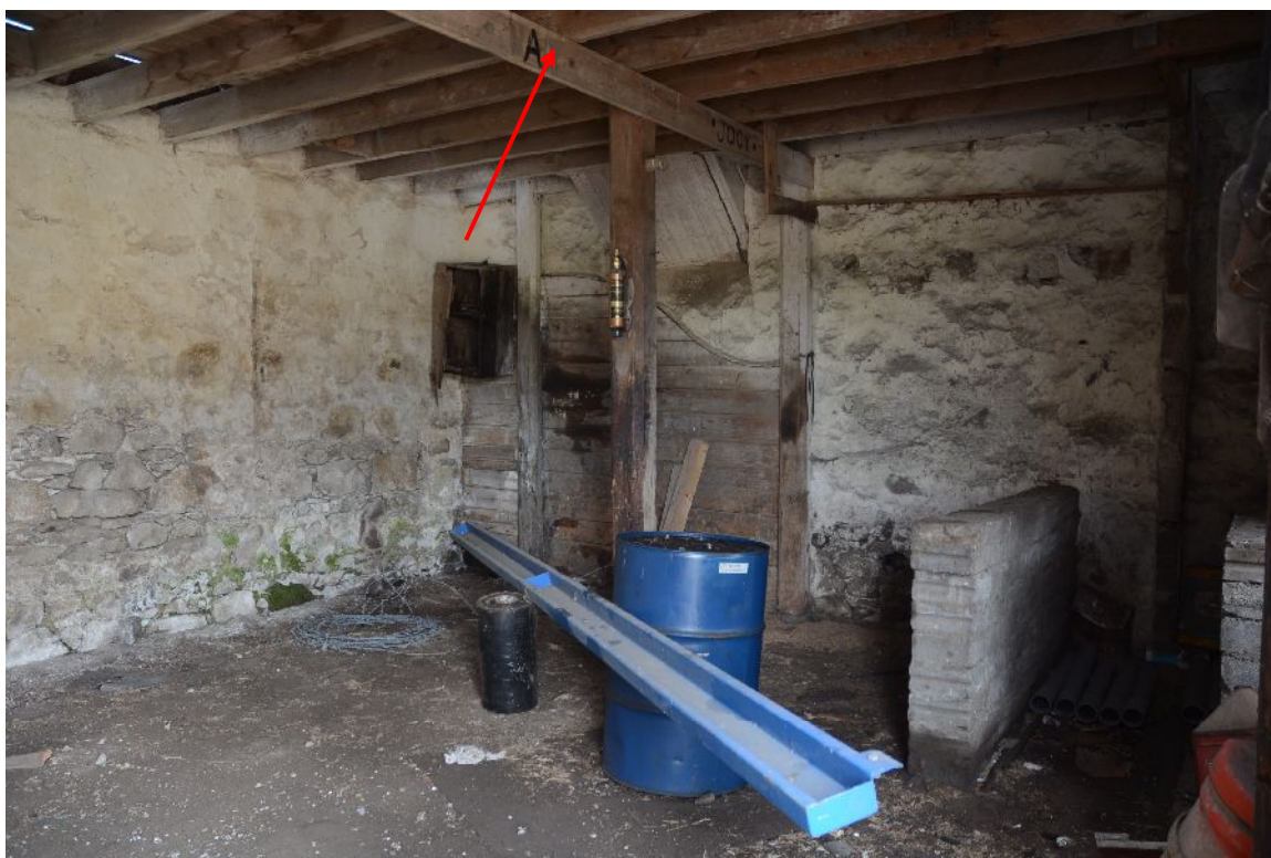
Illus 37 Building 3. Stable looking S. Names on beam above (red arrow)
