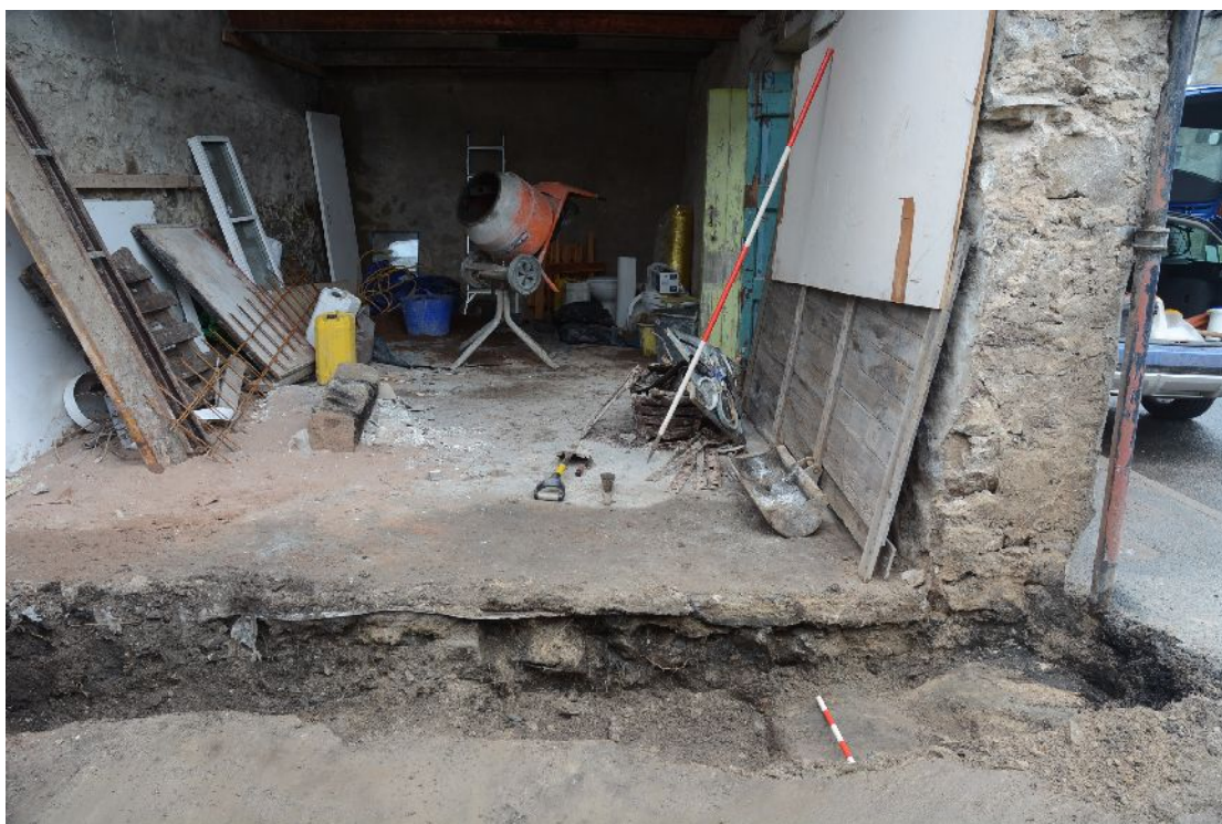
Illus 5 Looking S into No 8 George Street across the trench where gable removed. Note small measuring rod is on the line of the front wall stone foundation.
