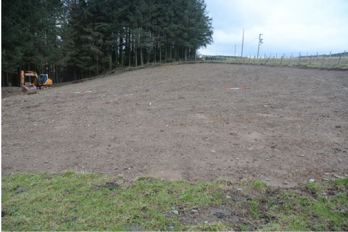
Illus 1 General view of site with topsoil stripped, looking SW
