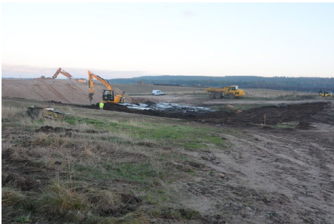
Illus 9 General view of soil stripping looking S
