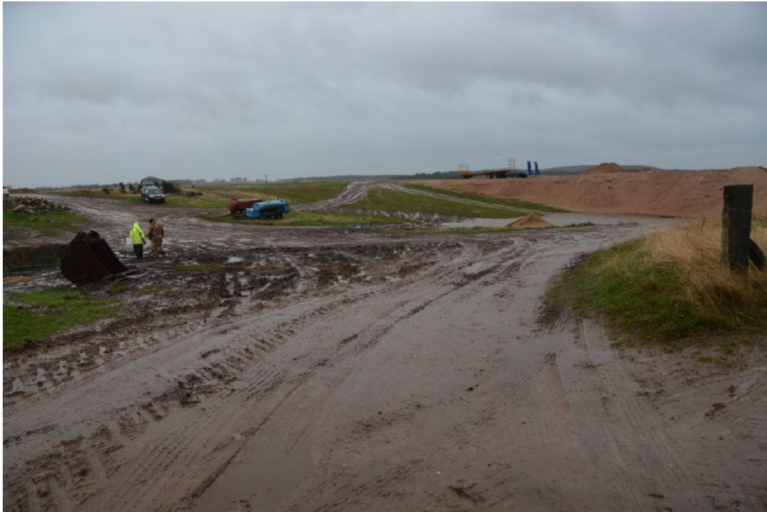
Illus 2 General view of site 7 th January 2016
