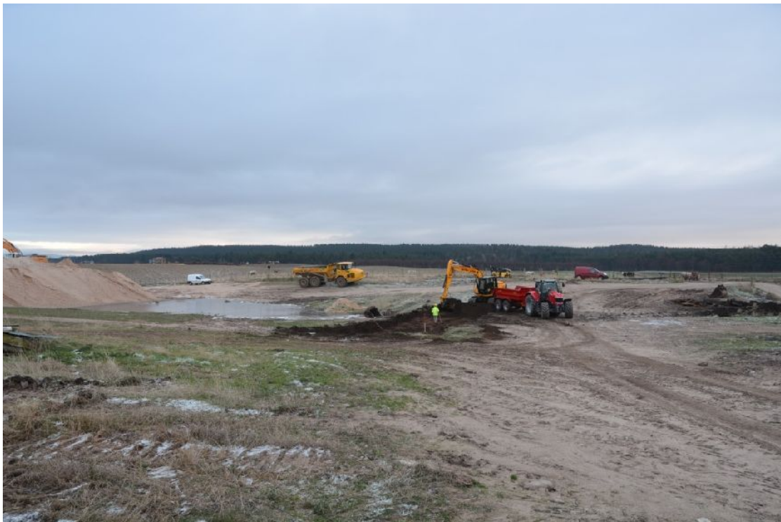
Illus 1 General view during soil strip looking S
