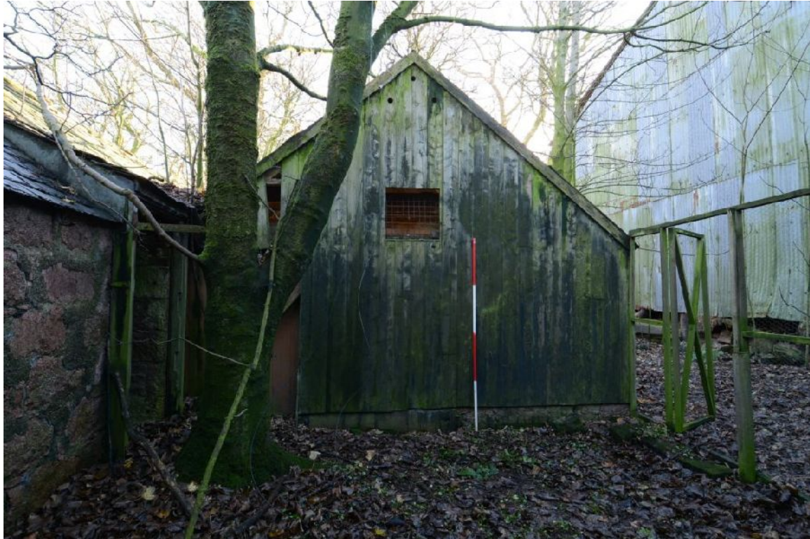
Illus 20 Building 3 abutting Building 2, looking SE
