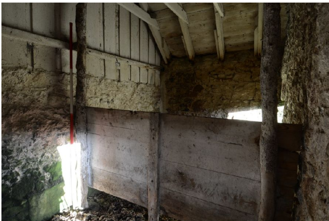
Illus 16 Timber partition between the two pig stalls in Building 2, area D
