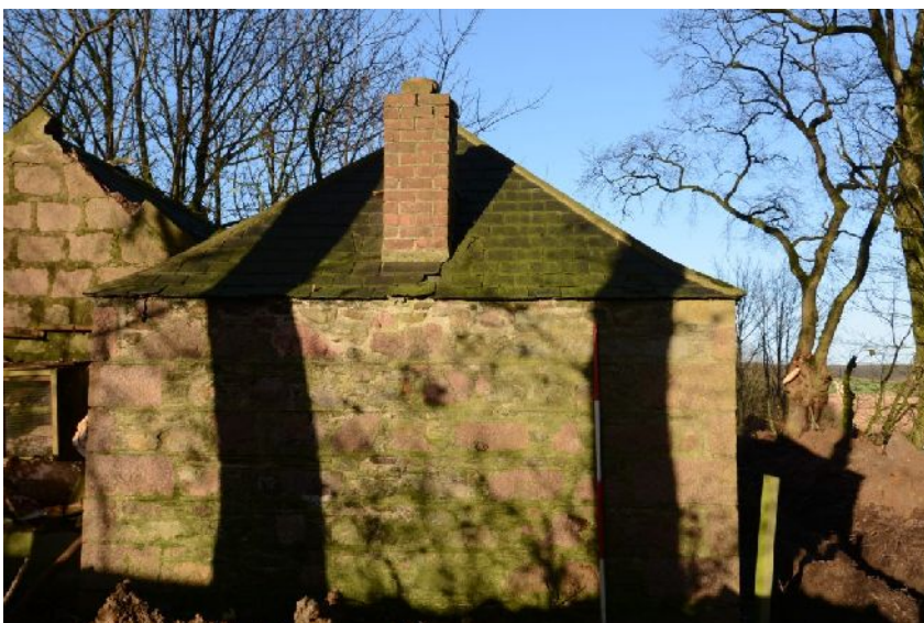
Illus 6 Building 1 Chimney at SE end
