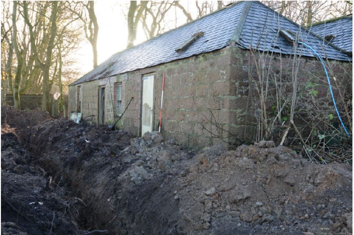
Illus 5 NE (front) facade of Building 1, looking S.
