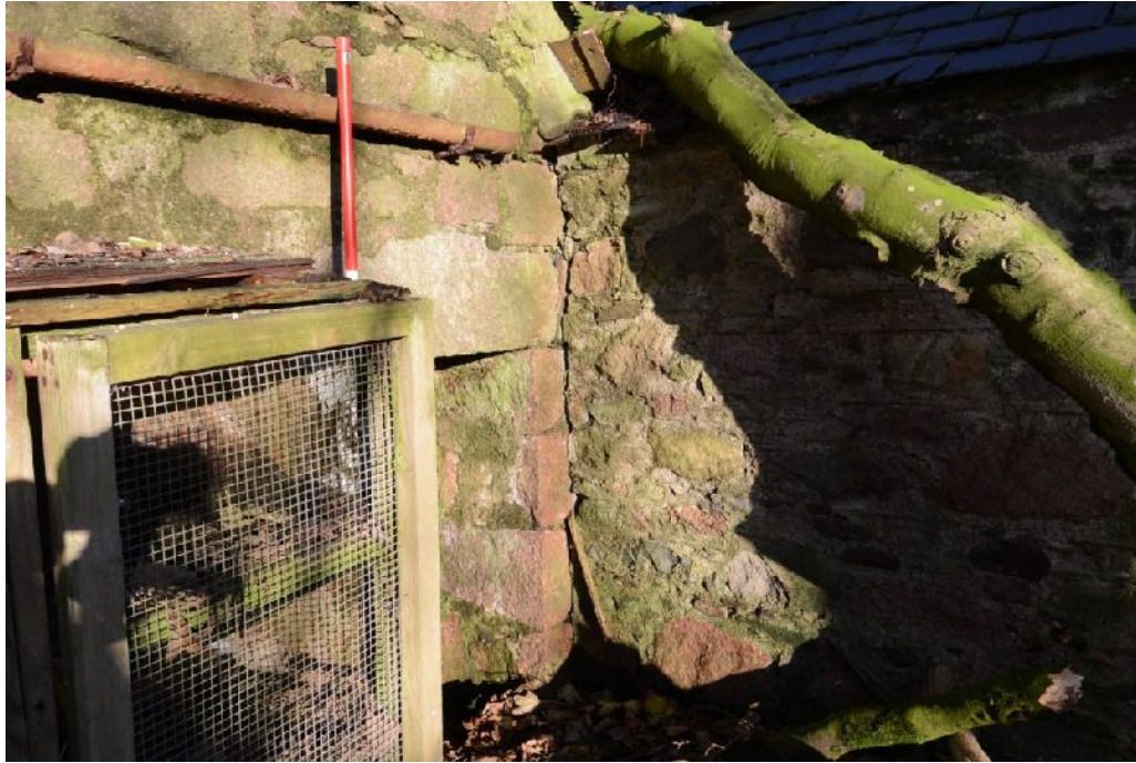
Illus 21 S end of back wall of Building 1 abutting SE corner of Building 2
