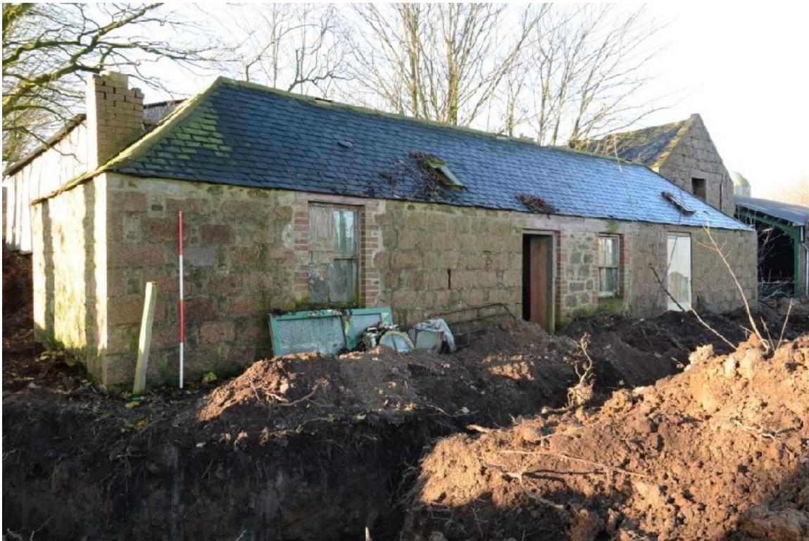
Illus 22 Building 1 NE frontage showing secondary insertions
