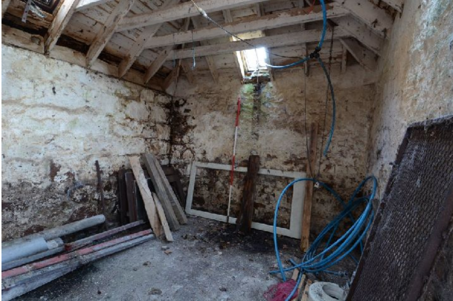
Illus 7 Interior of Building 1, 'Room' A, looking W
